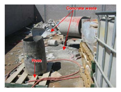
**Photograph 17: Mesa Municipal Court** Concrete waste and washout hose located near mixer
