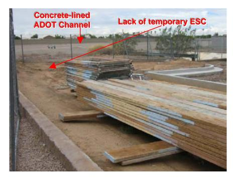
**Photograph 11: Superstition Springs Commerce Center** View showing proximity of site to the ADOT Channel and lack of BMPs
