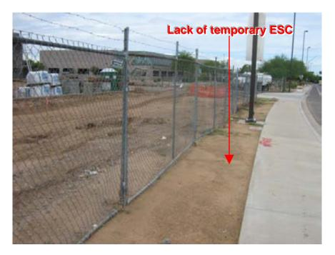
Photograph 12: Superstition Springs Commerce Center BMPs were not implemented as perimeter control along Hampton Avenue, between the disturbed area and the offsite curb and gutter flowline
