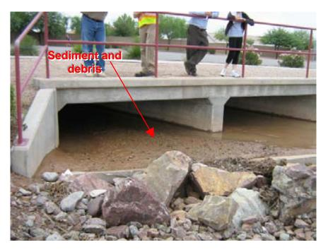
Photograph 7: Mountain View Village Center Sediment and debris were observed in the drainage channel above the flow control structure
