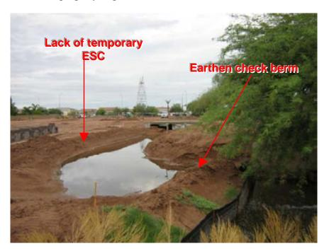
Photograph 2: Mountain View Village Center View of drainage channel leading west across the site and earthen check berms installed along this course
