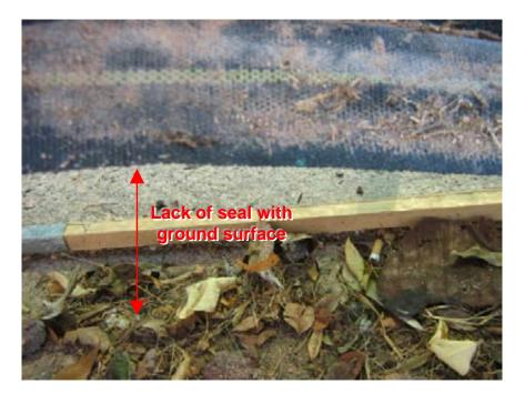
Photograph 16: Mesa Municipal Court Sections of the silt fence along the southern perimeter were not maintained with adequate entrenchment
