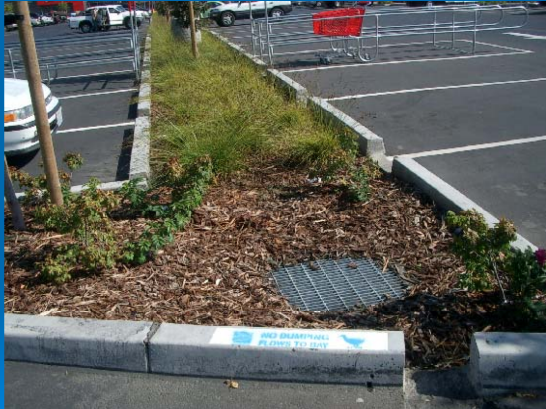
Parking lot treatment- vegetative buffer strip
