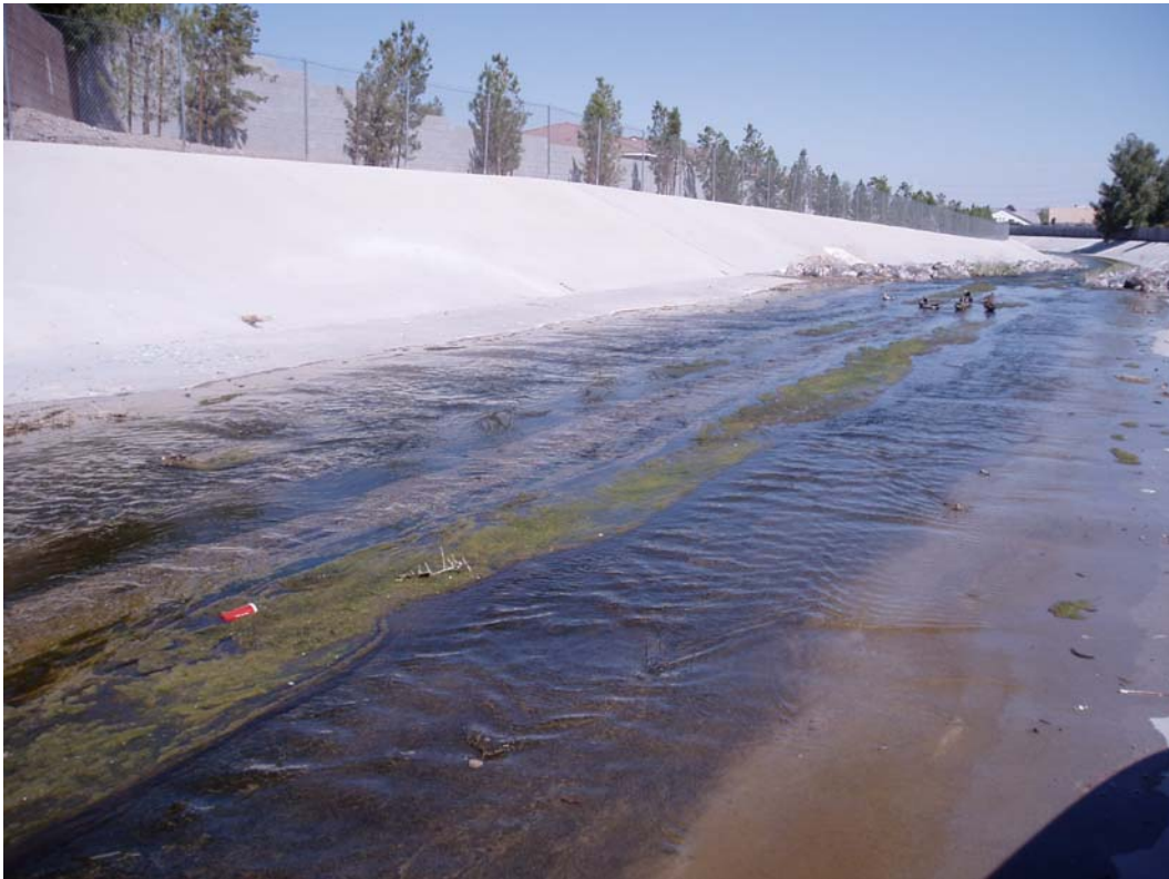
Photo 19. Bottom of channel.
