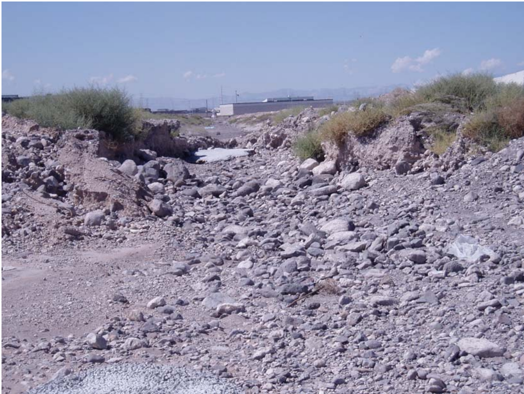
Photo 23. Culvert to Gibson Channel.
