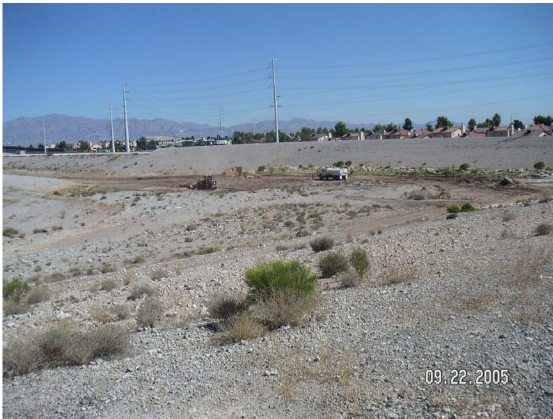
Photo 5. Angel Park South Detention Basin.
