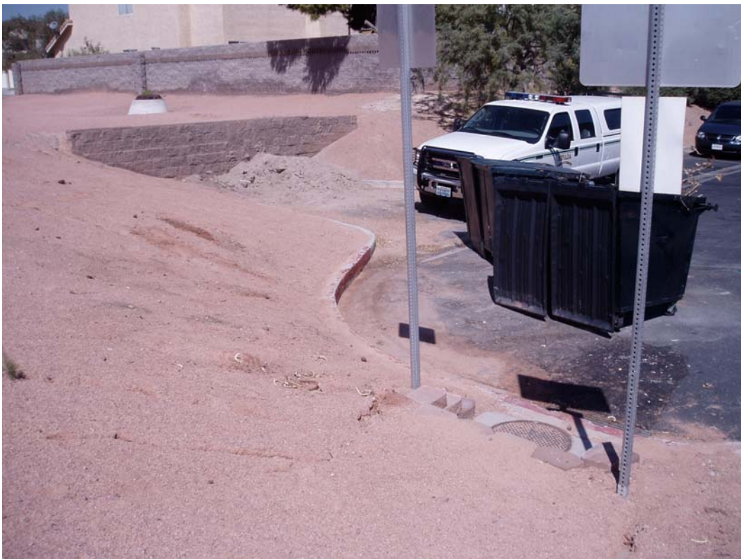
Photo 8. Parks and Recreation Department dirt storage. Trackout visible to inlet, which flows to outfall in Photo 7.
