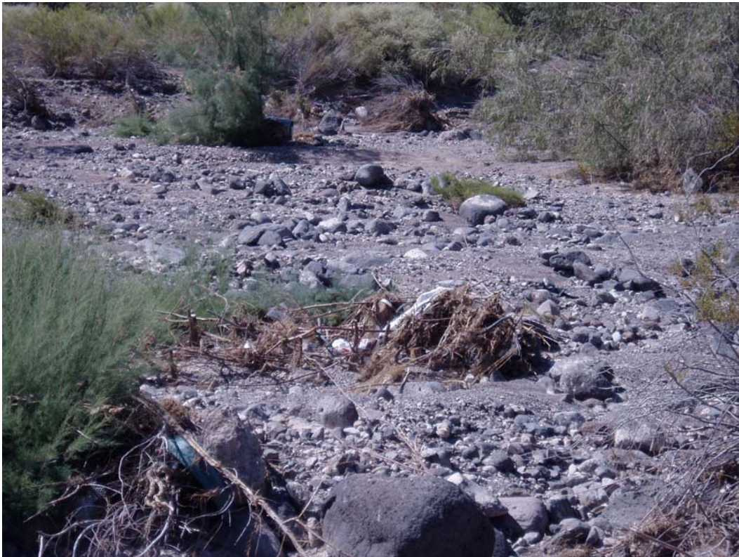
Photo 5. Tamarisk and debris in Project Green area of Pittman Wash.
