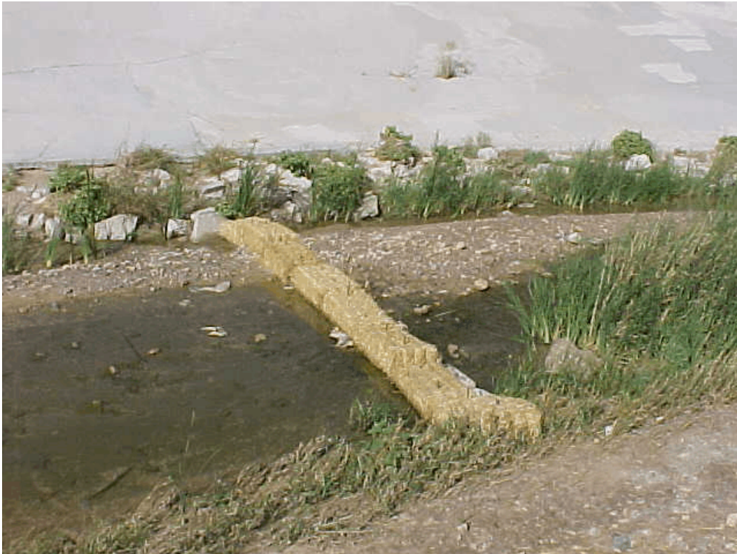
Photo 5. View of straw bale filter in Duck Creek Channel downstream from the construction area.
