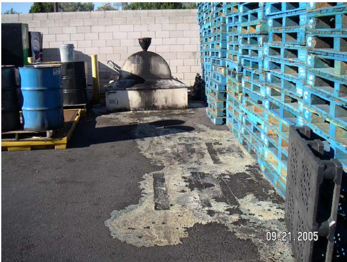
Photo 10. Dried milk solids on asphalt inside facility.
