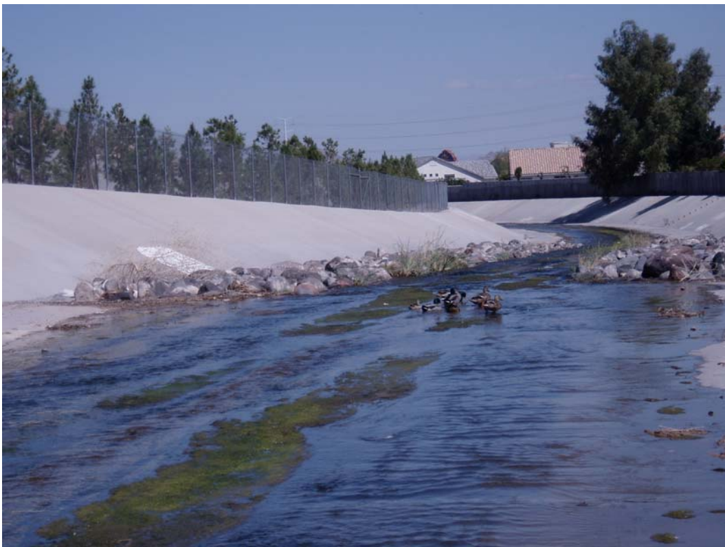
Photo 20. Bottom of channel.
