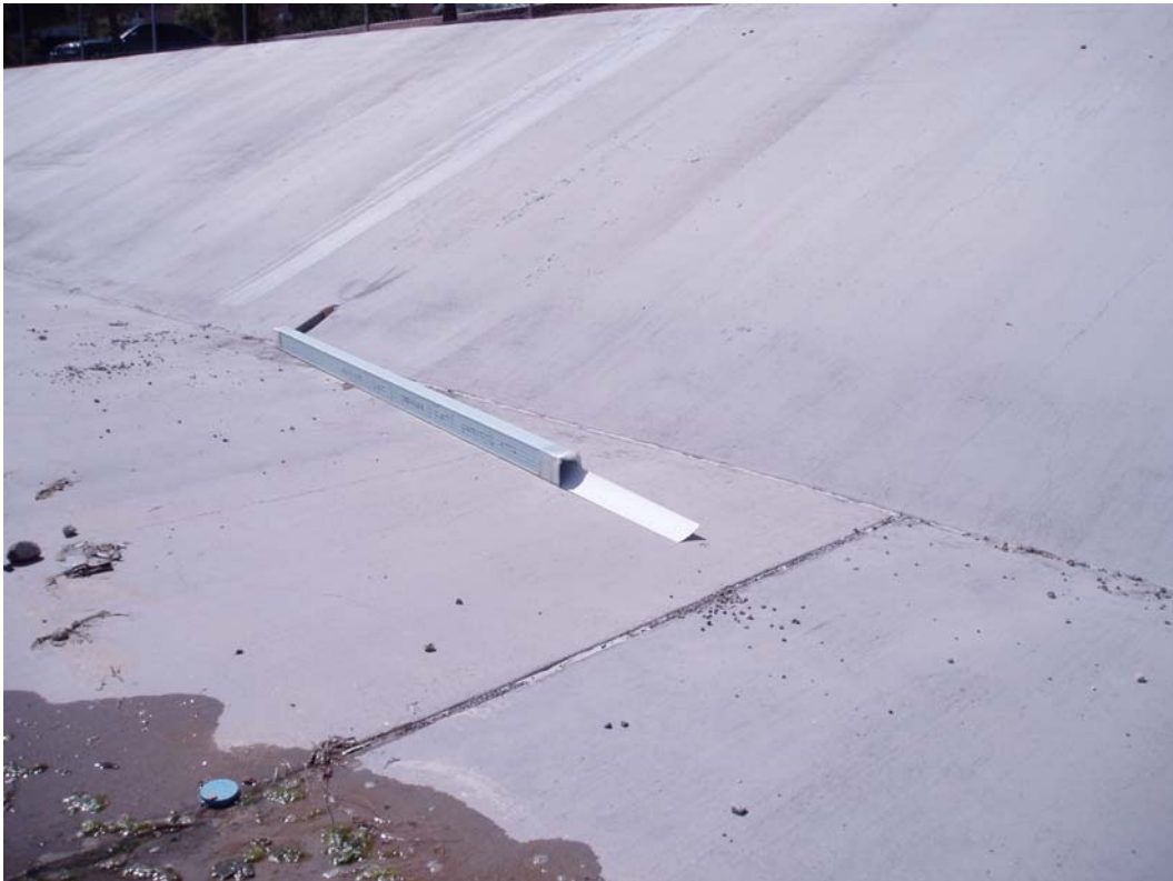
Photo 21. Empty box dumped in channel.
