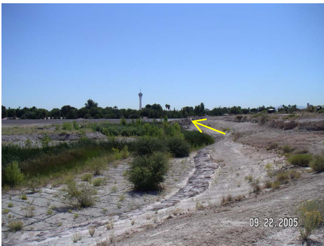
Photo 8. Meadows Detention Basin - inlet area.
