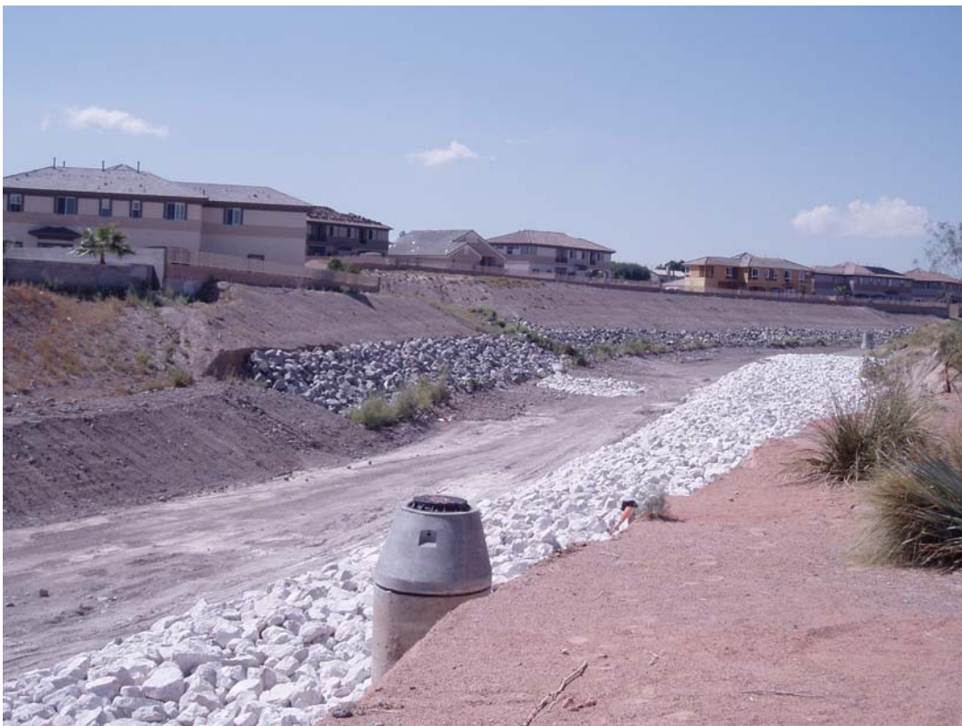
Photo 10. Riprap along Upper Pittman Wash.
