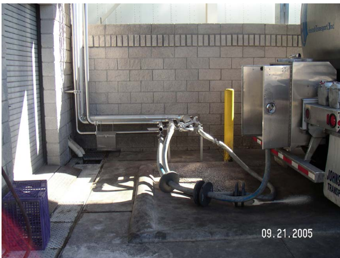
Photo 6. Tank truck off loading area.
