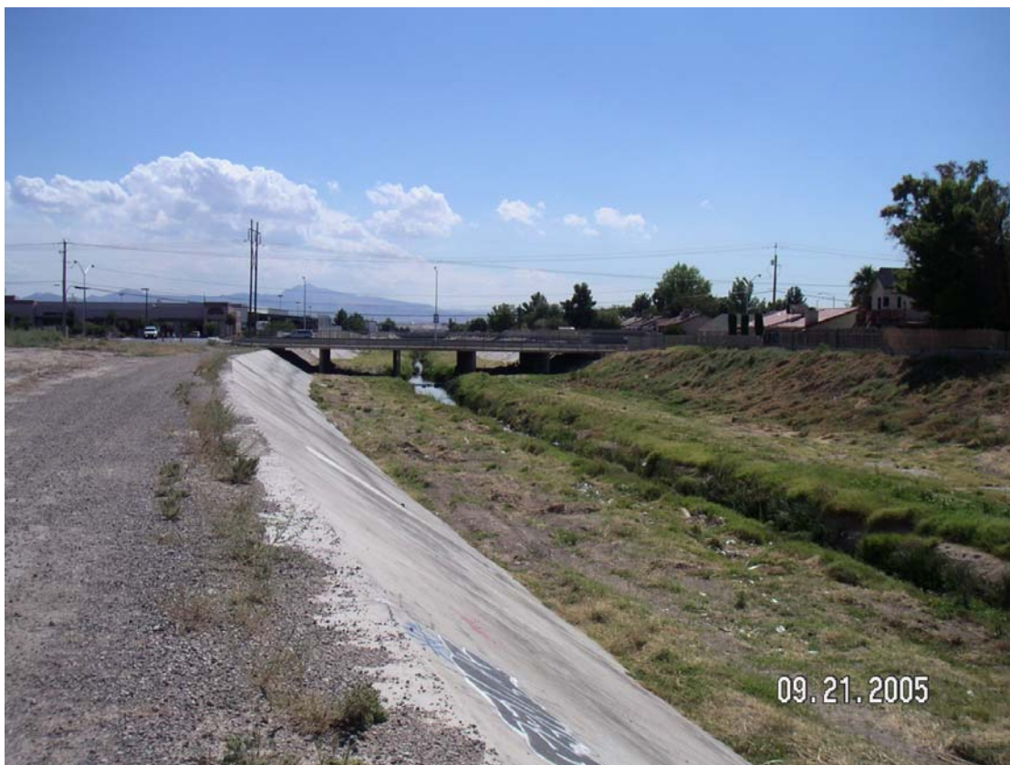
Photo 3. View of Las Vegas Wash near intersection of Stewart Avenue and Nellis Boulevard.
