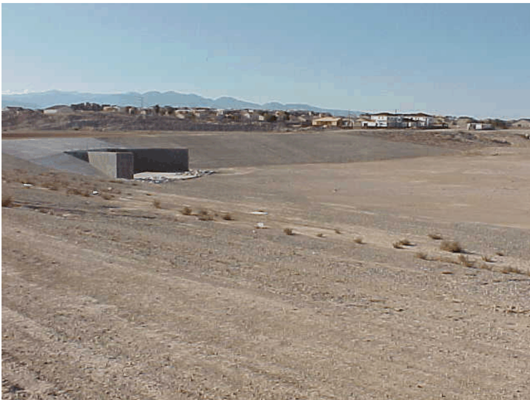
Photo 6. Inlet to detention basin at southwest corner.
