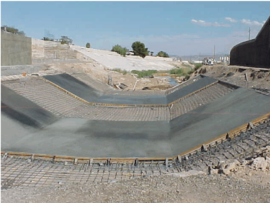
Photo 4. View downstream from earthen dam of Duck Creek Channel (photo center) and retaining walls (photo left and right).
