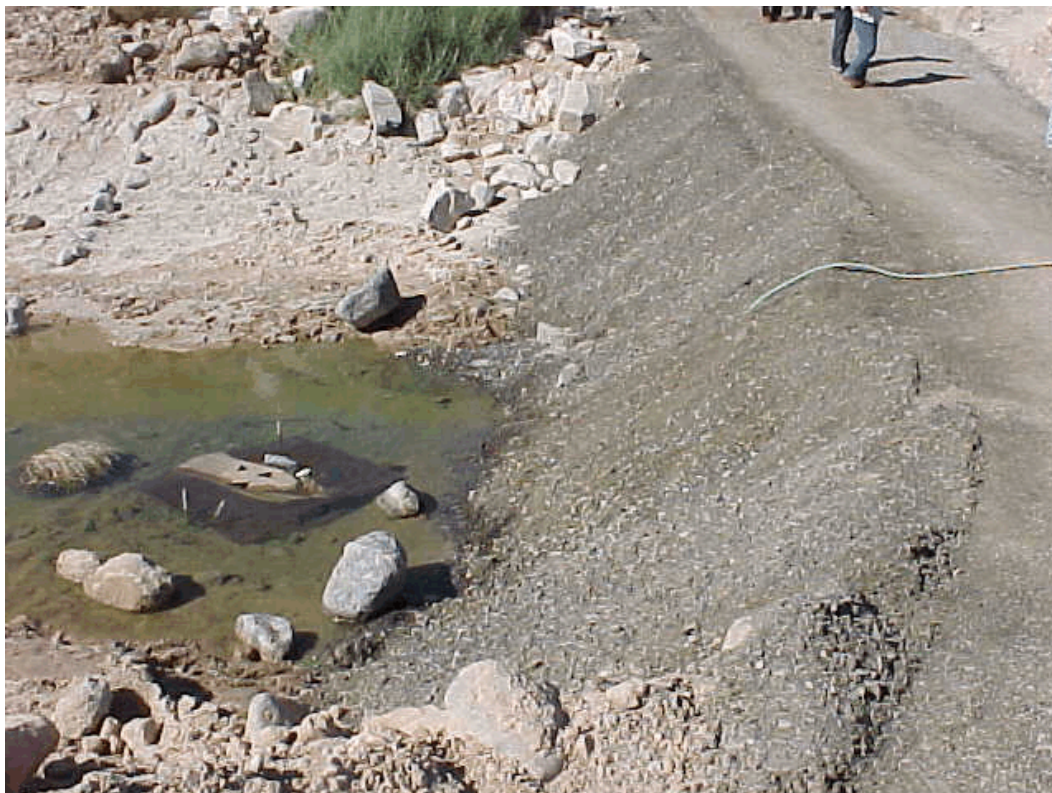
Photo 1. Diversion inlet (photo left) and earthen dam.
