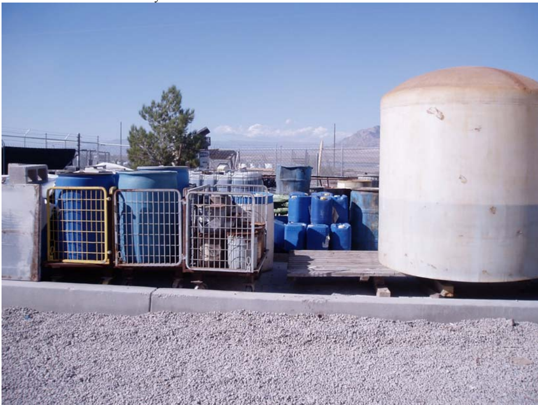
Photo 2. Bermed area for chemical storage.
