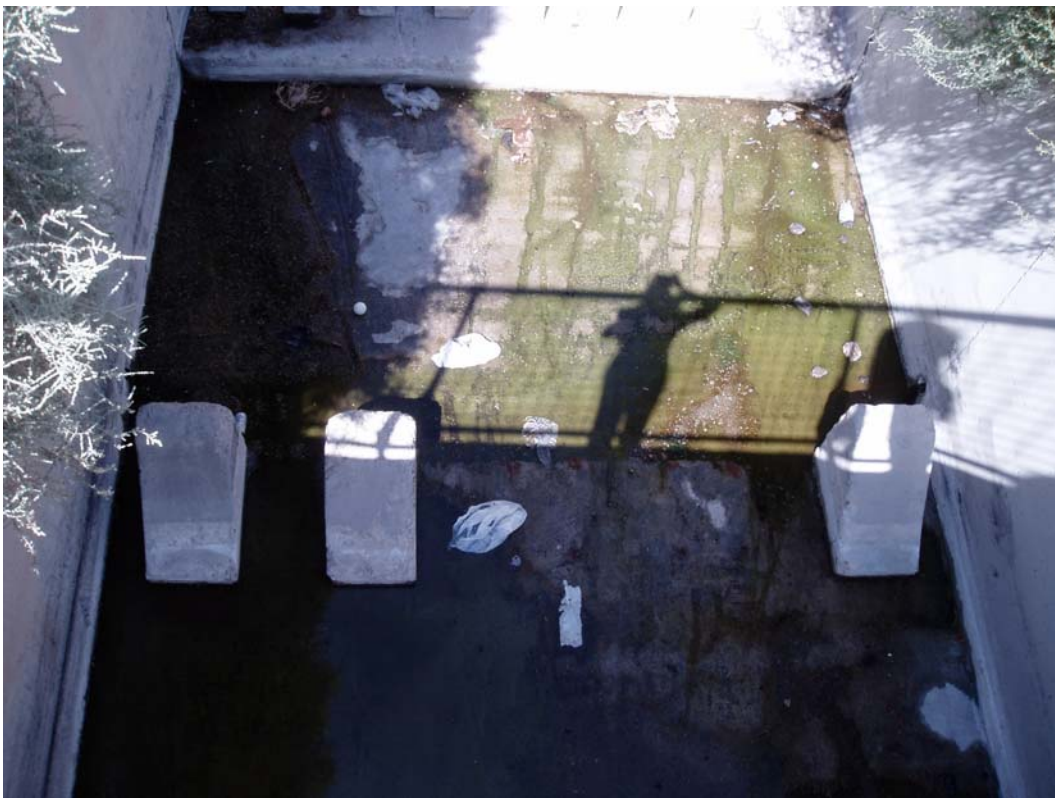
Photo 12. Bottom of Union Pacific Railroad Channel.
