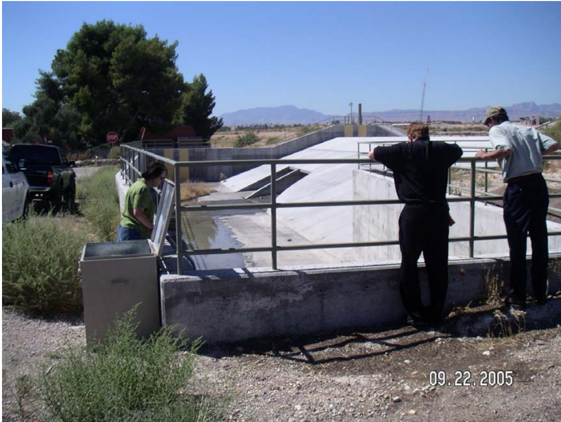
Photo 13. Meadows Detention Basin - effluent sampler and outfall.
