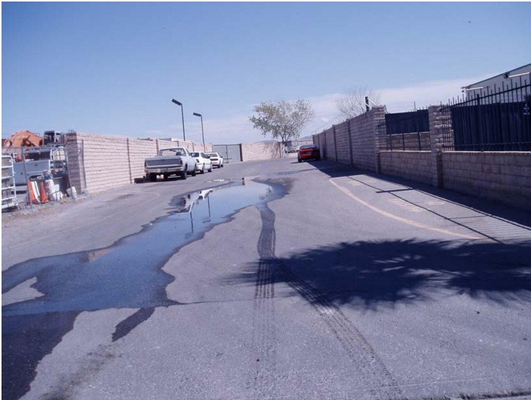
Photo 29. Discharge coming from B.Witt parking lot.
