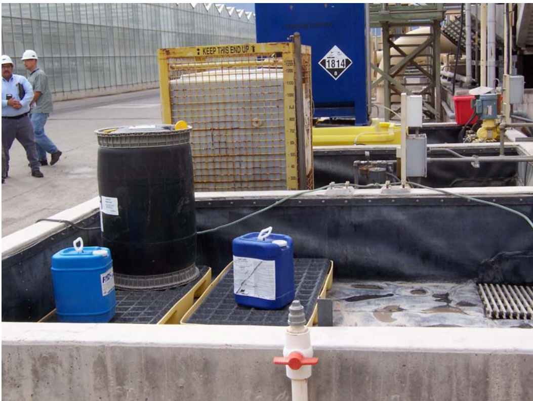
Photo 2. The inspector did note that all containers five gallons or larger have been provided with secondary containment as required by local ordinance.
