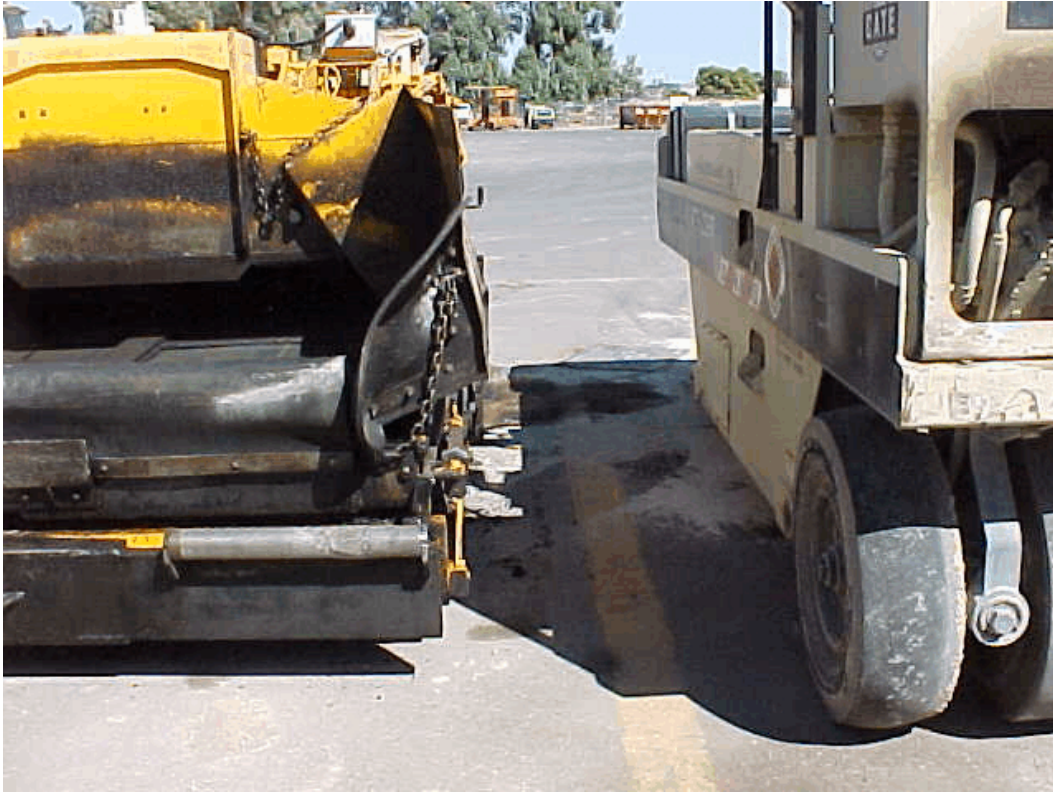
Photo 11. Fleet (secondary) facility: Truck and paving equipment parking area with spills/leakage staining on pavement.
