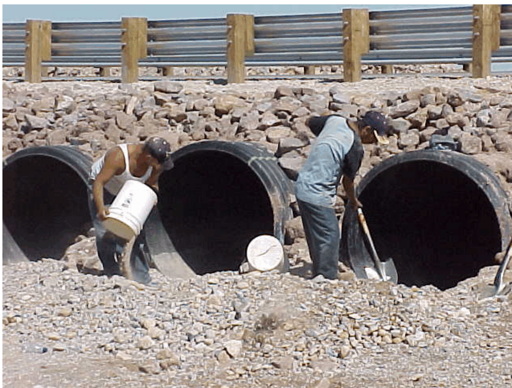
Photo 4. KB Home hand cleaning of culverts in wash.
