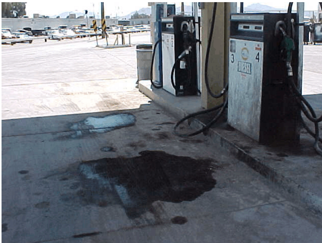
Photo 7. Spillage at fuel island.
