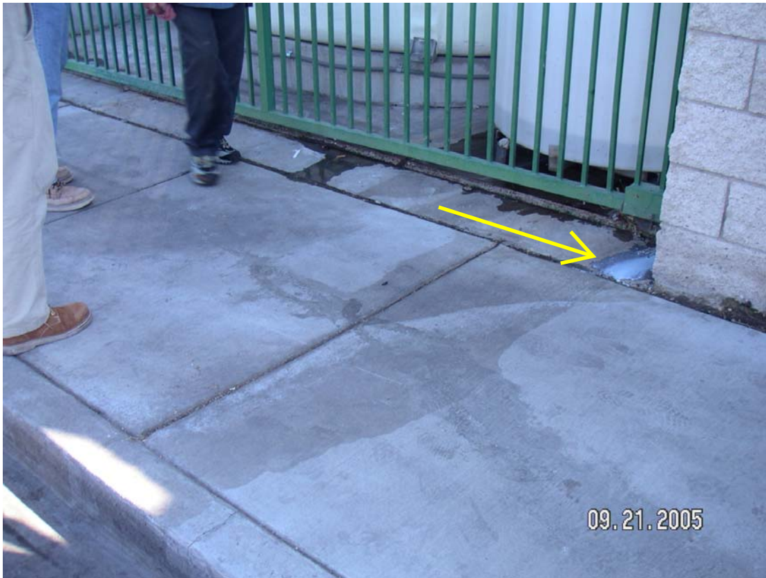
Photo 9. Discharge to street from leaking tank.
