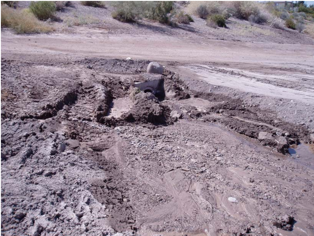
Photo 17. Outfall that discharges groundwater.
