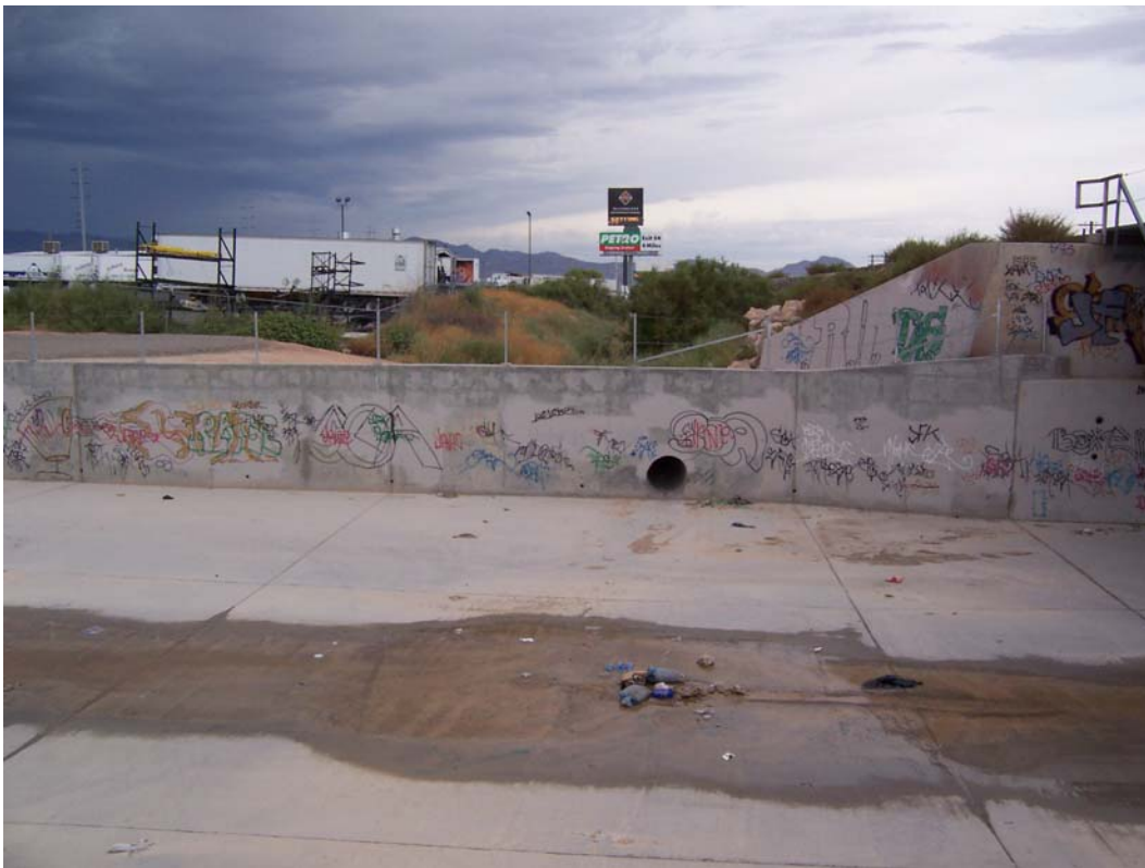
Photo 1. View across Channel A wash.
