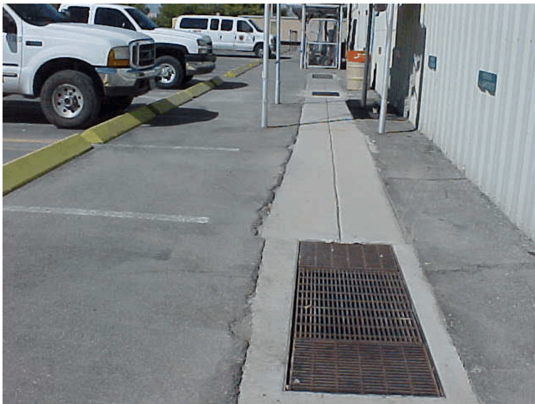
Photo 1. Fleet (primary) facility: Unprotected storm water inlets at north edge of parking area.
