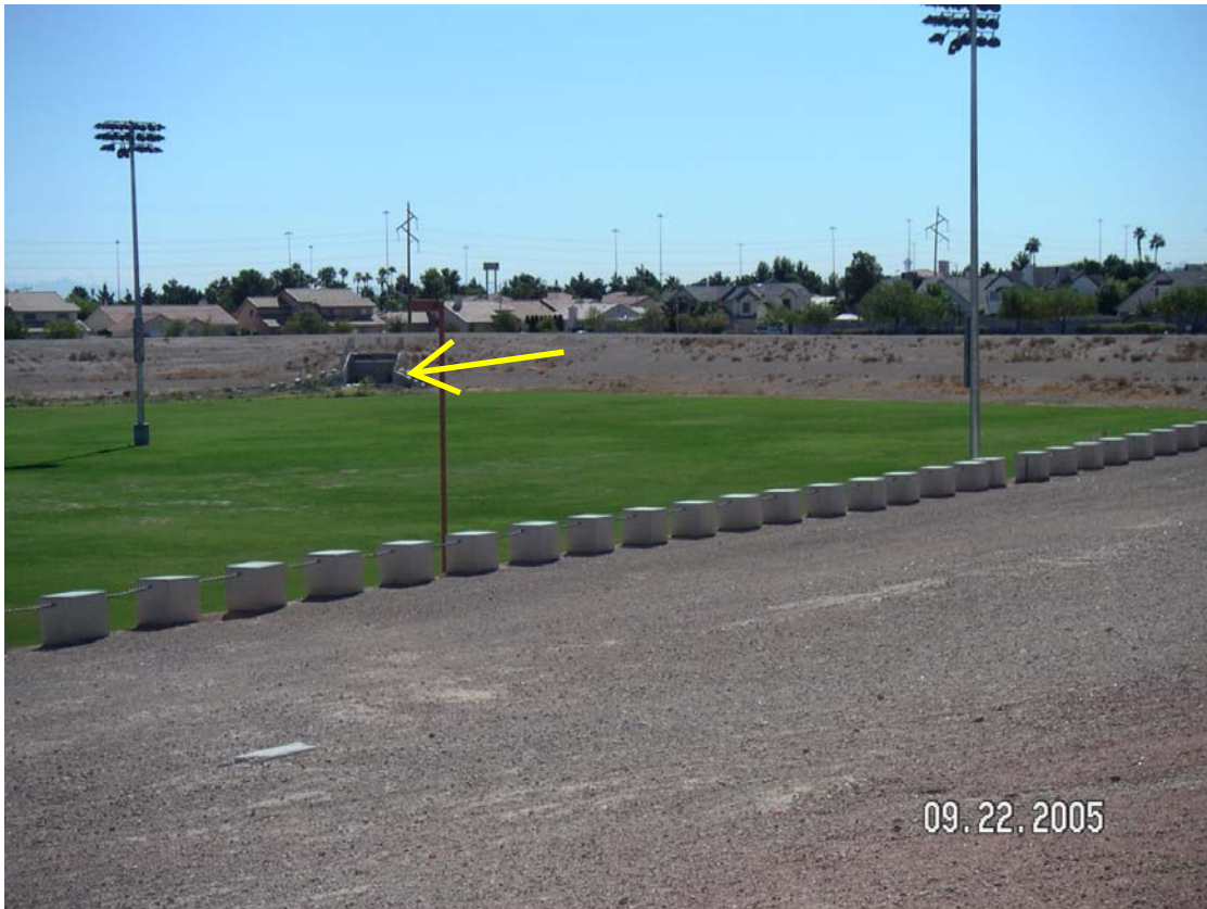
Photo 1. Gowan Detention Basin - inlet.
