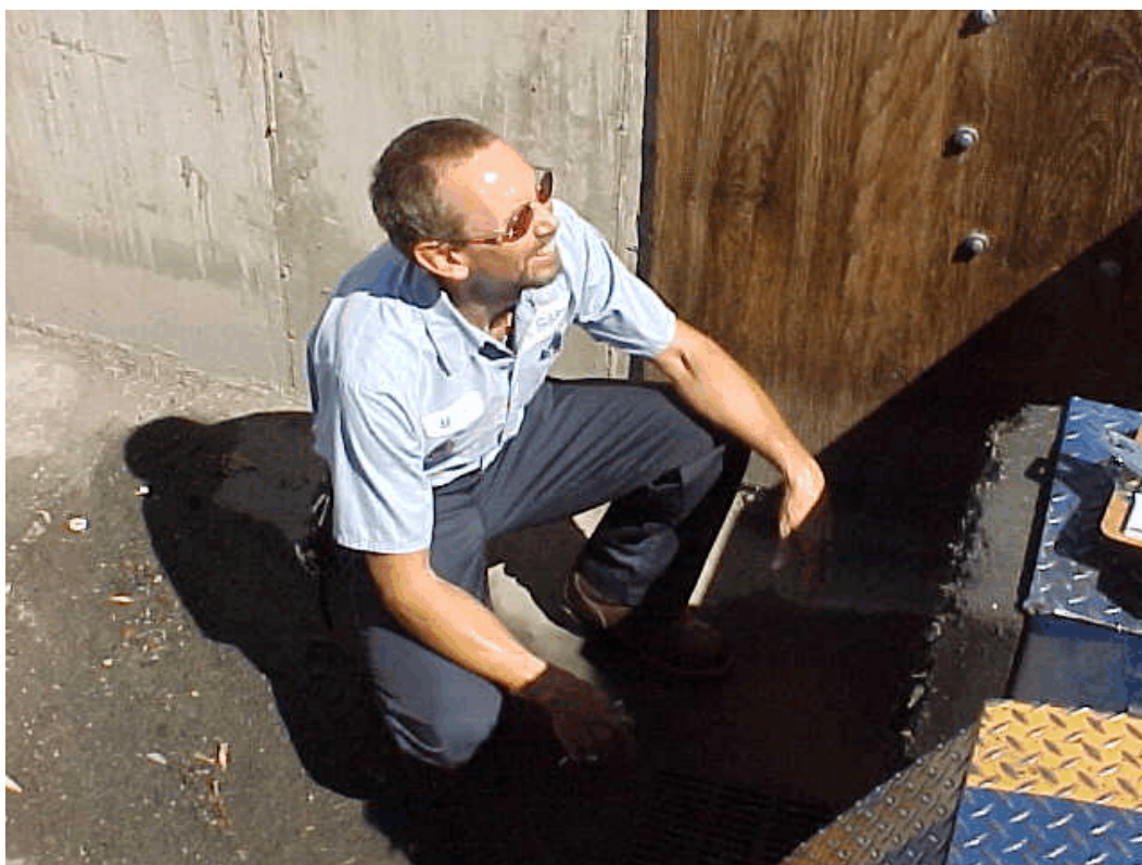
Photo 4. Mr. Palsgrove inspecting loading dock and dead sump for collection of storm water.
