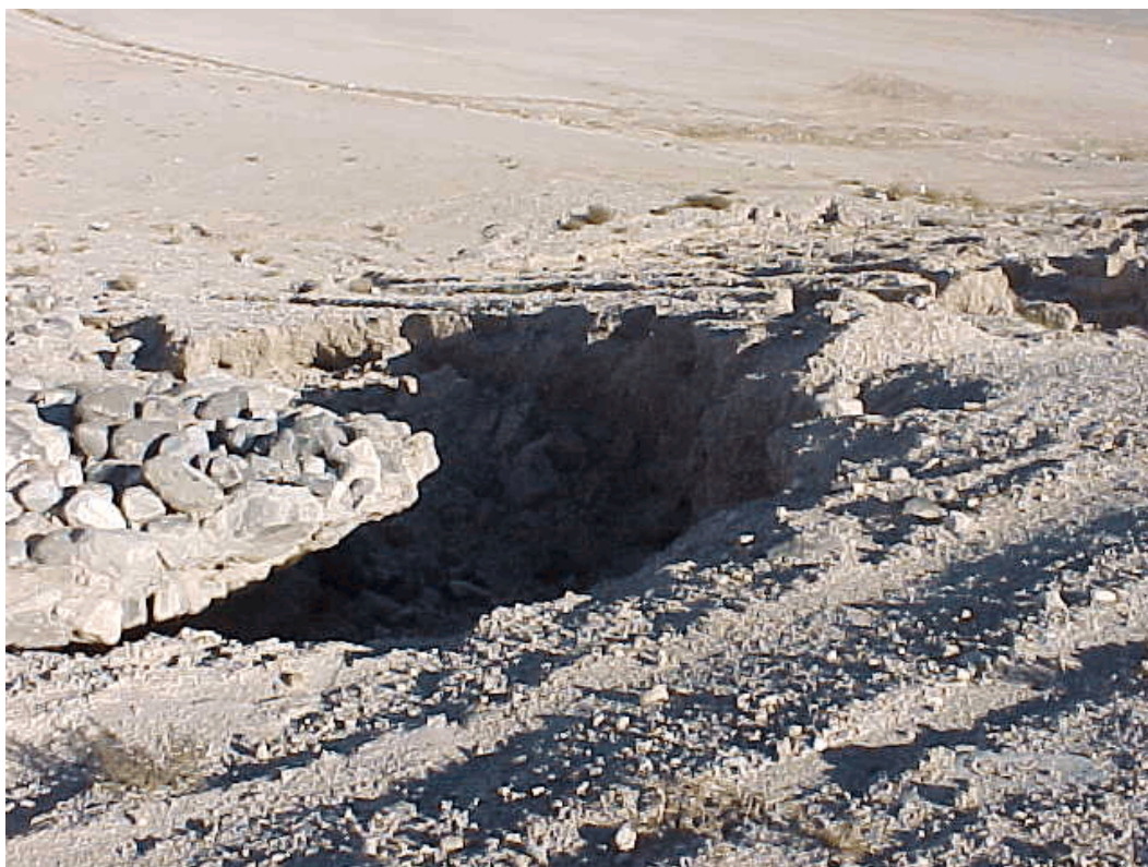
Photo 9. Erosion on west wall of detention basin.
