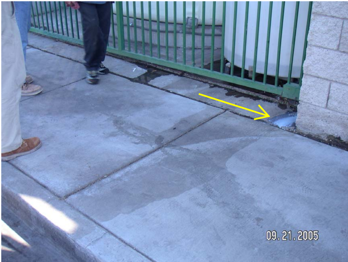
Photo 9. Discharge to street from leaking tank.
