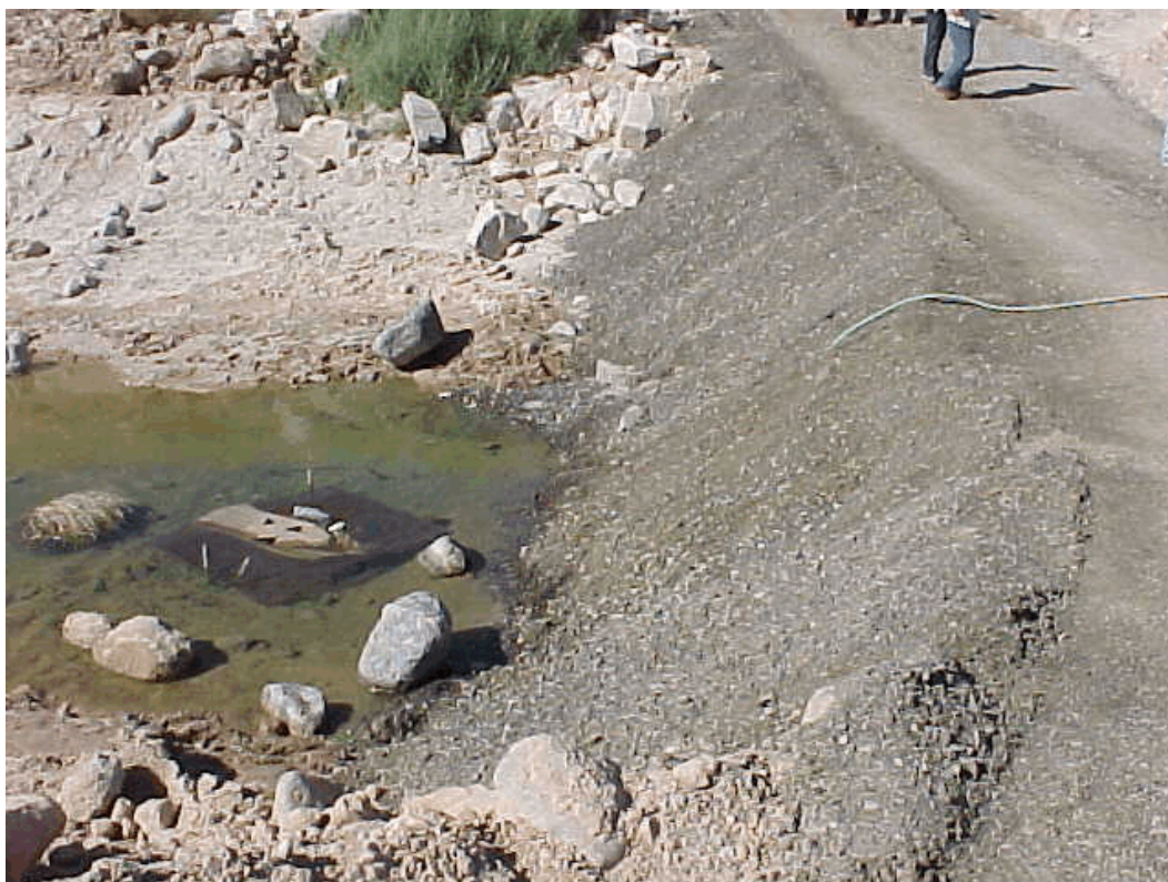
Photo 1. Diversion inlet (photo left) and earthen dam.
