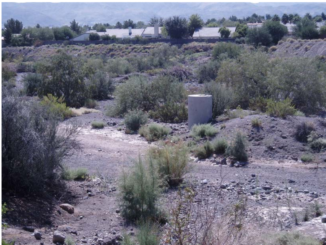
Photo 3. Project Green, elevated manhole in photo center.
