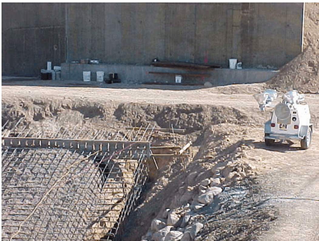
Photo 2. Downstream side of earthen dam. Note concrete runoff on face of dam. Note 5-gallon pails of chemicals along the retaining wall.
