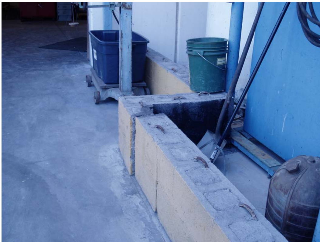
Photo 1. Crack in secondary containment.
