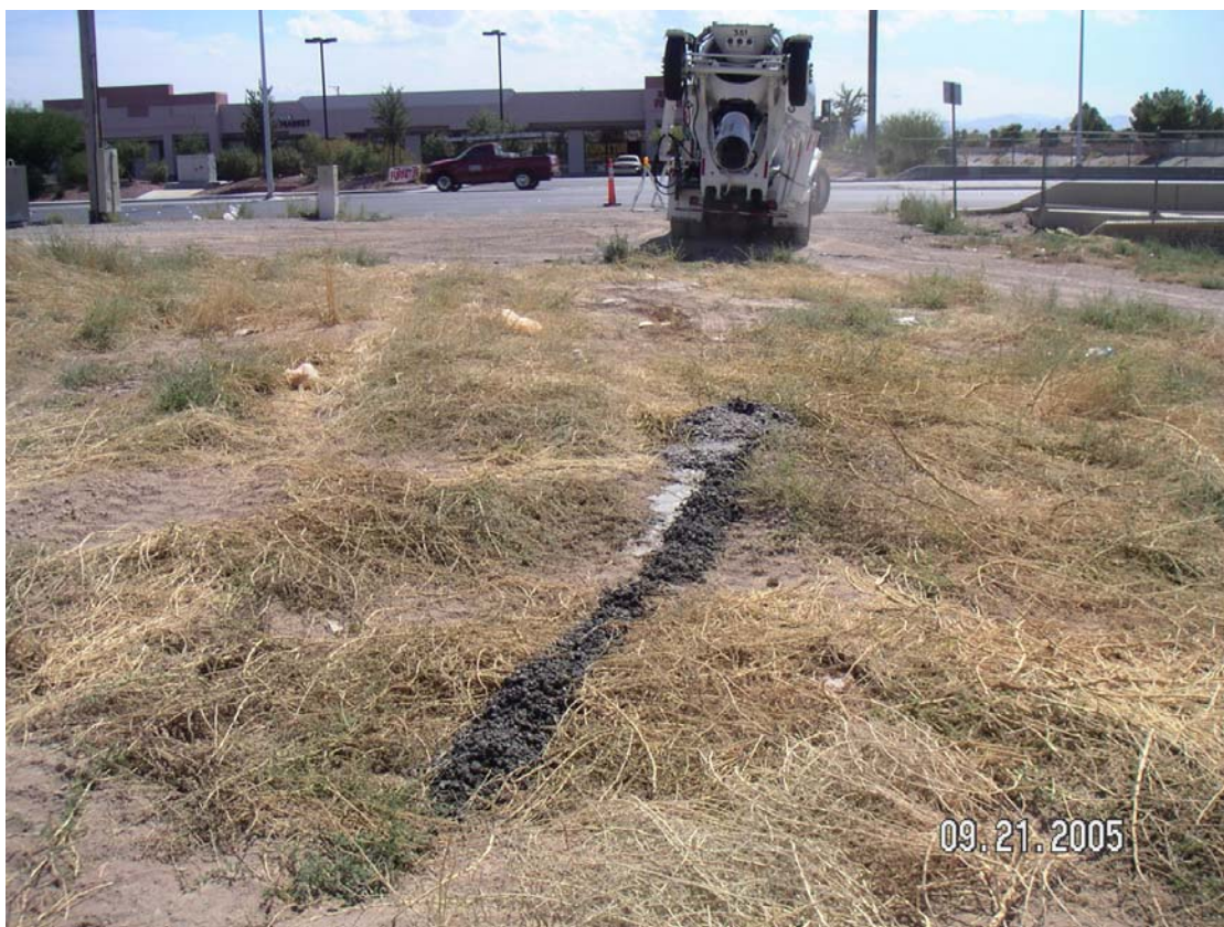
Photo 2. Wash-out material left by concrete truck.
