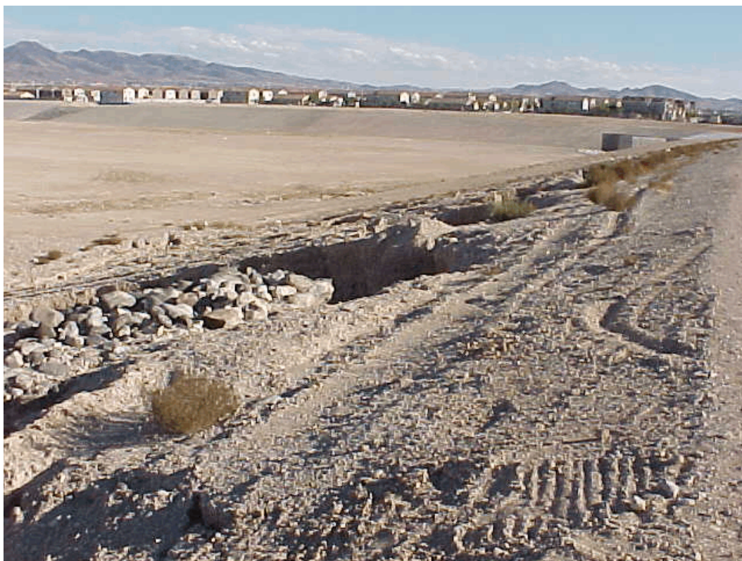
Photo 8. Erosion on west wall of detention basin.
