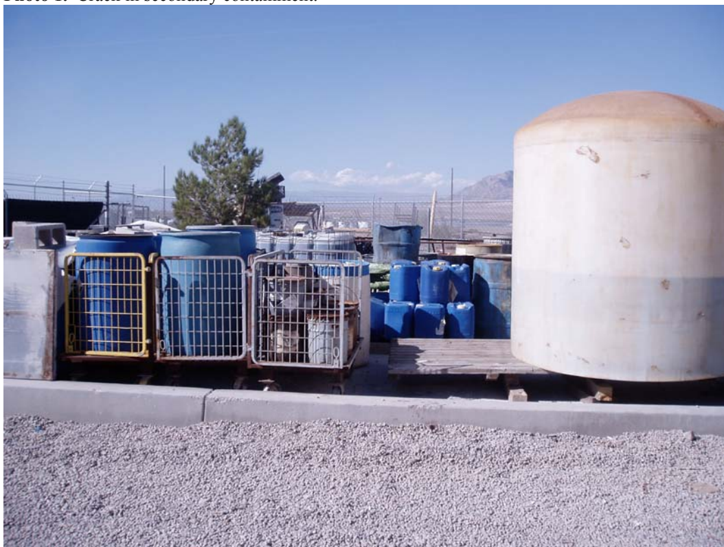
Photo 2. Berm area for chemical storage.
