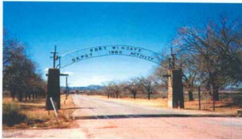
Fort Wingate Depot Area Entrance
