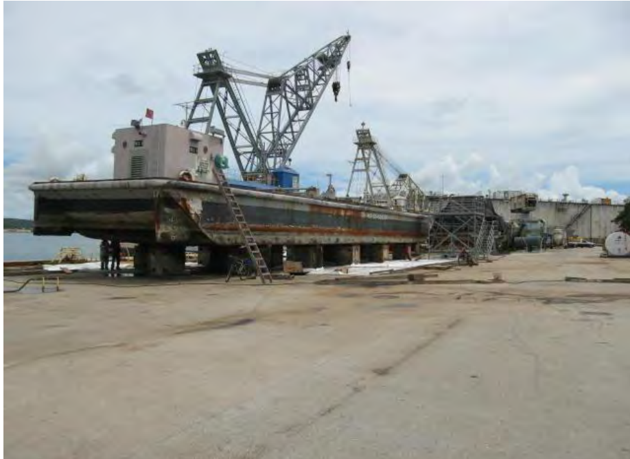
Photo 7 – Barge undergoing work Shoreside. Note hosing to left and puddled water nearby.
