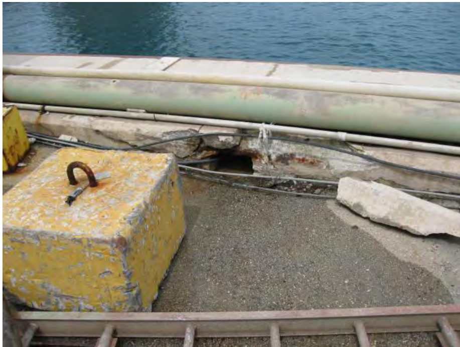
Photo 8 – Evidence of discharge of non-stormwater to harbor from a scupper immediately adjacent to the where a barge was undergoing work onshore.
