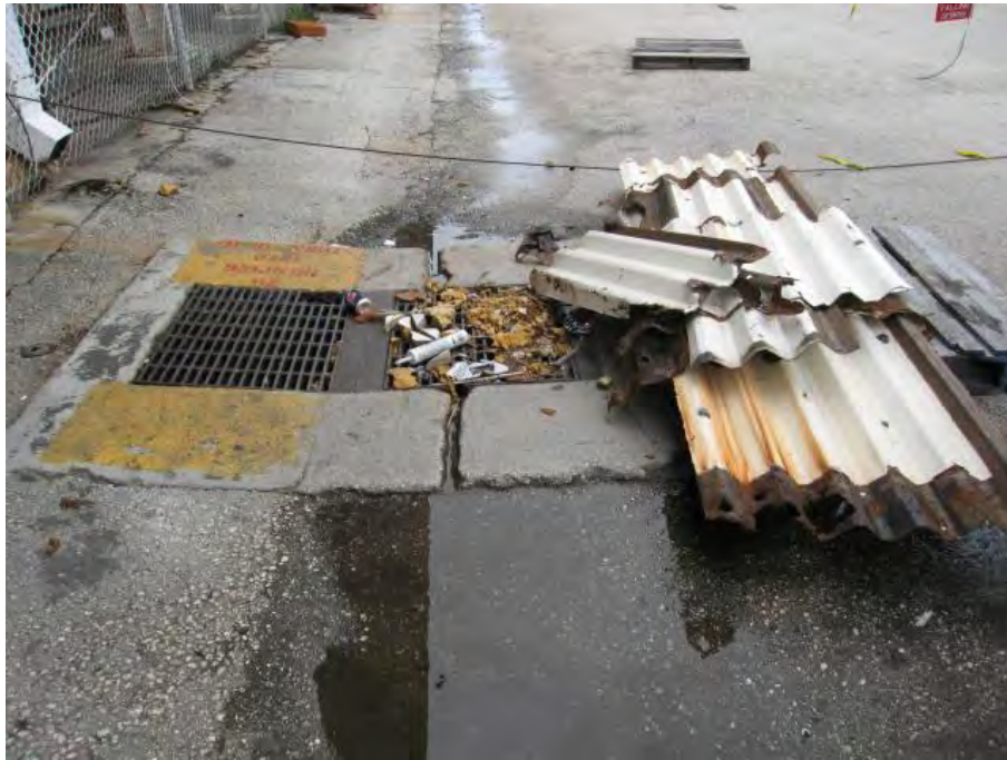
Photo 5 – Accumulated debris on top of drain inlet located outside of electrical shop
