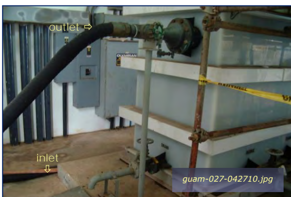
Photo #3-9: Papa Wharf - Bilge Oily Water Separator Taken By: Greg V. Arthur Date: 04/27/10
