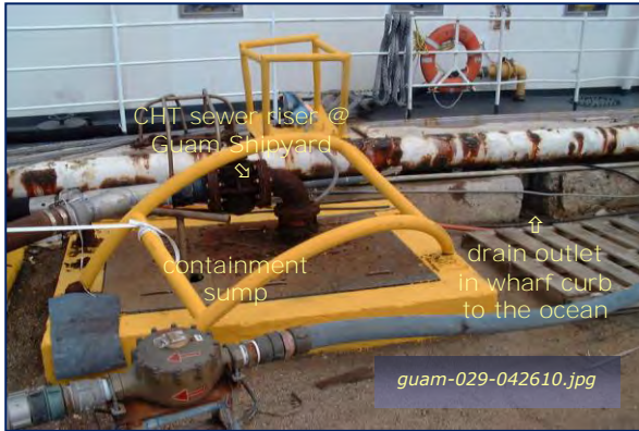
Photo #3-1: Oscar Wharf - CHT Sewer Riser Taken By: Greg V. Arthur Date: 04/26/10
