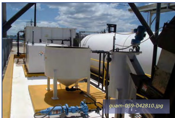
Photo #3-13: Beta Wharf – Curbing Around BOWTS Taken By: Greg V. Arthur Date: 04/28/10
