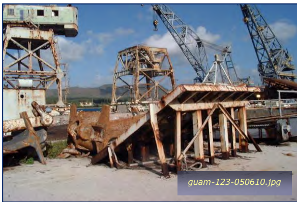
Photo #3-18: Finger Pier – Scrapyard Taken By: Greg V. Arthur Date: 05/06/10
