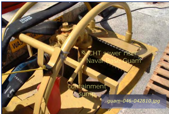
Photo #3-3: Sierra Wharf - CHT Sewer Riser Taken By: Greg V. Arthur Date: 04/28/10
