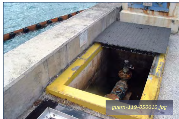
Photo #3-6: Victor Wharf - Bilge Pump Station Riser Taken By: Greg V. Arthur Date: 05/06/10
