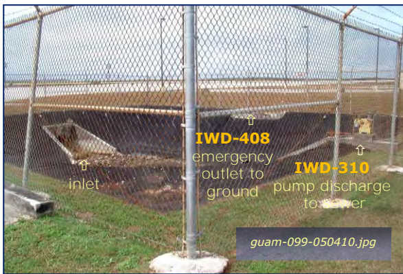
Photo #1-21: Bldg 2641 – HSC-25 Catchment Pit Taken By: Greg V. Arthur Date: 05/04/10
