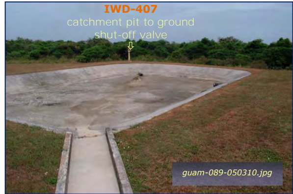
Photo #1-14: Bldg 19017 – Catchment Pit Taken By: Greg V. Arthur Date: 05/03/10
