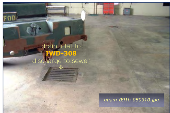
Photo #1-18: Bldg 21008 – Southside Drain Inlet Taken By: Greg V. Arthur Date: 05/03/10
