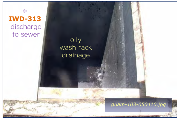
Photo #1-26: Bldg 18001 – Pit Prior to Oil Water Sep Taken By: Greg V. Arthur Date: 05/04/10
