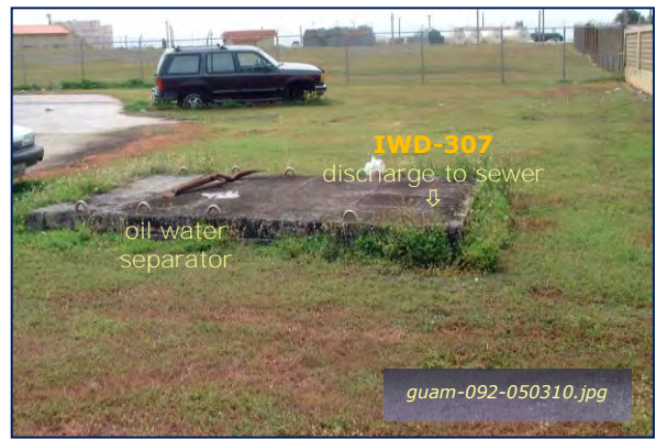
Photo #1-16: Bldg 26051 – Oil Water Separator Taken By: Greg V. Arthur Date: 05/03/10
