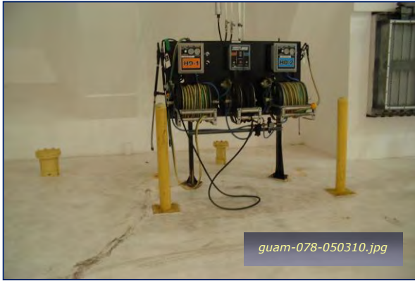
Photo #1-1: Hanger 2 - Aircraft Wash Stand Taken By: Greg V. Arthur Date: 05/03/10
