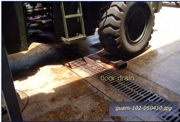
Photo #1-25: Bldg 18001 – Wash Rack Drains Taken By: Greg V. Arthur Date: 05/04/10
