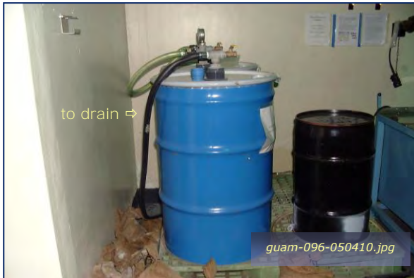
Photo #1-19: Bldg 17006 – NDT Holding Drums Taken By: Greg V. Arthur Date: 05/04/10
