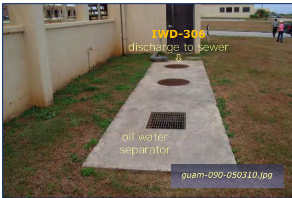
Photo #1-15: Bldg 18040 – Oil Water Separator Taken By: Greg V. Arthur Date: 05/03/10
