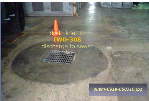
Photo #1-17: Bldg 21008 – Northside Drain Inlet Taken By: Greg V. Arthur Date: 05/03/10
