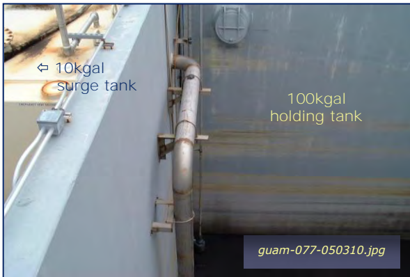
Photo #1-3: Hanger 2 - Holding and Surge Tanks Taken By: Greg V. Arthur Date: 05/03/10
