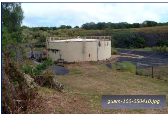
Photo #1-23: Andersen AFB Landfill – Holding Tank Taken By: Greg V. Arthur Date: 05/04/10
