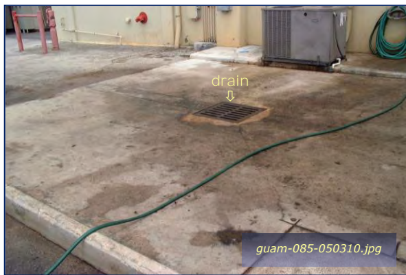
Photo #1-9: Bldg 18004 – Ground Support Washrack Taken By: Greg V. Arthur Date: 05/03/10
