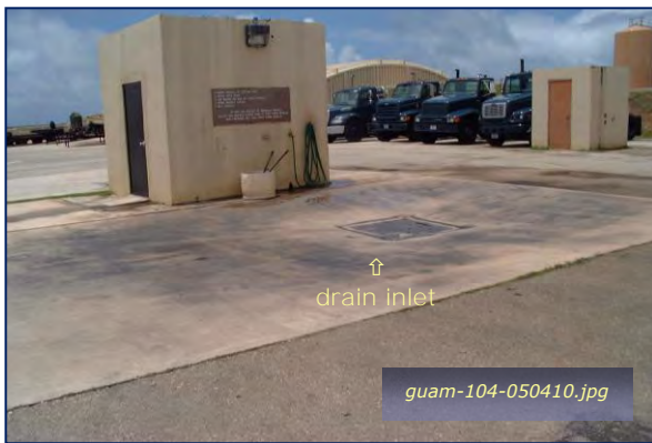
Photo #1-27: Bldg 18035 – Outdoor Wash Rack Taken By: Greg V. Arthur Date: 05/04/10
