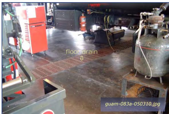
Photo #1-11: Bldg 26229 – Floor Drains Taken By: Greg V. Arthur Date: 05/03/10
