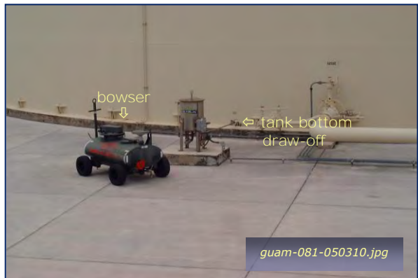
Photo #1-6: Tank Bottoms Draw-off to Bowser Taken By: Greg V. Arthur Date: 05/03/10
