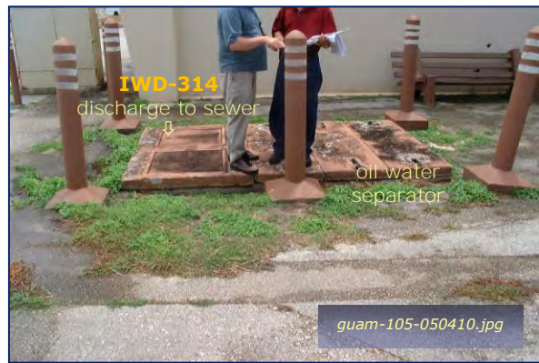
Photo #1-28: Bldg 18035 – Oil Water Separator Taken By: Greg V. Arthur Date: 05/04/10
