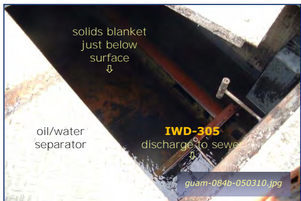
Photo #1-12: Bldg 26229 – Oil Water Separator Taken By: Greg V. Arthur Date: 05/03/10
