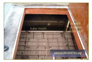
Photo #1-1: Mesh Tube Coalescing Oil Water Sep
