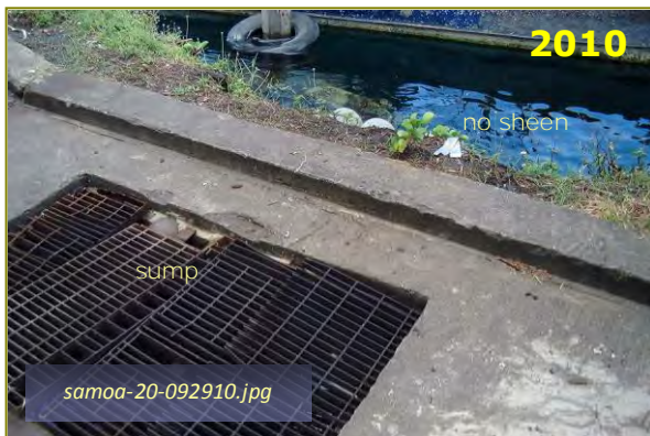
Photo #13: Discharge Sump 002 - Sept 2010 Taken By: Greg V. Arthur Date: 09/29/10
