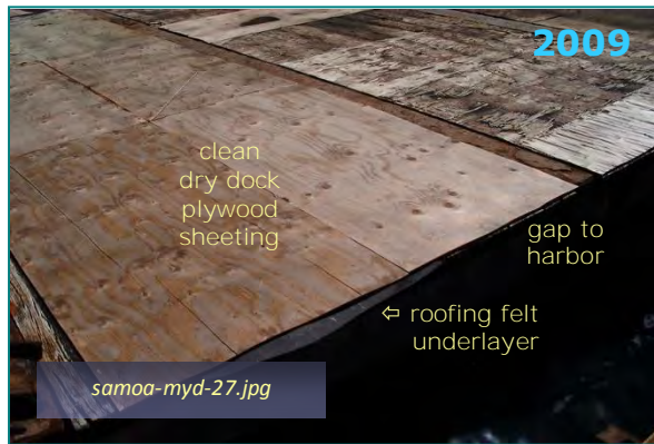
Photo #4: 3000-Ton Dry Dock Decking – April 2009 Taken By: Greg V. Arthur Date: 04/27/09
