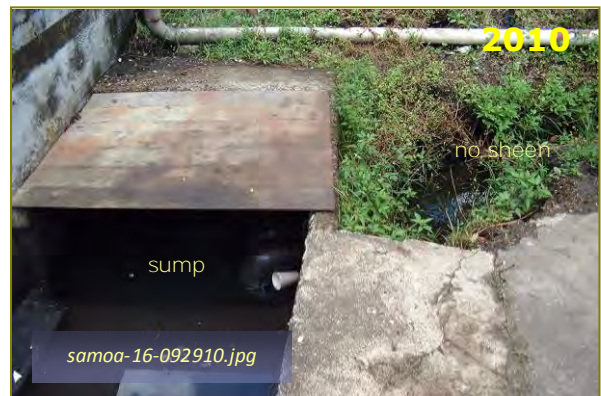
Photo #14: Discharge Sump 003 - Sept 2010 Taken By: Greg V. Arthur Date: 09/29/10
