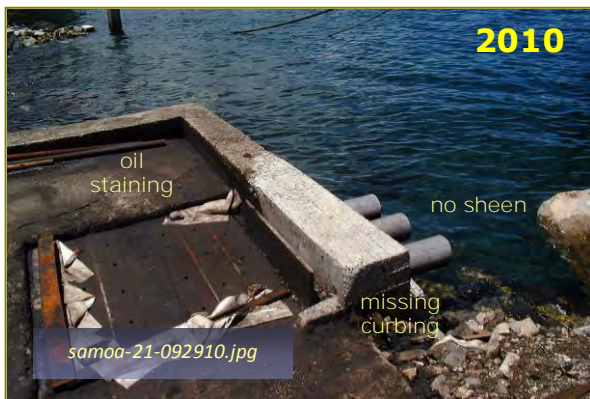
Photo #11: Catch Basin #1 - discharge sump 001 Taken By: Greg V. Arthur Date: 09/29/10
