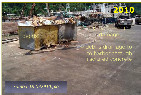
Photo #5: Catch Basin #3 – South Dock Taken By: Greg V. Arthur Date: 09/29/10
