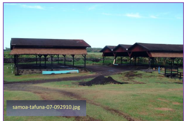
Photo #6: Tafuna STP – Sludge Drying Beds No.2 Taken By: Greg V. Arthur Date: 09/29/10
