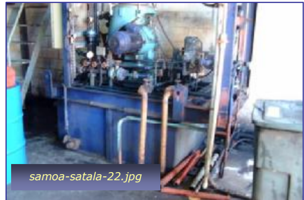
Photo #2: One of Four Lube Oil Centrifuges Taken By: Greg V. Arthur Date: 04/30/09
