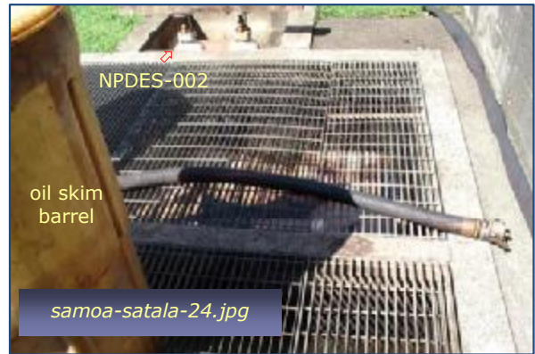
Photo #8: NPDES Sump #2 - Western Oil Water Sep Taken By: Greg V. Arthur Date: 04/30/09
