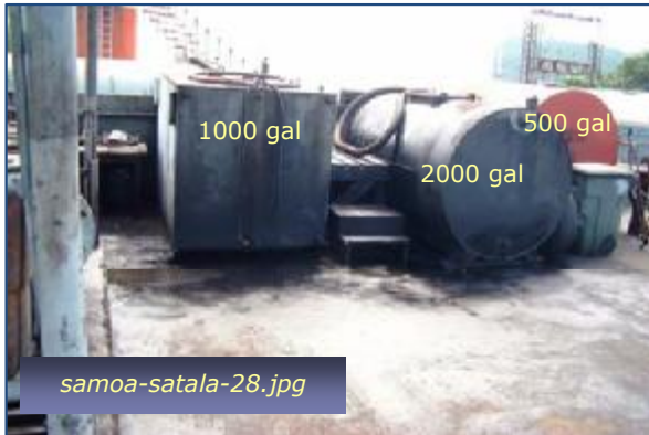
Photo #13: Waste Oil Step 1 - Batch Settling Tanks Taken By: Greg V. Arthur Date: 04/30/09
