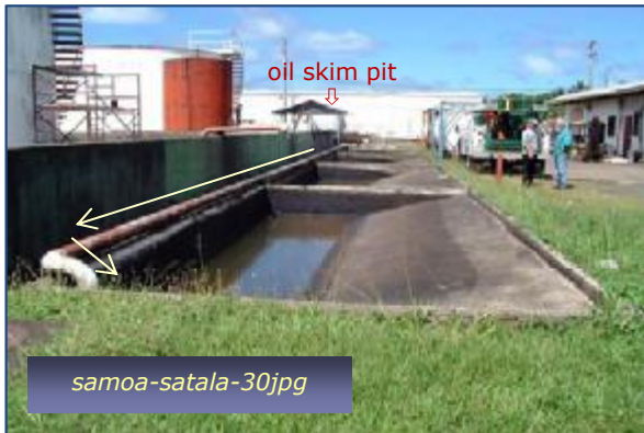
Photo #15: Waste Oil Step 3 - Settling Basins Taken By: Greg V. Arthur Date: 04/30/09
