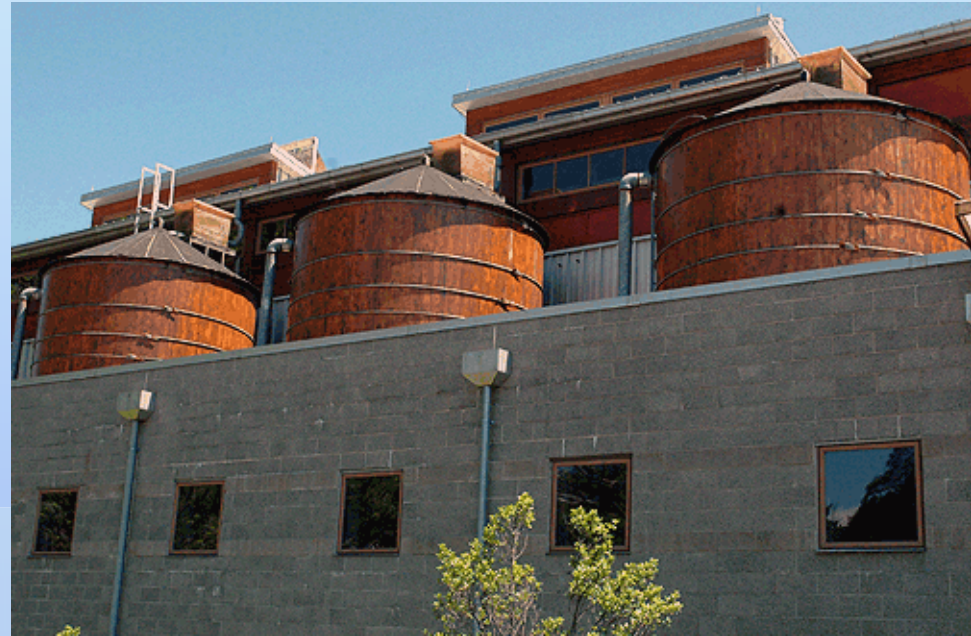
Philip Merrill Building cisterns. Photo: Chesapeake Bay Foundation.
