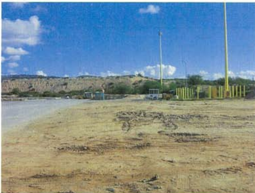
Photograph 6: View of Pier 7 showing a portion of the disturbed area associated with lighting improvements (looking northeast)
