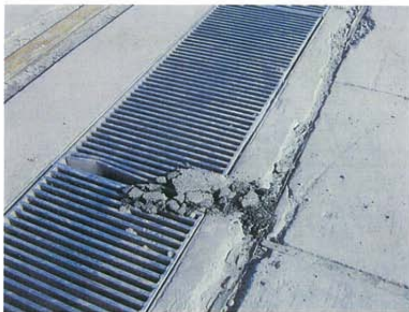
Photograph 12: View of location shown in Photograph 11
