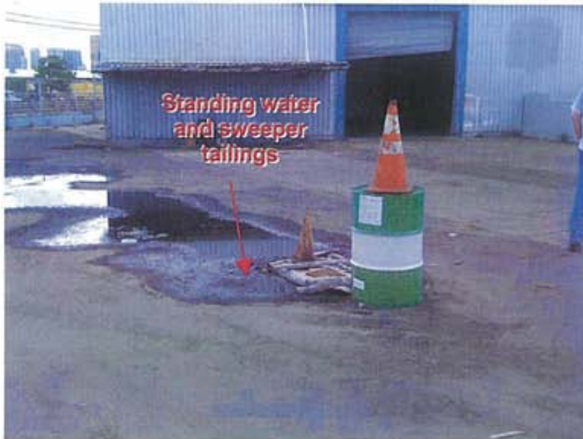
Photograph 3: Evidence of previous sweeper washout activity, including standing water and sweeper tailings near the storm drain inlet
