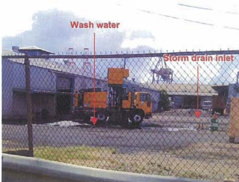
Photograph 1: At Honolulu Harbor – Pier 34, a HDOT maintenance crew was observed washing out a street sweeper bin adjacent to a storm drain inlet
