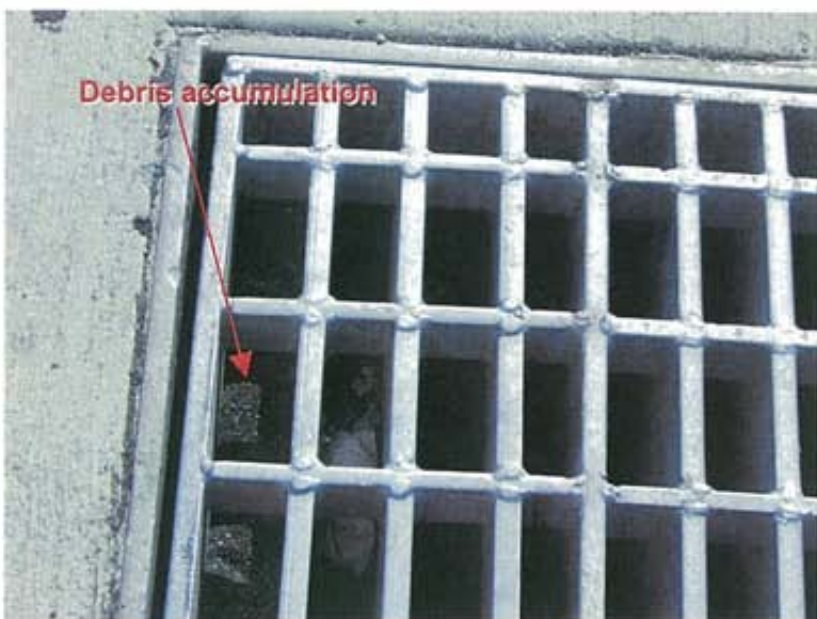
Photograph 20: View inside trench drain shown in Photograph 18
