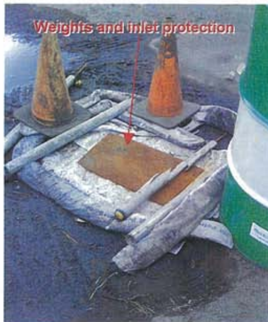
Photograph 4: View of storm drain inlet that was not adequately protected
