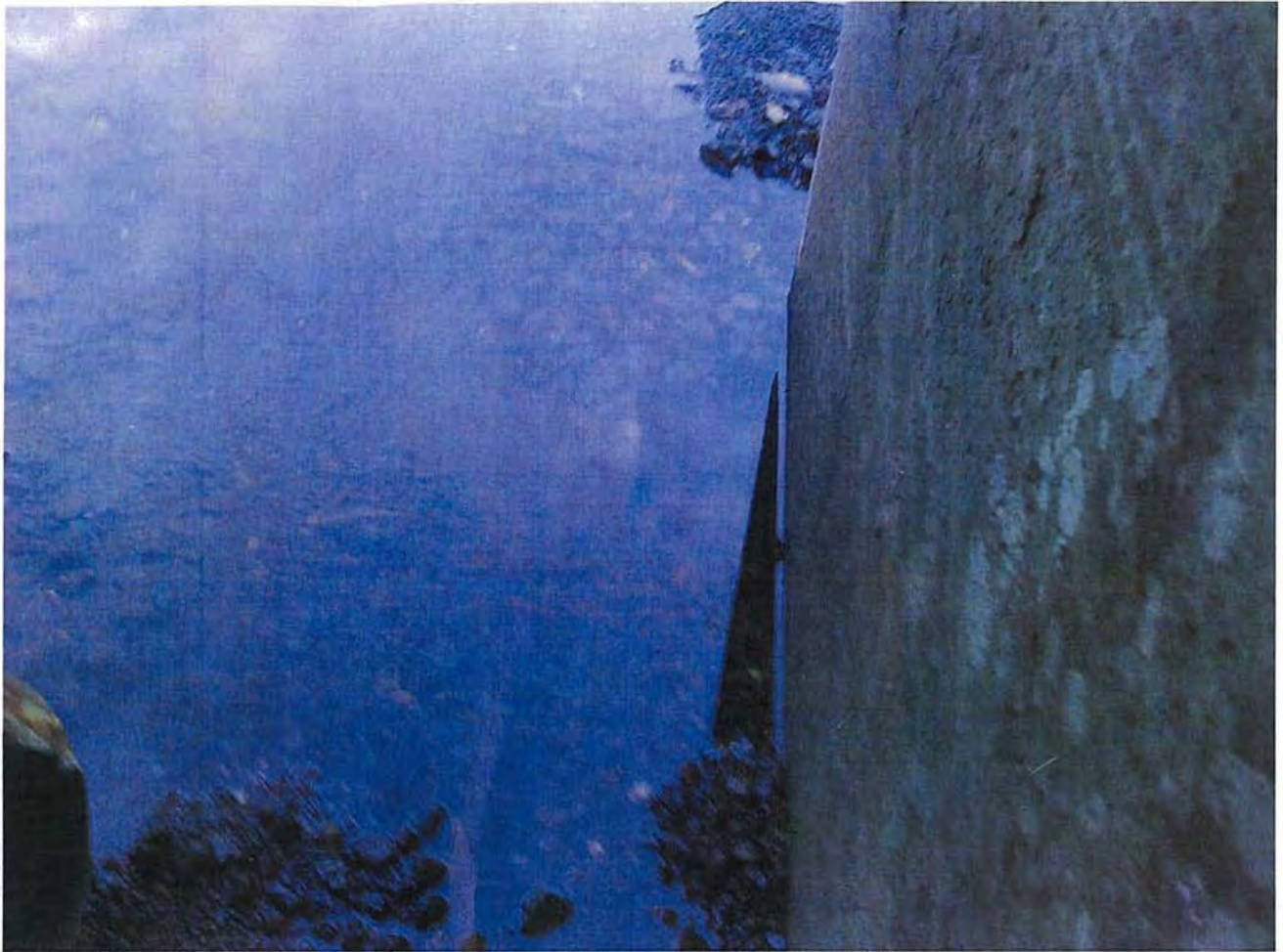
Electrochem cut storm drain 12-9-10
