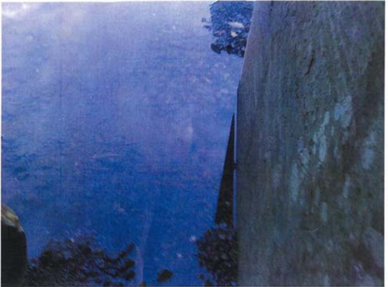
Electrochem cut storm drain 12-9-10
