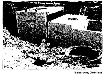
Crews install the 'Storm Vault' water treatment system at the City of Reno's Corporation Yard recently. The vault is intended to reduce water pollution.
