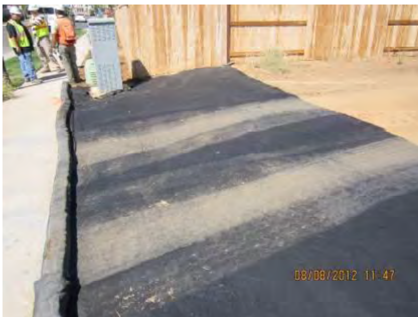
Photograph 3. Close-up view of area used for vehicle access shown in Photograph 2.
