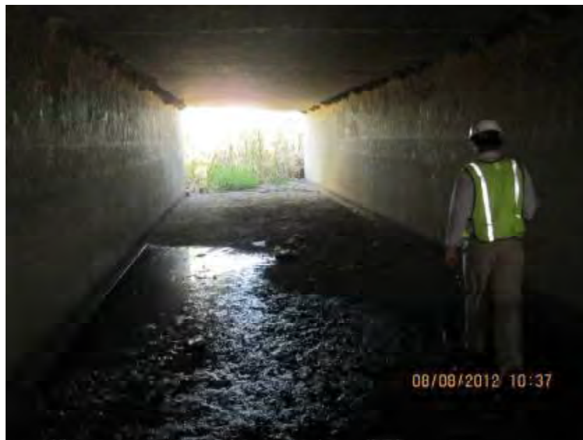
Photograph 2. View of box culvert access to outfall.
