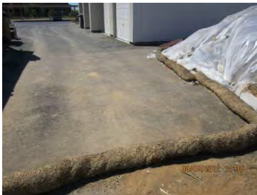
Photograph 4. Additional example of stockpile surrounded by straw wattles which were not entrenched into the ground.
