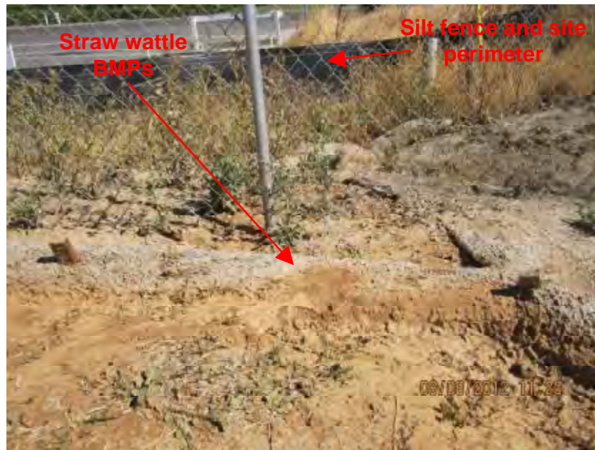
Photograph 6. Close-up view of straw wattle which had accumulated sediment to its full height.
