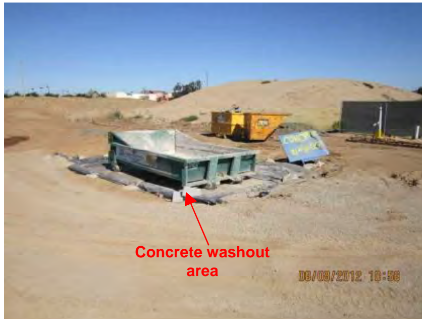
Photograph 1. View of concrete washout area at the construction site.
