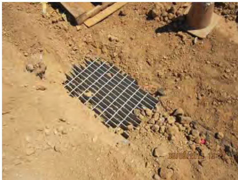
Photograph 7. Laguna Corporate Center Construction Project – Close-up view of storm drain inlet shown in Photograph 6.
