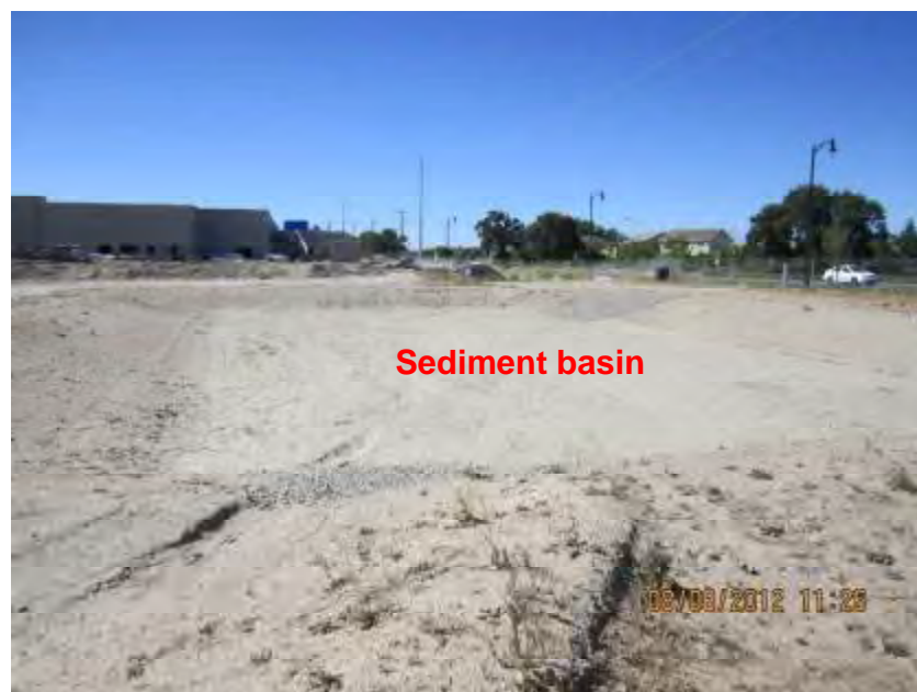
Photograph 2. View of temporary sediment basin near the northwest corner of the site.
