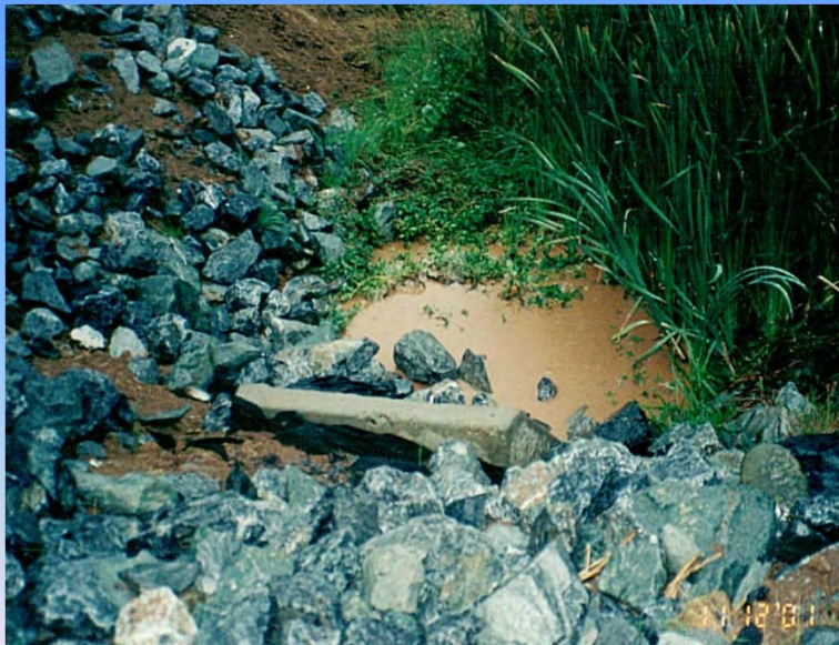
...and outfalls to a drainage ditch or channel.
