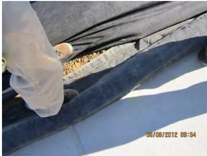
Photograph 2. View of “heavy weight wattle” sediment control BMP which was not entrenched into the ground.
