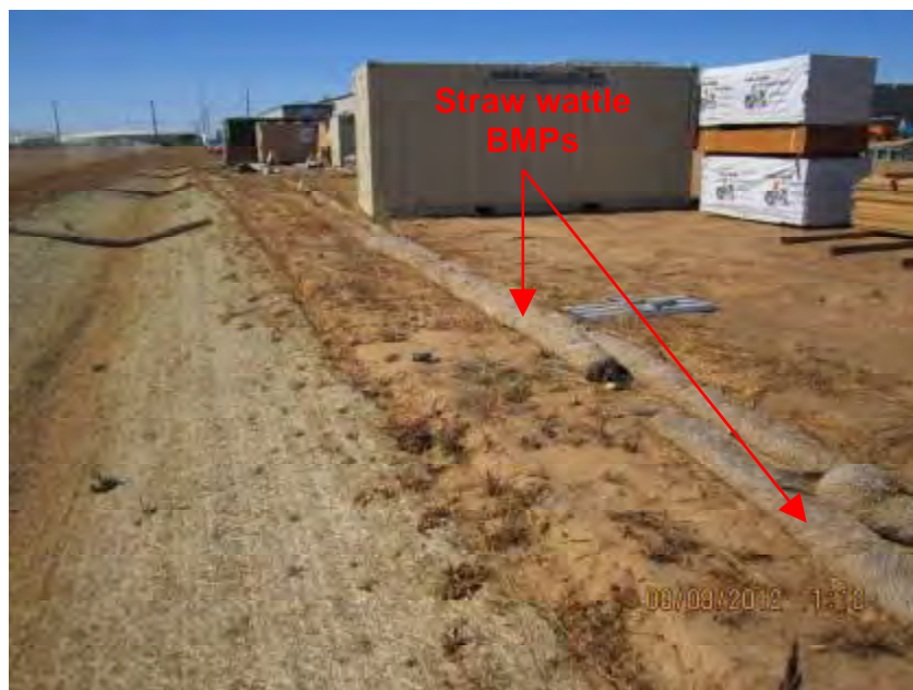
Photograph 3. View of straw wattle BMPs installed along the eastern edge of the site. Note that the straw wattles were not entrenched into the ground.
