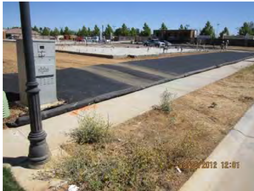
Photograph 2. View of area with geotextile coverage that was used for vehicle access.
