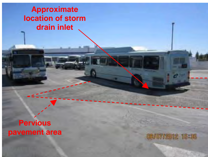
Photograph 6. View of bus parked over a storm drain inlet in an area of pervious pavement.
