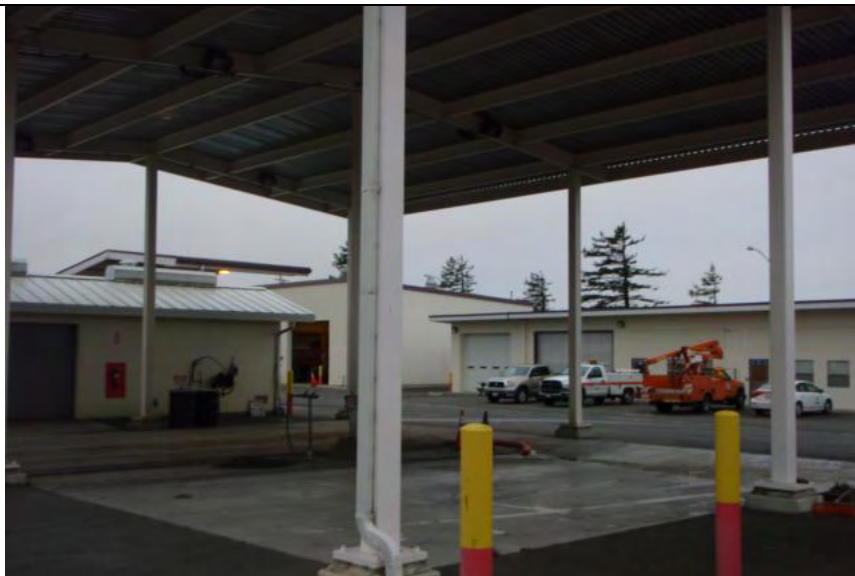
Photograph 1 – Covered wash rack
