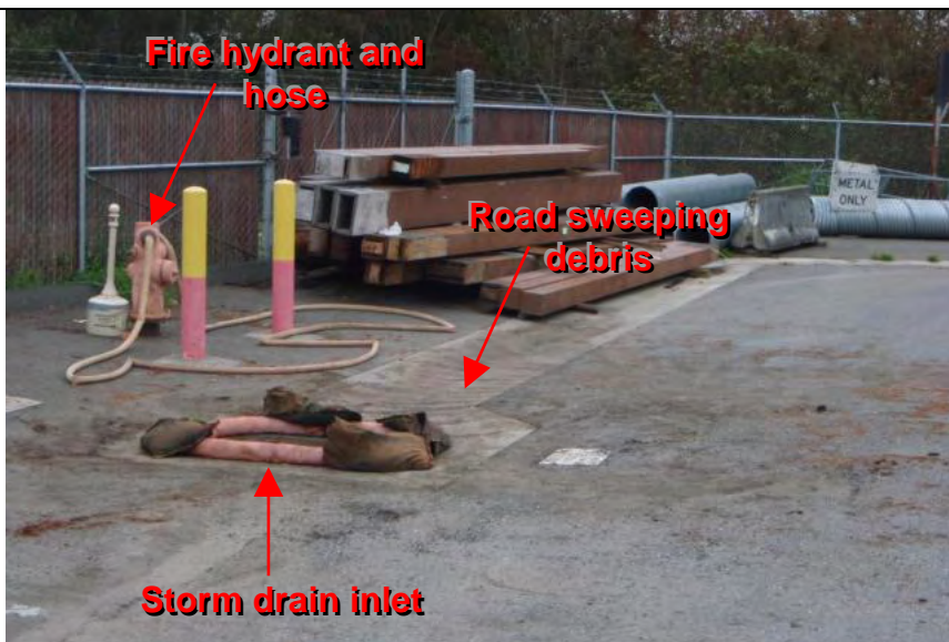
Photograph 3 – Area in northwest corner of facility used for road sweeper washing. (Note: Pollutant accumulation around storm drain inlet)
