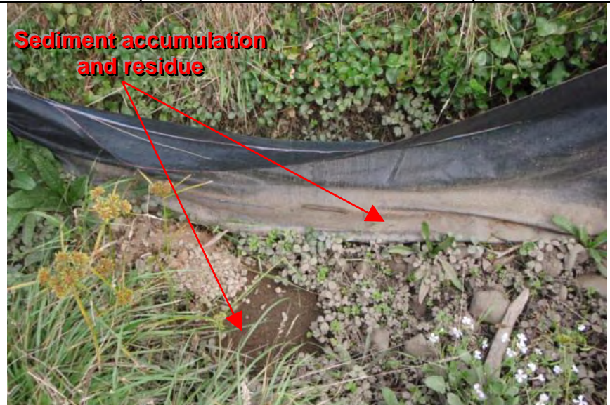
Photograph 4 – Closer view of silt fence BMP shown in Photograph 3
