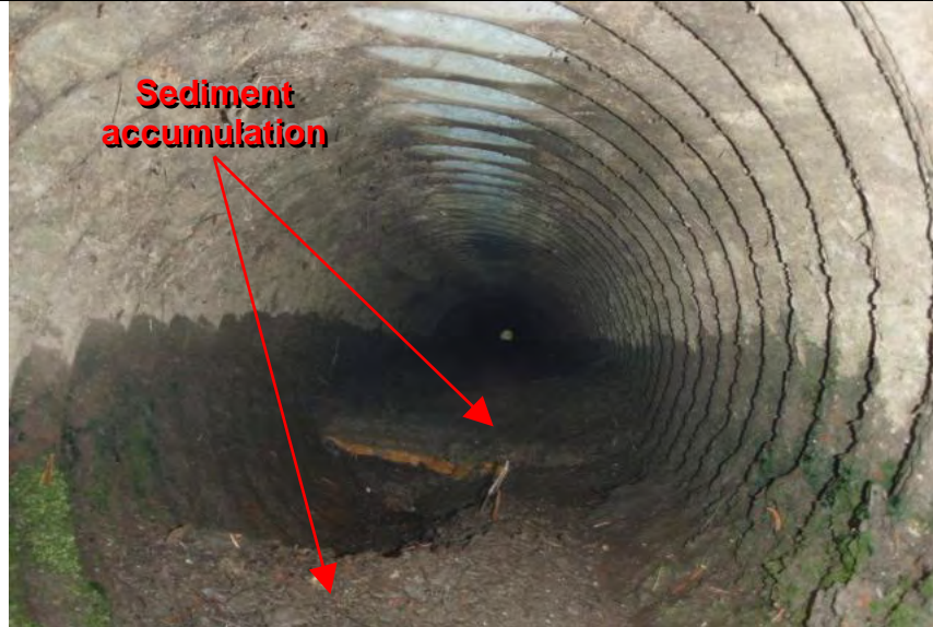
Photograph 5— View into storm drain pipe from outlet
