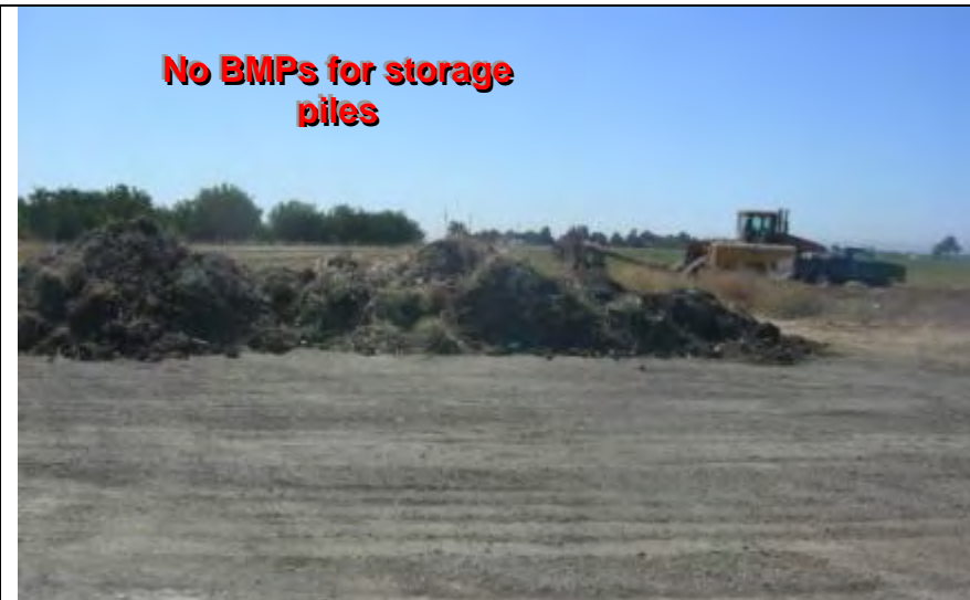
Photograph 2 – Lack of BMPs to contain stockpiled soils from tree removal
