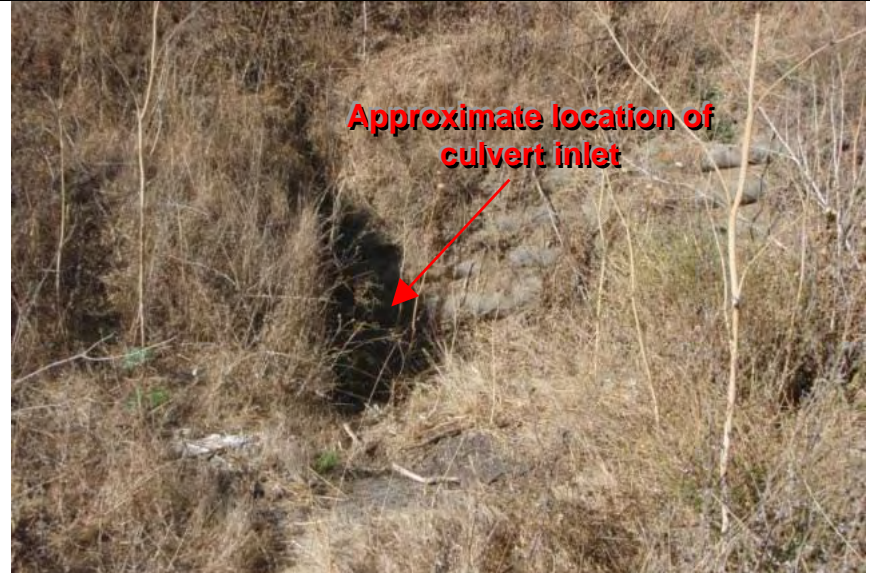
Photograph 6 – Location of culvert inlet in the northwestern portion of the waste storage site
