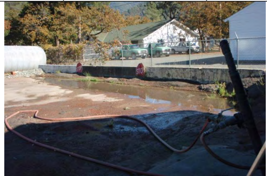
Photograph 12 – Bermed area used for truck bed washing
