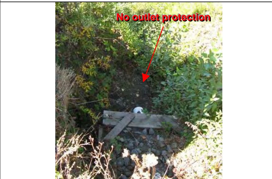
Photograph 11— Outlet pipe down-gradient of facility outfall
