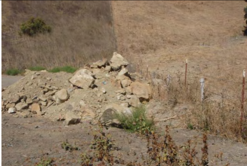
Photograph 5 – Note lack of BMPs for containment around stockpile and the stockpile's proximity to the fenceline
