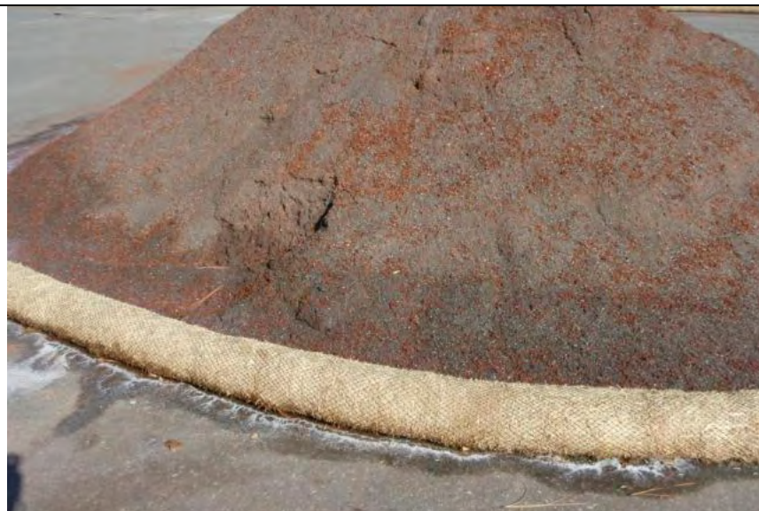
Photograph 7— Closer view of straw wattle BMP around stockpile (Note: Apparent salt residue)
