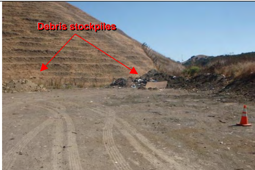
Photograph 2 –Lack of BMPs for containment or coverage of stockpiles
