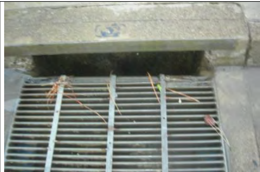
Photograph 2 – Storm drain from Photograph 1
