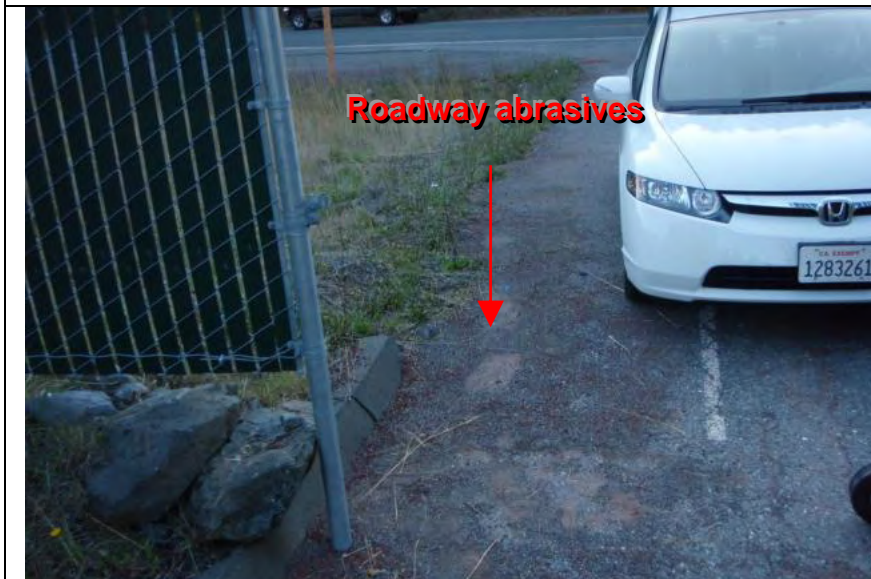
Photograph 7— Roadway abrasives outside facility entrance
