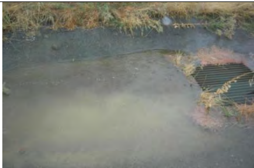
Photograph 4 – Storm drain inlet adjacent to temporary storage area
