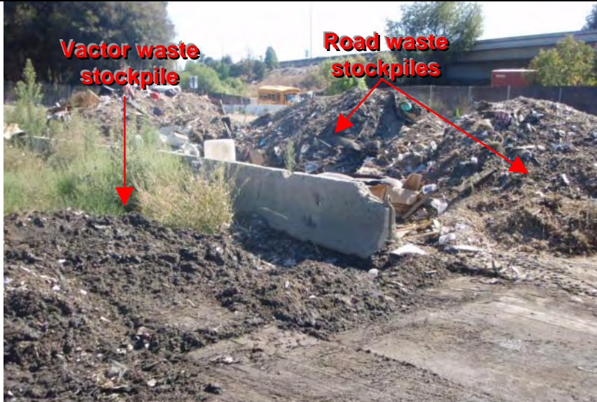
Photograph 3 – Lack of BMPs for containment or coverage of road waste stockpiles
