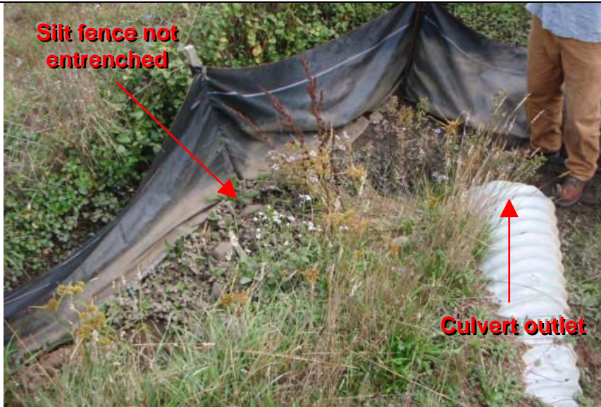
Photograph 3 – Storm drain outlet to drainage ditch in southeast corner of facility
