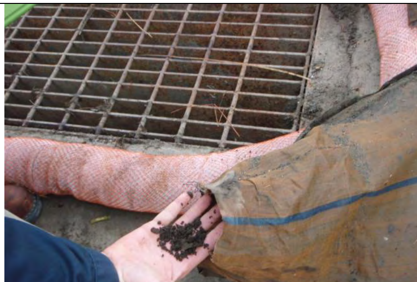
Photograph 6 – View of debris contained in bags used for securing absorbent booms
