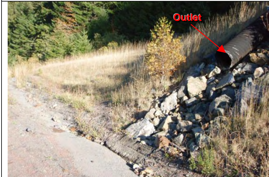
Photograph 3 – Discharge location from inlet shown in Photograph 2
