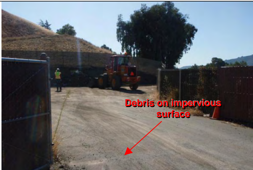
Photograph 1 – Entrance to temporary storage site. (Note: Impervious roadway entrance and tracking of debris)
