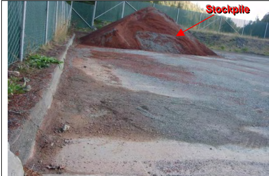
Photograph 1 – Stockpile without BMPs for coverage or containment
