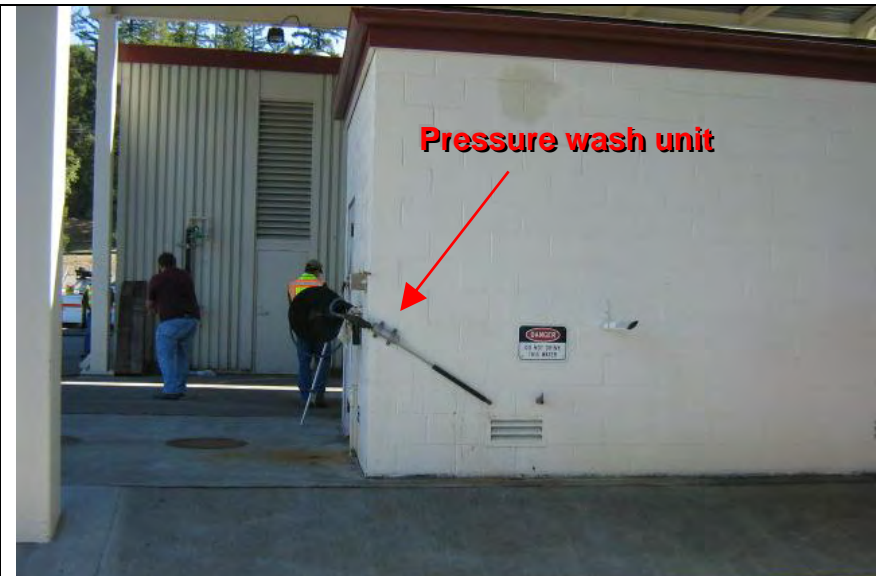
Photograph 1 – Covered wash rack
