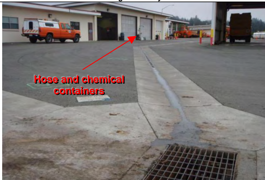
Photograph 12— View from down-gradient storm drain inlet to location of hose and chemical containers pictured in Photograph 11
