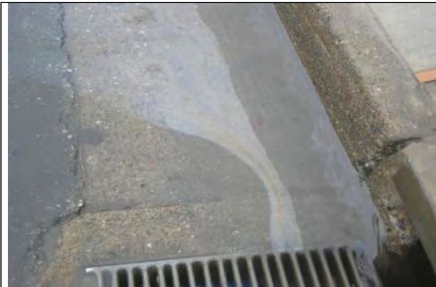
Photograph 1 – Visible sheen entering storm drain
