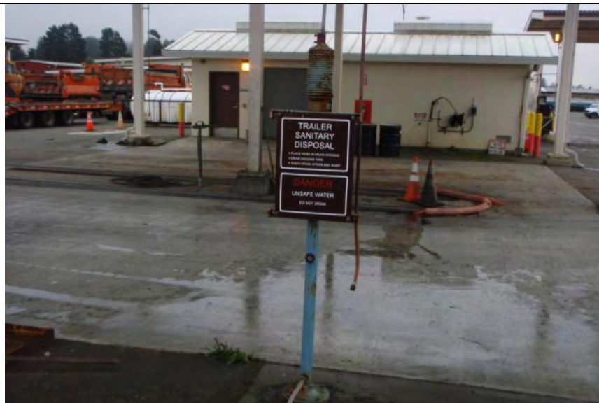
Photograph 2 – Another view of covered wash rack
