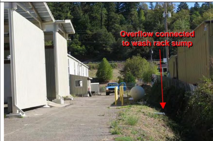
Photograph 3 – Sump overflow leading to drainage ditch
