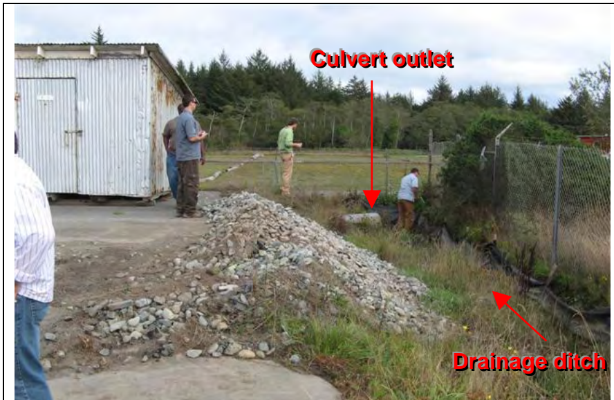
Photograph 9— View of drainage ditch and storm drain system culvert outlet
