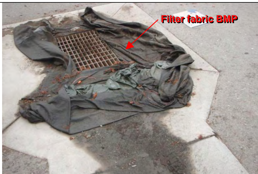
Photograph 4 – Second storm drain inlet near road sweeper washing area. Inlet is just out of the picture to the bottom left of Photograph 3.
