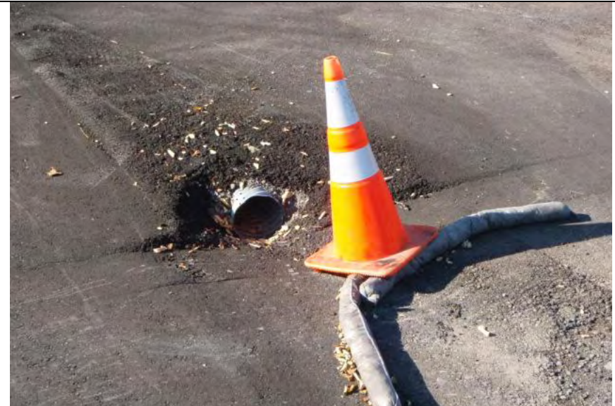
Photograph 2 – Culvert inlet that flows to northwest corner of facility
