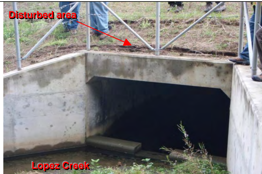
Photograph 10— Culvert crossing of Lopez Creek
