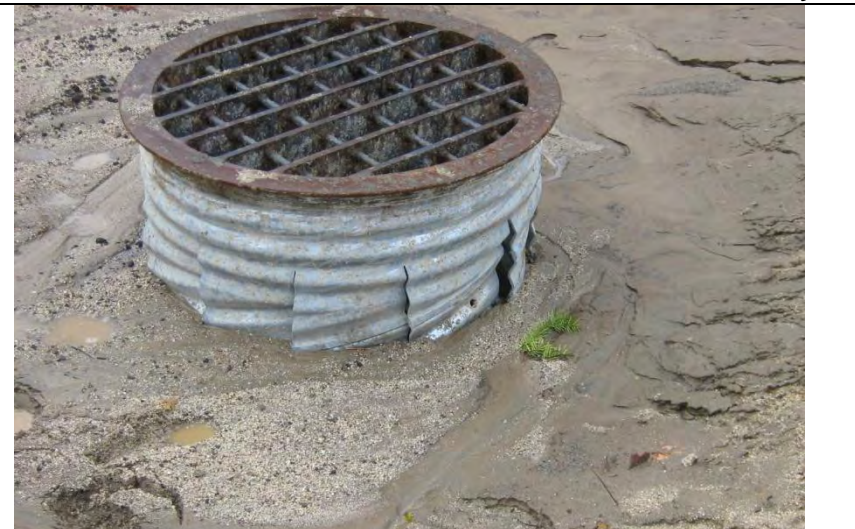
Photograph 12 – Close-up view of sediment basin No. 1 outlet structure with sediment accumulation
