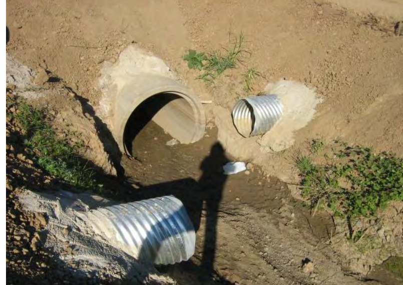
Photograph 8 – Culvert pipe outlet from Photograph 7 to irrigation channel.
