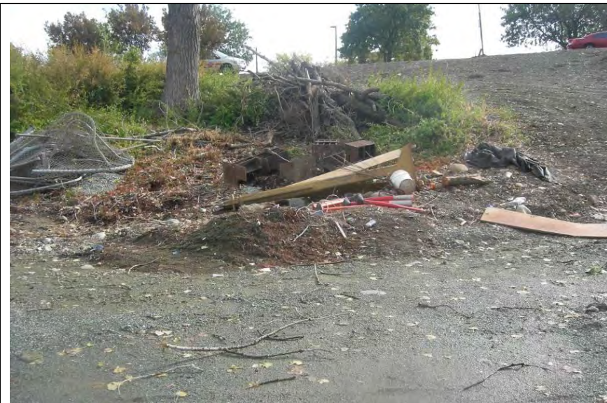
Photograph 5 – Lack of perimeter control BMPs around a construction material disposal stockpile
