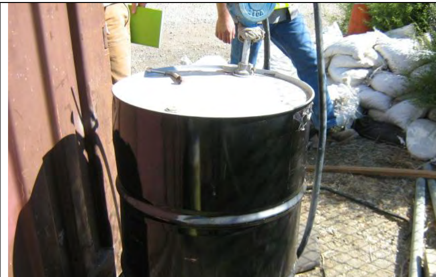
Photograph 6 – Asphalt release agent without secondary containment
