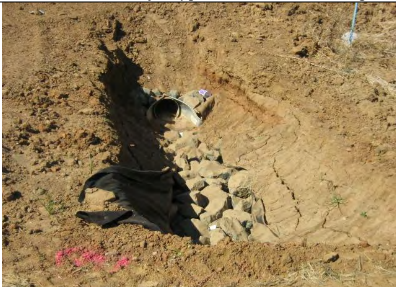
Photograph 7 – Drainage outlet at base of unstabilized slope shown in Photograph 6.
