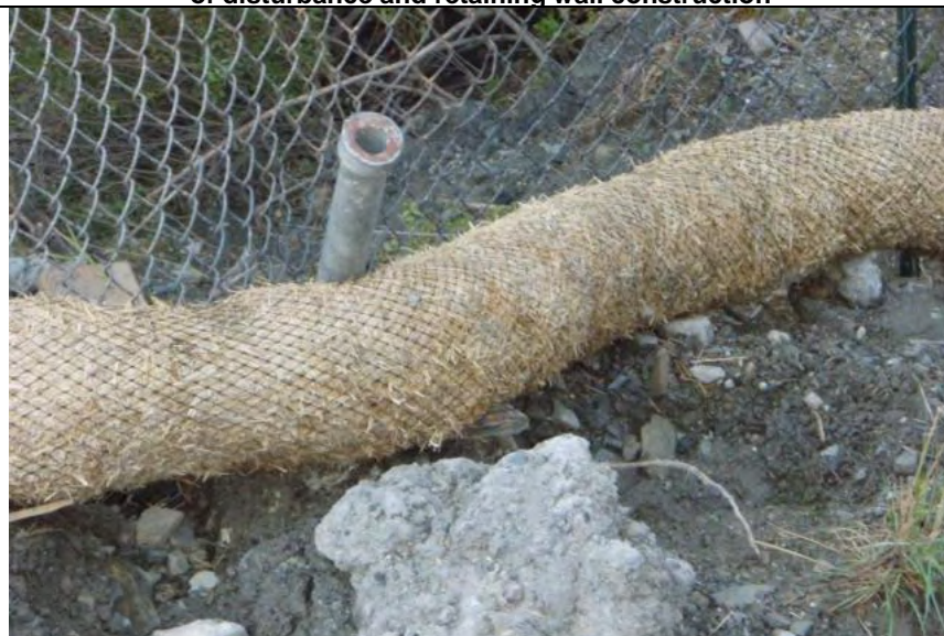
Photograph 4 – Close-up view of fiber roll not entrenched or staked into the ground
