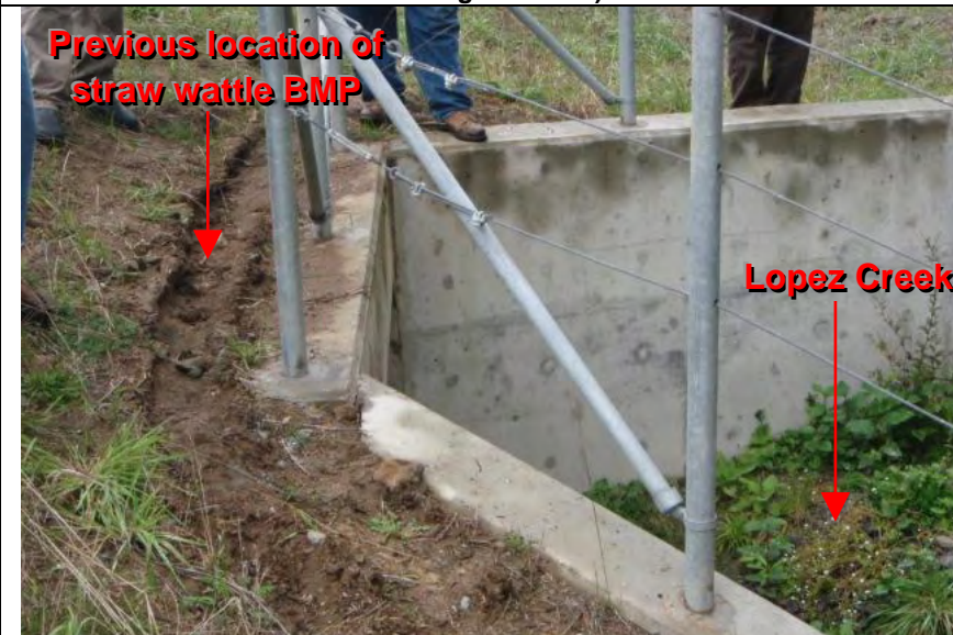
Photograph 8 – Area above culvert crossing of Lopez Creek
