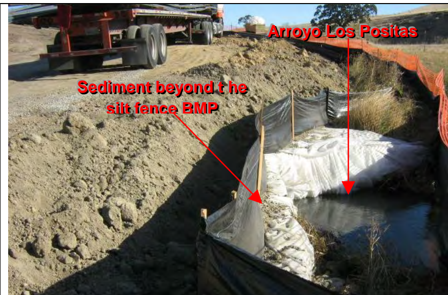
Photograph 1 – View of constructed Arroyo Los Positas diversion
