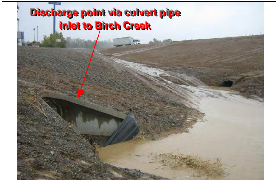
Photograph 9—Discharge point, culvert inlet and drainage pipe leading to Birch Creek
