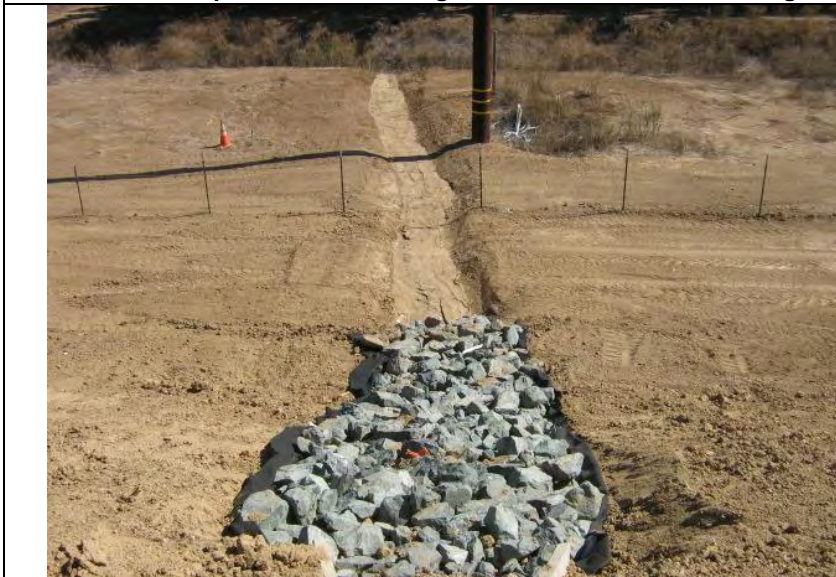
Photograph 27 – Slope drainage channel which drains to irrigation channel
