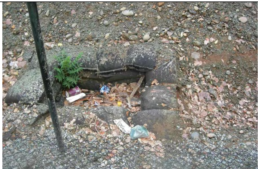
Photograph 8 – Storm drain inlet located along the bike path adjacent to Interstate 5
