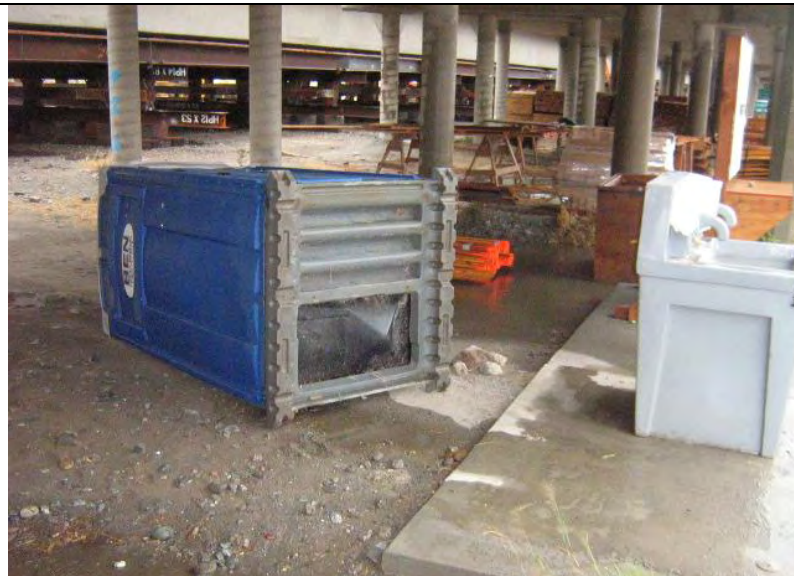
Photograph 12 – View of portable toilet blown over under Thomes Creek bridge
