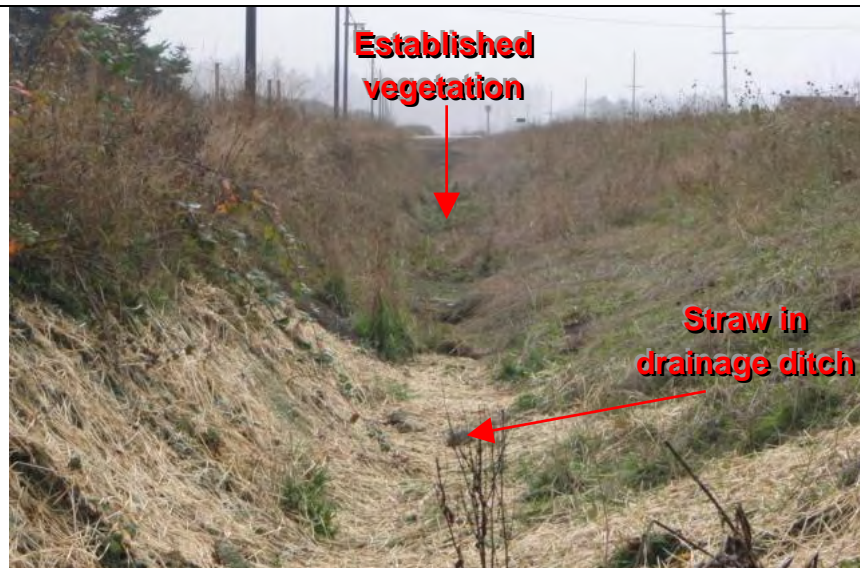
Photograph 4 – View of drainage ditch south of the culvert inlet
