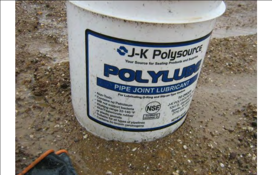
Photograph 8 – Close-up view of the full container of pipe joint compound in the eastern sediment basin
