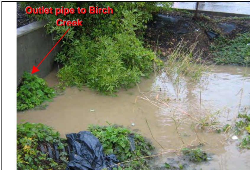
Photograph 13—Evidence of the discharge of sediment leading to Birch Creek
