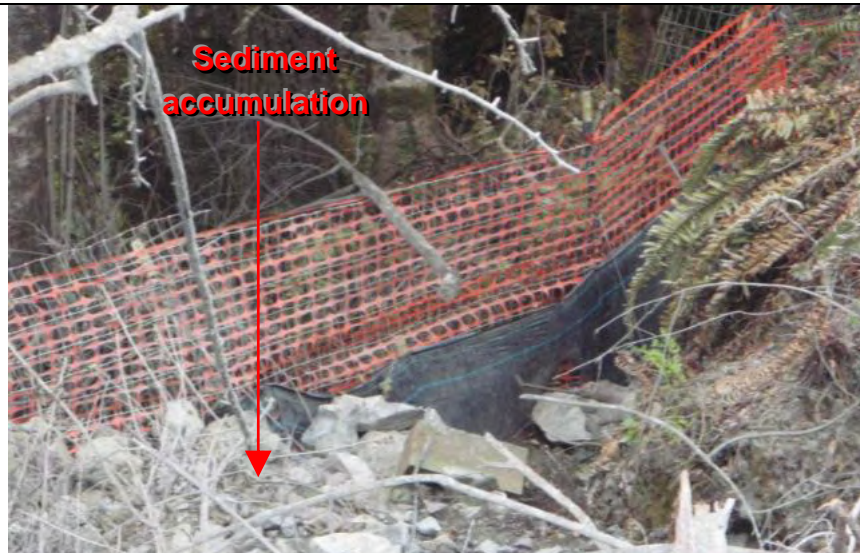
Photograph 3 – Example of sediment accumulation against silt fence BMP
