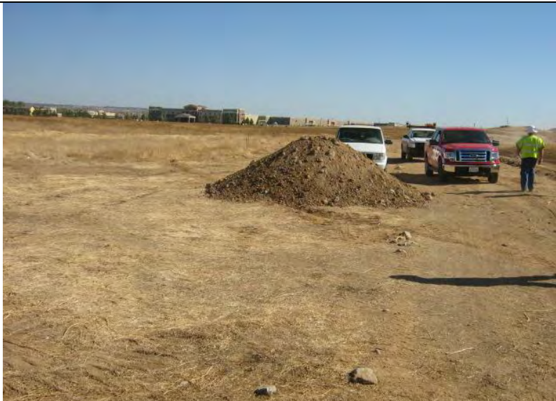
Photograph 9 – No BMPs implemented for stockpile management near the North Ingram Slough bridge crossing
