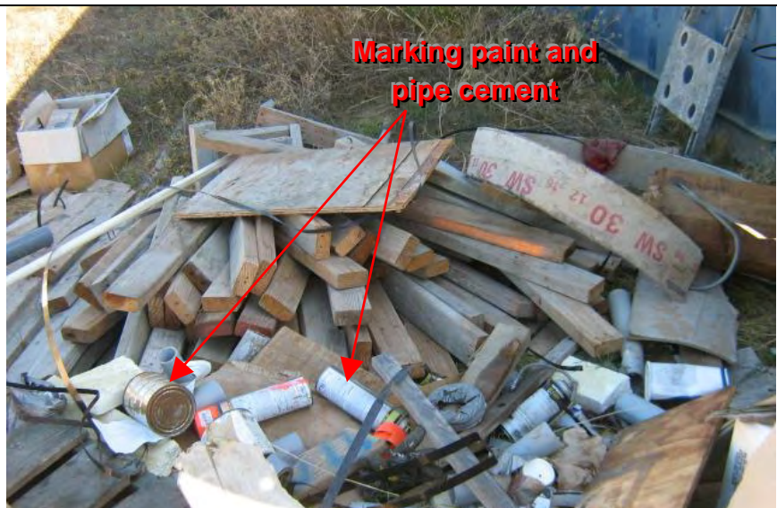
Photograph 3 – Construction wastes and chemicals improperly disposed
