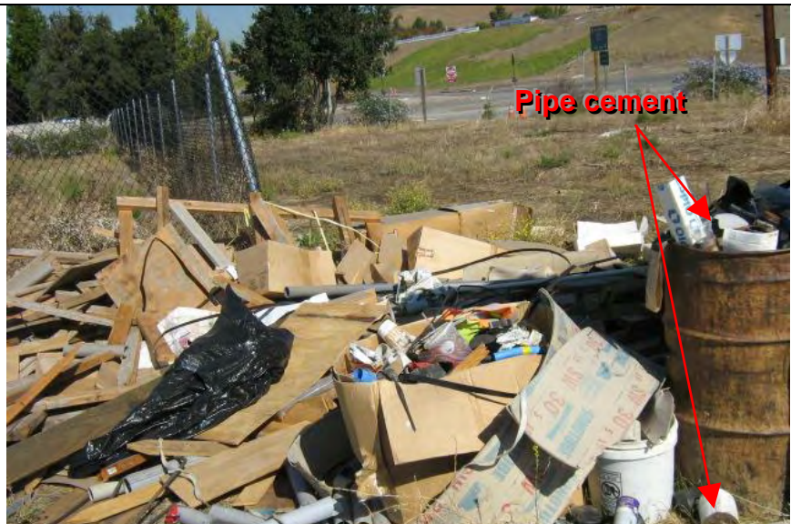
Photograph 1 – Construction wastes and chemicals improperly disposed
