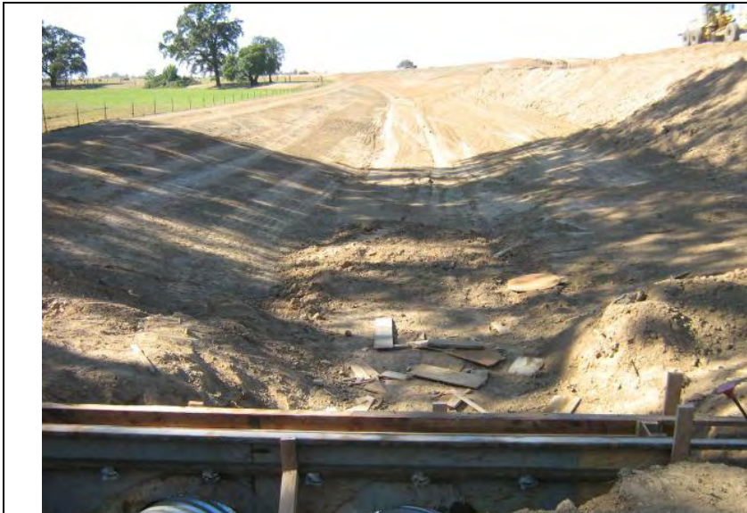
Photograph 17 – Upgradient areas of disturbance associated with pollution prevention BMP unstabilized. Drains to Auburn Ravine.
