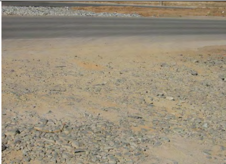
Photograph 6 – Close-up of Photograph 5 depicting sediment in VTC pad, and rock which was thin, sparse and compacted in areas
