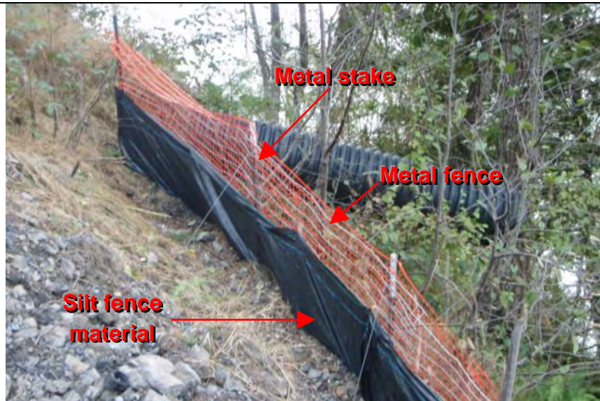
Photograph 1 – Example of reinforced silt fence BMP
