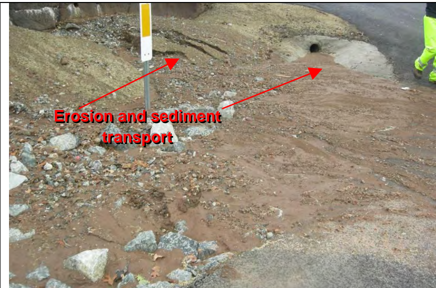
Photograph 5 – Lack of adequate BMPs to prevent discharge of sediment to the roadway
