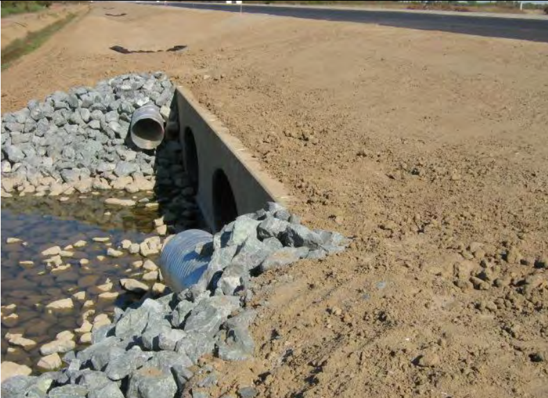
Photograph 13 – Adequate E&S controls were not implemented for areas of disturbance up-gradient of irrigation channel (East side)
