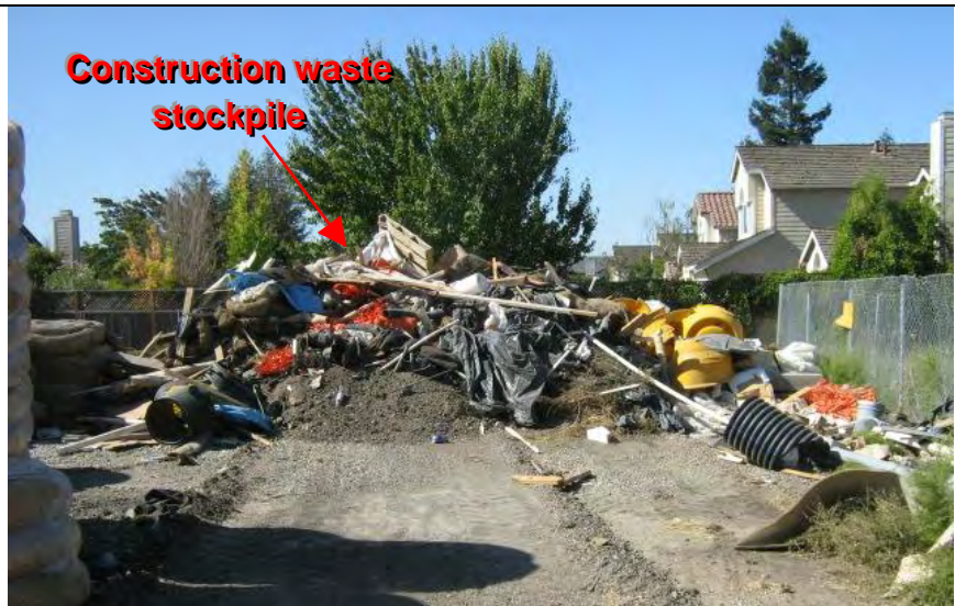
Photograph 5— Uncovered and uncontained construction waste
