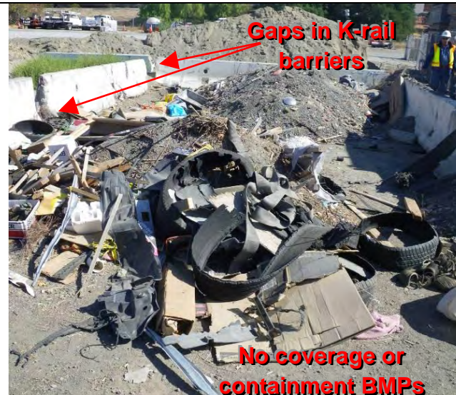
Photograph 10 – Sweeper and roadway waste stockpile
