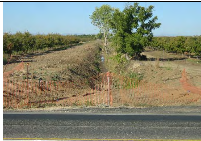
Photograph 10- View of down-gradient irrigation channel below outlet. Note: Inlet to this area is shown in Photograph 9.
