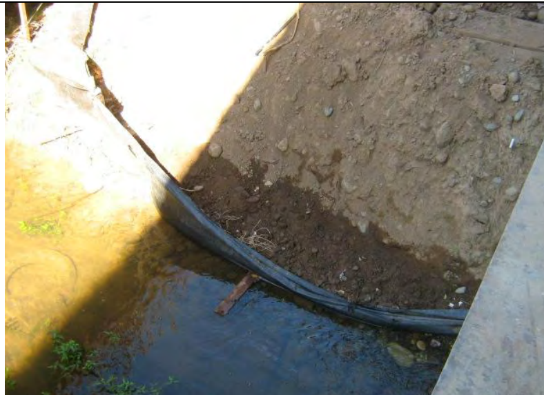
Photograph 22 – Close-up view of Photograph 21.
