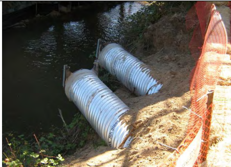
Photograph 18 – Disturbed slope area adjacent to pollution prevention BMP outlet pipes adjacent to Auburn Ravine.
