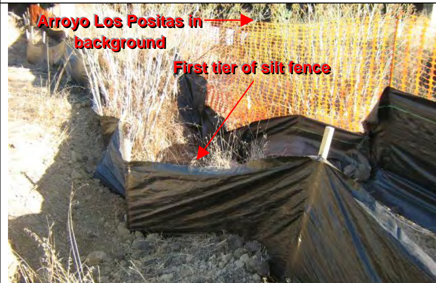
Photograph 4 – Silt fence BMP installed in a drainage depression
