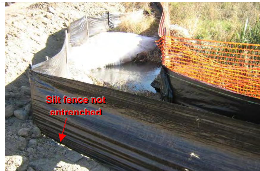
Photograph 2 – View of constructed Arroyo Los Positas diversion
