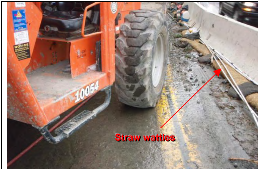
Photograph 17— View down-gradient from water container (Note: Wetness on impervious surface and placement of straw wattles)
