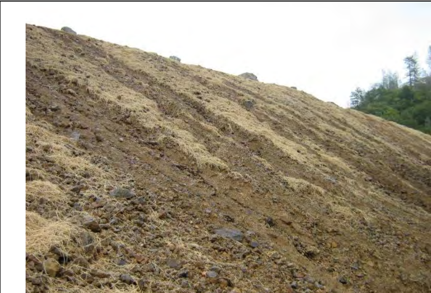
Photograph 1 – Evidence of erosion and slope failure on disturbed slope areas draining to Crystal Creek on the south side of State Highway 299
