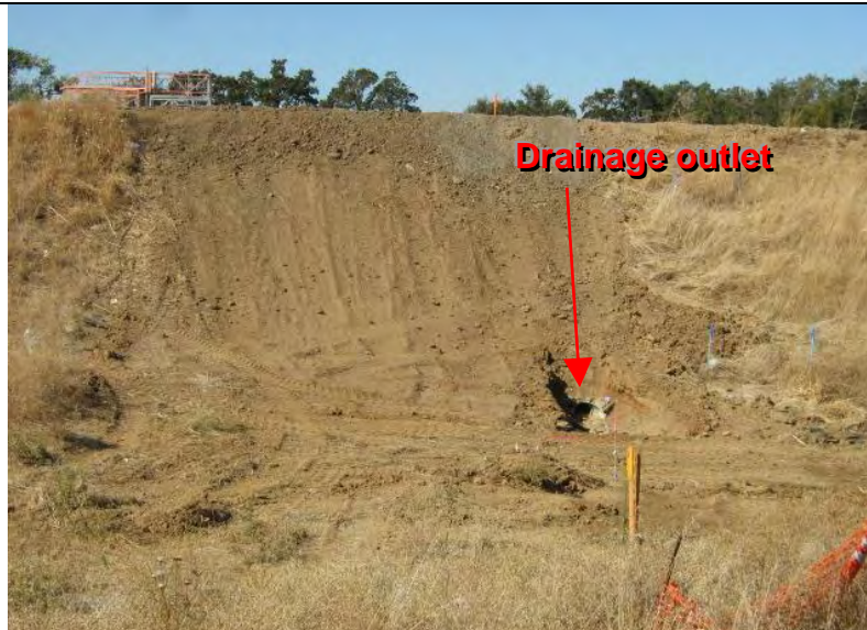
Photograph 6 – Drainage outlet below unstabilized embankment slope adjacent to the highway.
