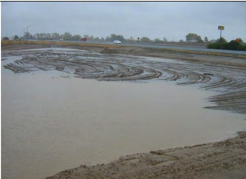
Photograph 1 – View of unstabilized sediment basin and embankment slopes
