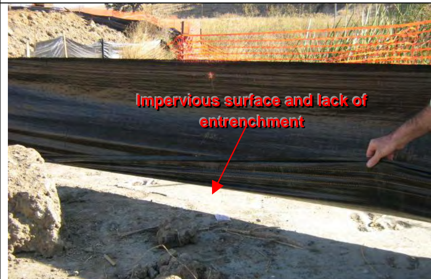
Photograph 3 – Close-up view of area shown in Photograph 2
