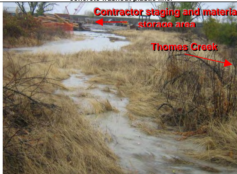
Photograph 4 – Evidence of the discharge of pollutants from the contractor staging and material storage areas
