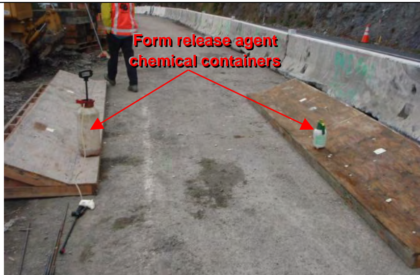
Photograph 10— Chemical sprayers not within secondary containment
