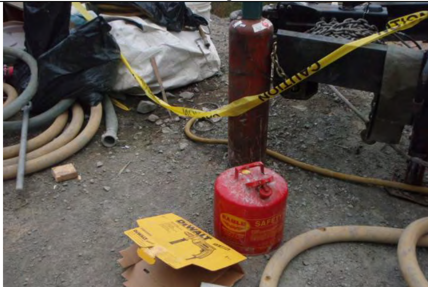
Photograph 11— Example of gas container not stored within secondary containment
