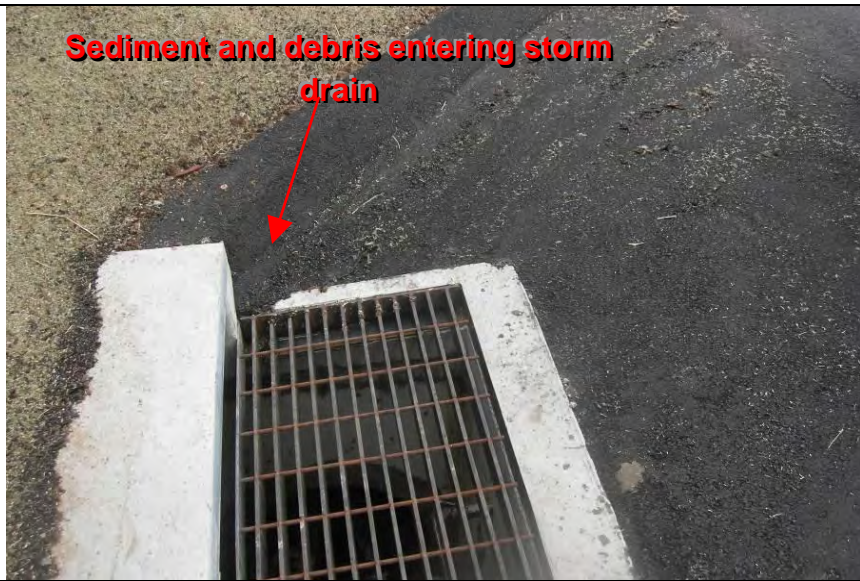
Photograph 4 – Storm drain located on the west side of Highway 299
