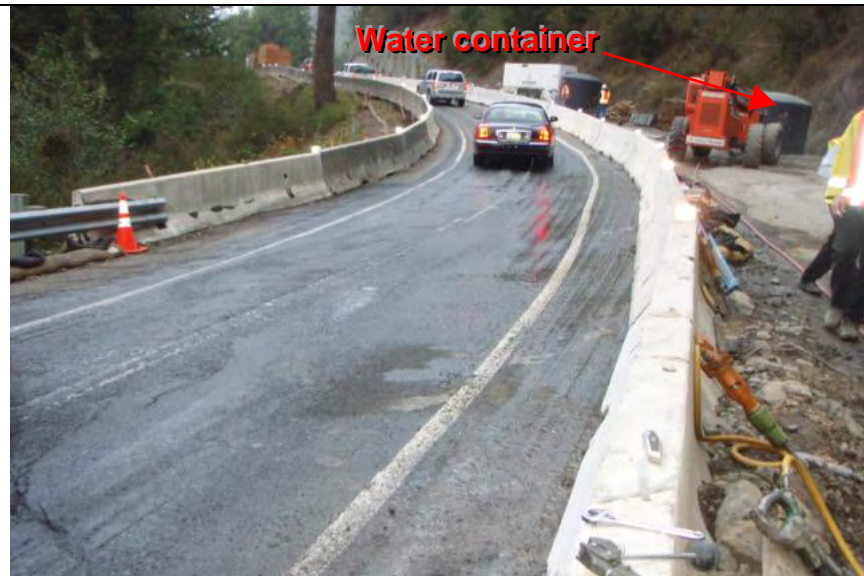
Photograph 18— View up-gradient to water container (Note: Wetness on roadway surface down-gradient of water container)
