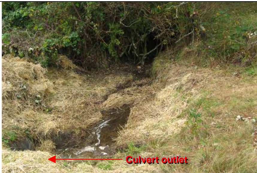
Photograph 7— Another view of the west side of culvert outlet
