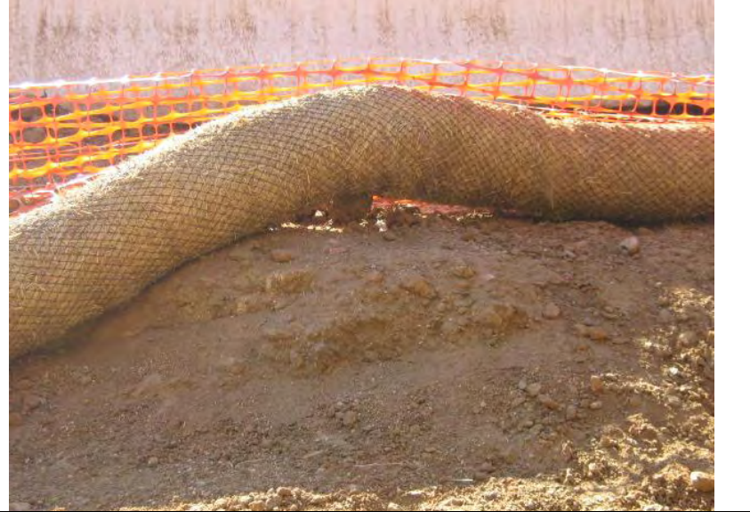
Photographs 16 – Straw wattle BMP not properly installed (e.g., not entrenched) up-gradient of Auburn Ravine
