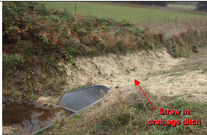
Photograph 5— View of drainage ditch south of the culvert inlet
