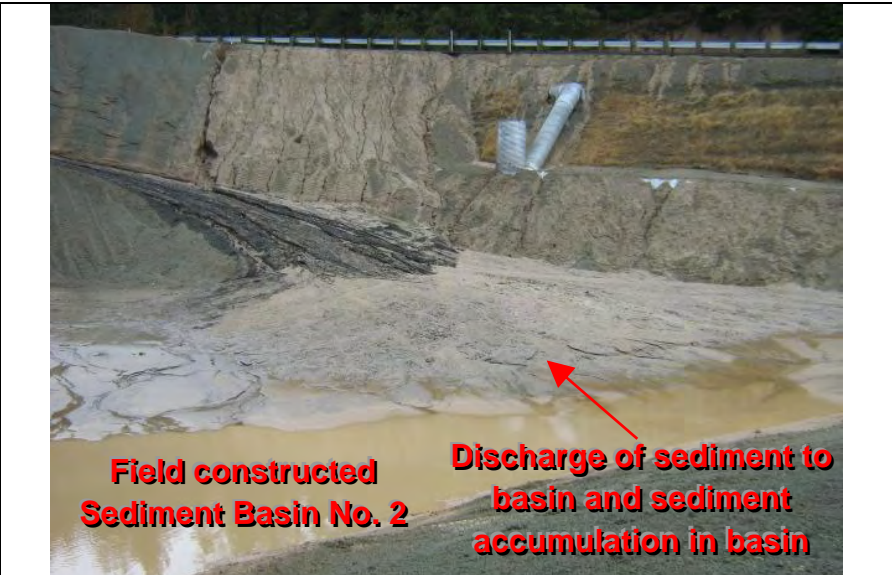
Photograph 2 – Discharge of sediment from disturbed slope area to field constructed sediment basin and sediment accumulation in the basin
