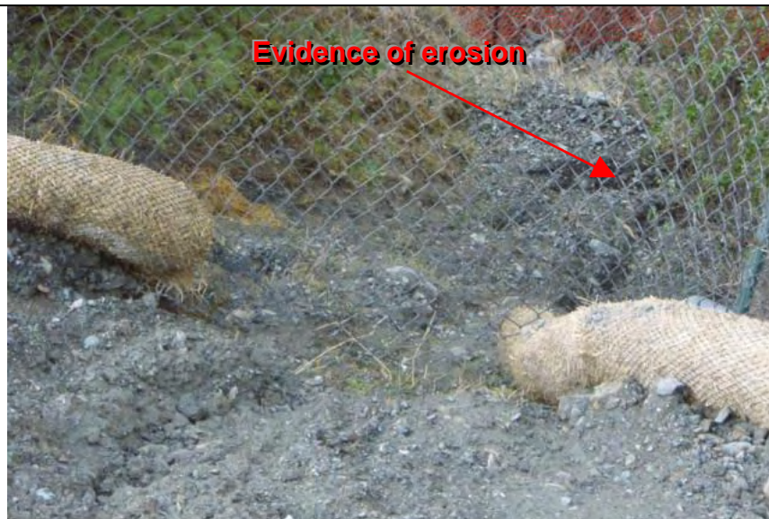
Photograph 8 – Closer view of straw wattle and erosion pictured in Photograph 7
