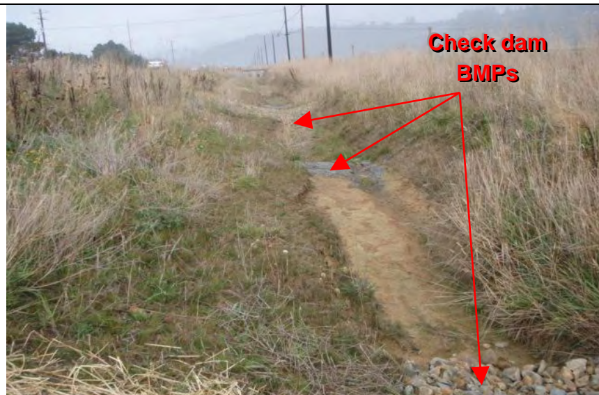
Photograph 3 – View up drainage channel
