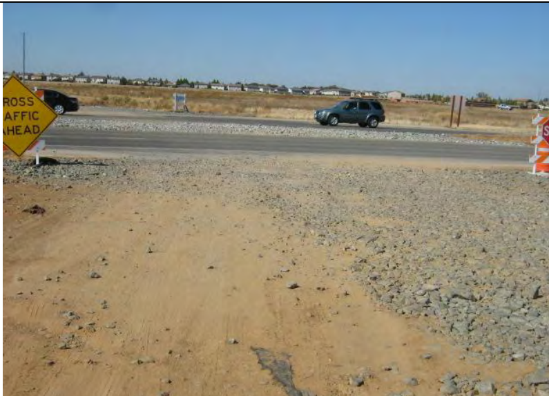
Photograph 5 – Vehicle tracking pad BMP not adequately maintained (e.g., sediment in pad, and rock thin and sparse in areas)
