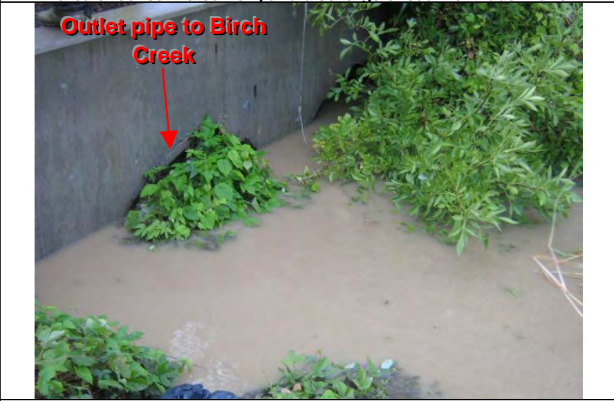
Photograph 12 – View of outlet pipe from Photograph 11 leading to Birch Creek
