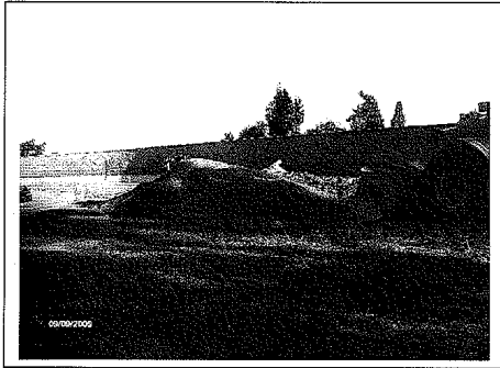
13. AC grindings should be either covered or perimeter control prior to rain.
