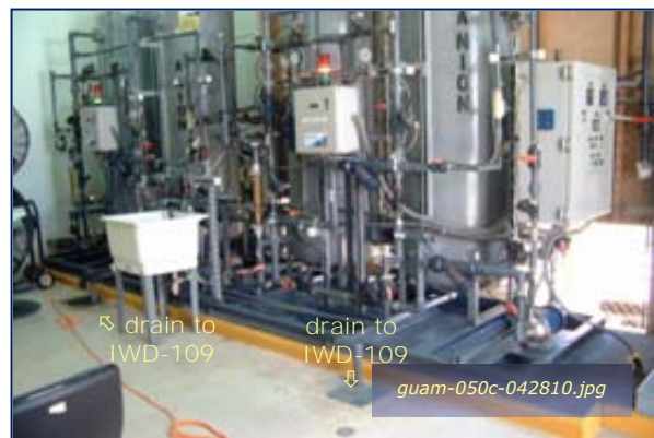
Photo #4-28: Bldg 4907 Demin Plant - IX Unit Taken By: Greg V. Arthur Date: 04/28/10
