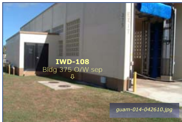
Photo #4-23: Bldg 375 Outdoor Washrack - O/W Sep Taken By: Greg V. Arthur Date: 04/26/10
