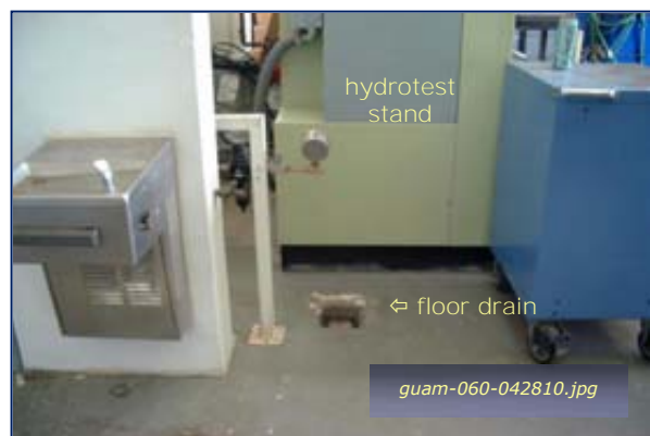
Photo #4-34: Bldg 4430 Shore Repair Facility Taken By: Greg V. Arthur Date: 04/28/10
