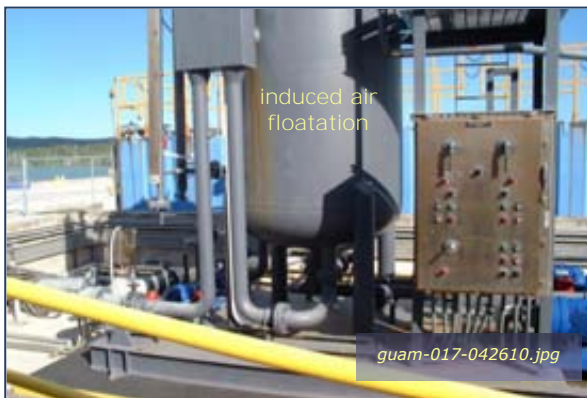
Photo #4-5: Victor Wharf BOWTS – IAF Unit Taken By: Greg V. Arthur Date: 04/26/10
