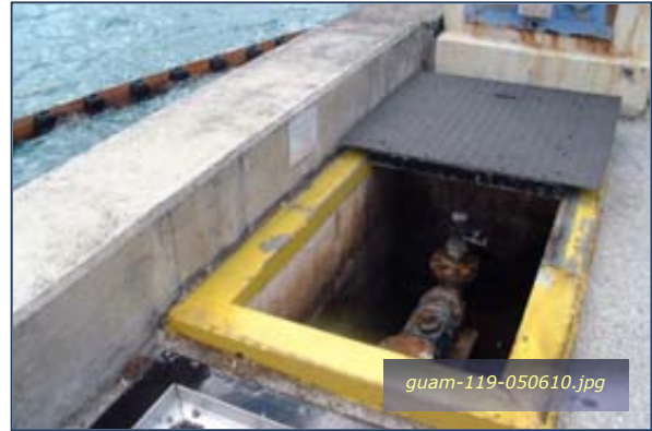
Photo #4-2: Bilge Pump Station Riser at Victor Wharf Taken By: Greg V. Arthur Date: 05/06/10
