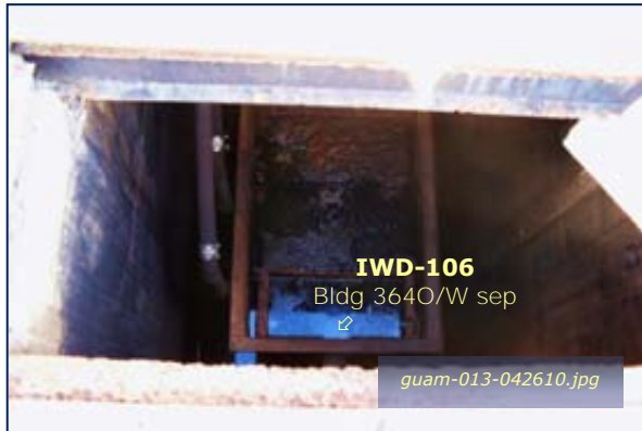
Photo #4-19: Bldg 364 Motor Pool - O/W Sep Vault Taken By: Greg V. Arthur Date: 04/26/10
