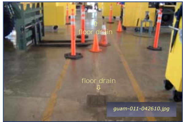
Photo #4-20: Bldg 364 Motor Pool - Floor Drains Taken By: Greg V. Arthur Date: 04/26/10
