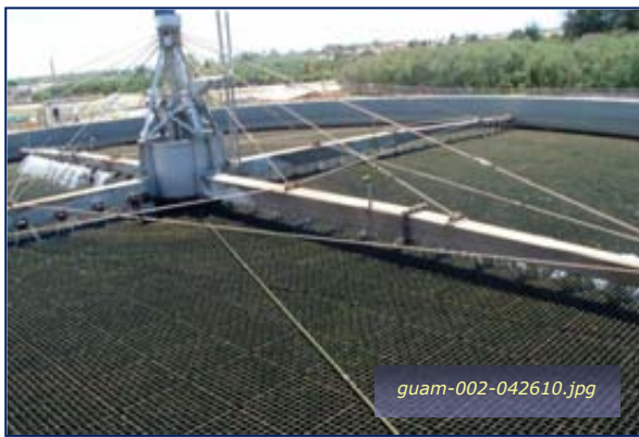
Photo #3-1: Top View - Biotower Trickling Filter Taken By: Greg V. Arthur Date: 04/26/10
