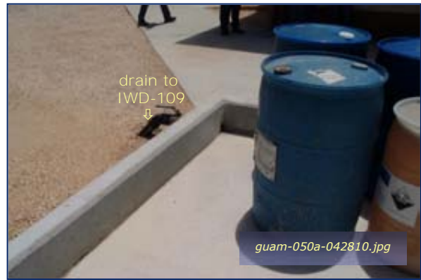
Photo #4-26: Bldg 4907 Demin Plant - Rack Drain Taken By: Greg V. Arthur Date: 04/28/10
