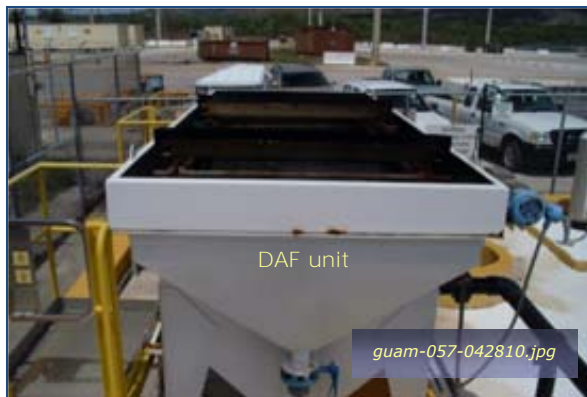
Photo #4-9: Polaris Point BOWTS - DAF Unit Taken By: Greg V. Arthur Date: 04/28/10
