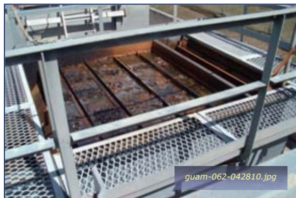
Photo #4-12: FISC Fuel Farm - O/W Plate Coalesce Taken By: Greg V. Arthur Date: 04/28/10
