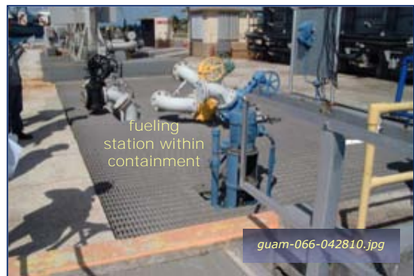
Photo #4-16: FISC Fueling Pier – Containment Drain Taken By: Greg V. Arthur Date: 04/28/10
