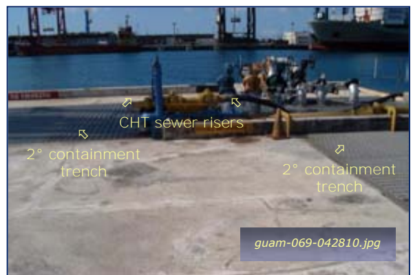
Photo #3-10: Echo Fueling Pier CHT Sewer Riser Taken By: Greg V. Arthur Date: 04/28/10
