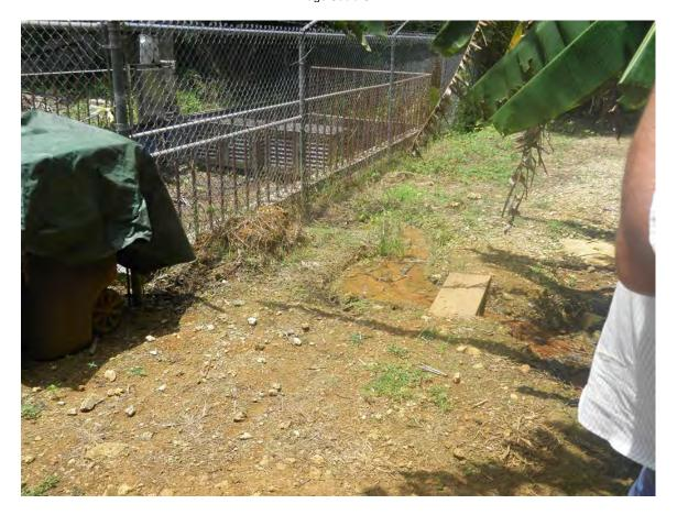
Picture 6: Water from a leaking potable water line was running in a shallow ditch into the plant. Ditch was bridged by the board in the middle right.
