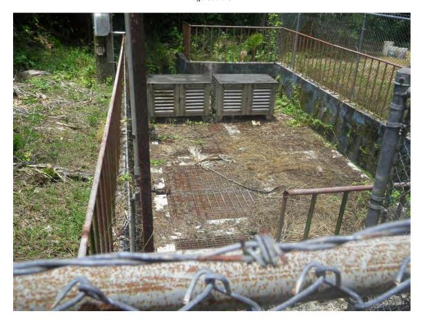
Picture 4: Blower housing for aeration system. Blowers were not operating.
