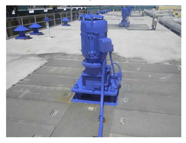
Picture 13: Digester aerator motor.
