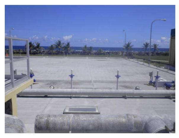
Picture 10: Concrete roof over primary clarifiers.
