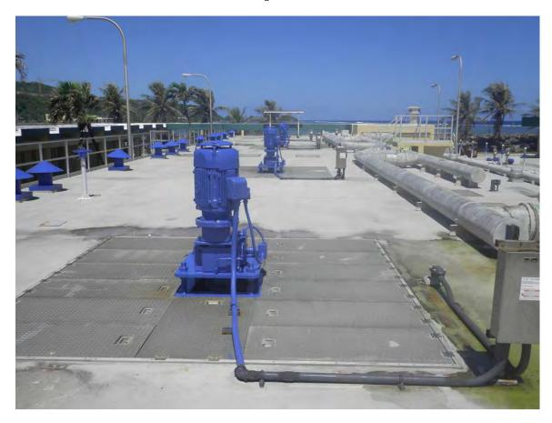
Picture 12: Drive motors for aerated digesters.
