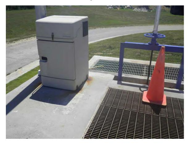
Picture 19: Effluent automatic sampler.
