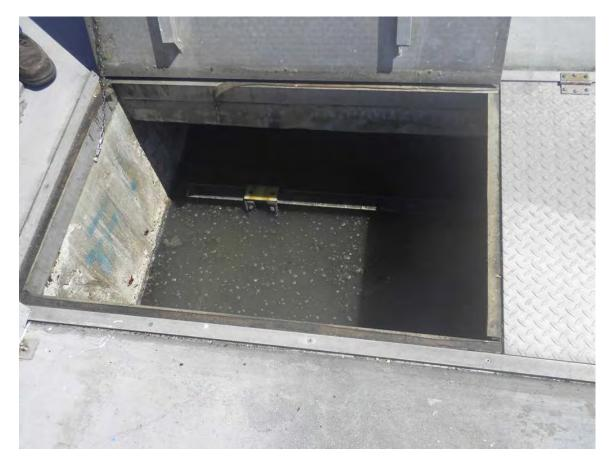
Picture 9: Flight in primary clarifier through access hatch.
