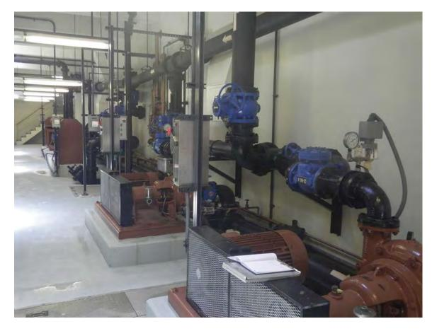
Picture 25: Sludge pumps for primary clarifiers.
