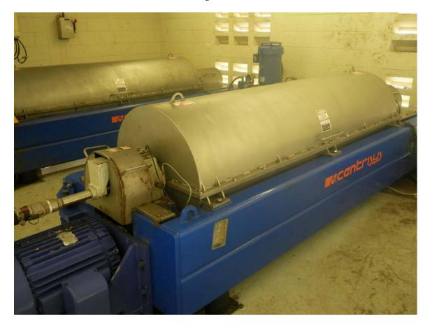
Picture 21: Dewatering centrifuges.
