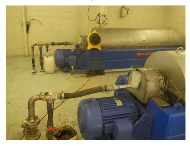
Picture 22: Feed lines for centrifuges.
