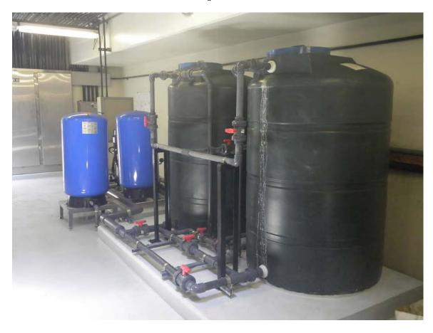
Picture 24: Dewatering polymer feed tanks.
