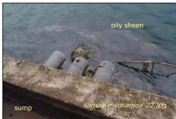
Photo #12: Catch Basin #1 - Oily Sheen in Harbor Taken By: Greg V. Arthur Date: 04/01/08
