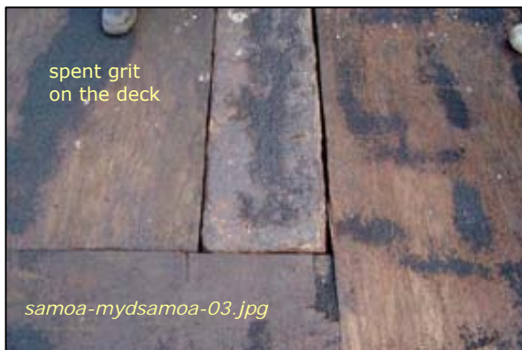
Photo #3: 3000-Ton Dry Dock - Gaps Between Boards Taken By: Greg V. Arthur Date: 04/01/08
