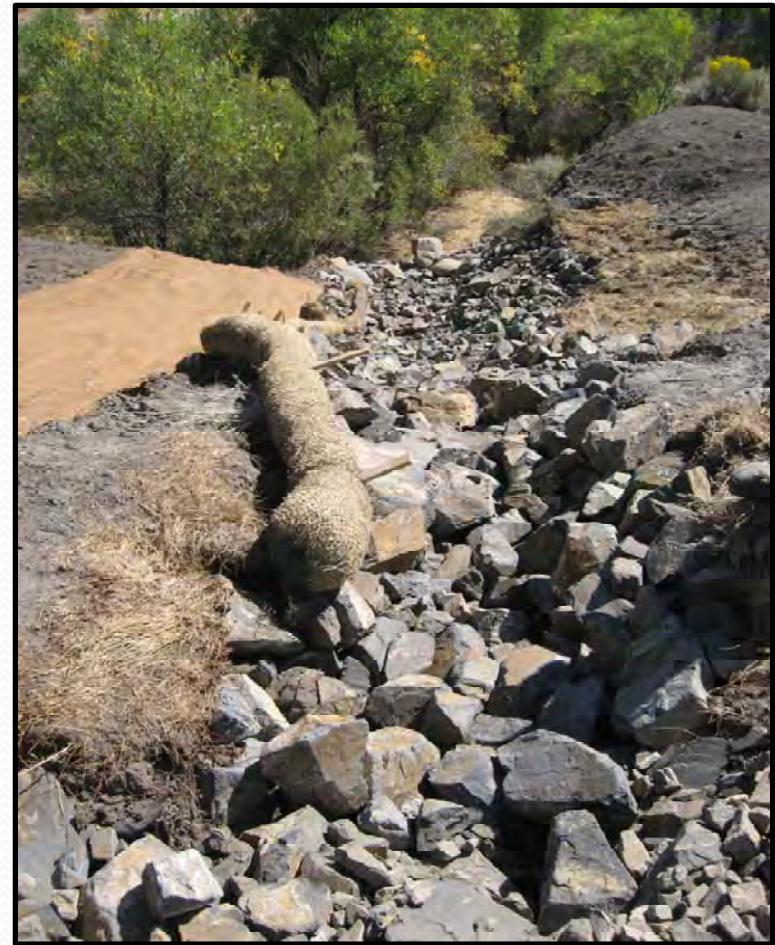
Washoe Tribe of NV & CA to decrease runoff and sedimentation
