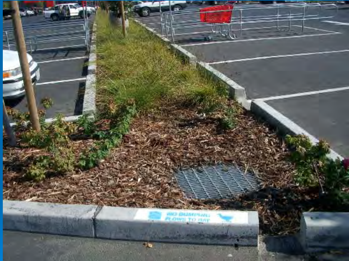
Parking lot treatment- vegetative buffer strip
