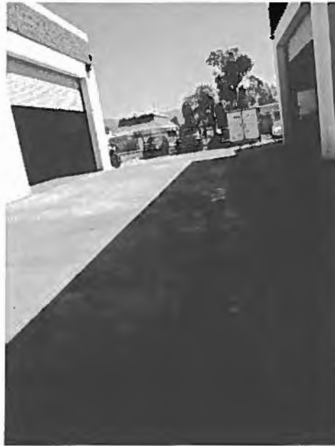
Photograph 1. Bill's Quality Auto Care – View of the impervious area located on the east side of the facility garage.
