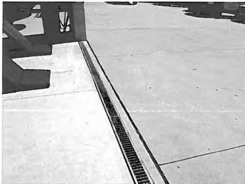
Photograph 2. Bill's Quality Auto Care – View of a trench grate located indoors adjacent to the impervious outdoors facility area.
