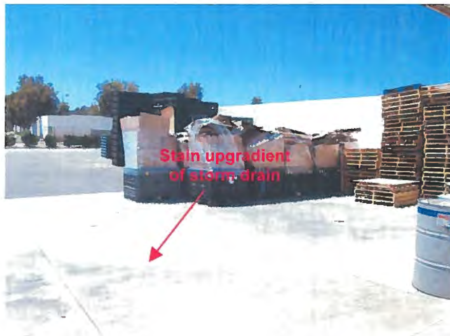
Photograph 2. PTI Facility I/C Site Visit – Additional view of the paved yard located on the west side of the building. Note the additional view of the stain shown in Photograph 1.
