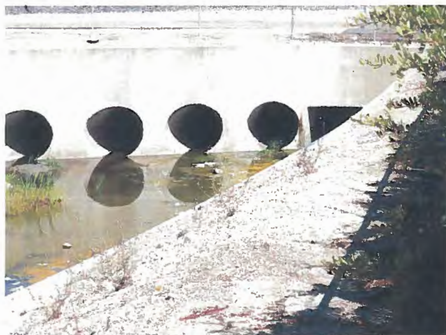
Photograph 2. City MS4 Outfall – El Rio Drain Outfall – Close-up view of the outfall from the City MS4 to the VCWPD.
