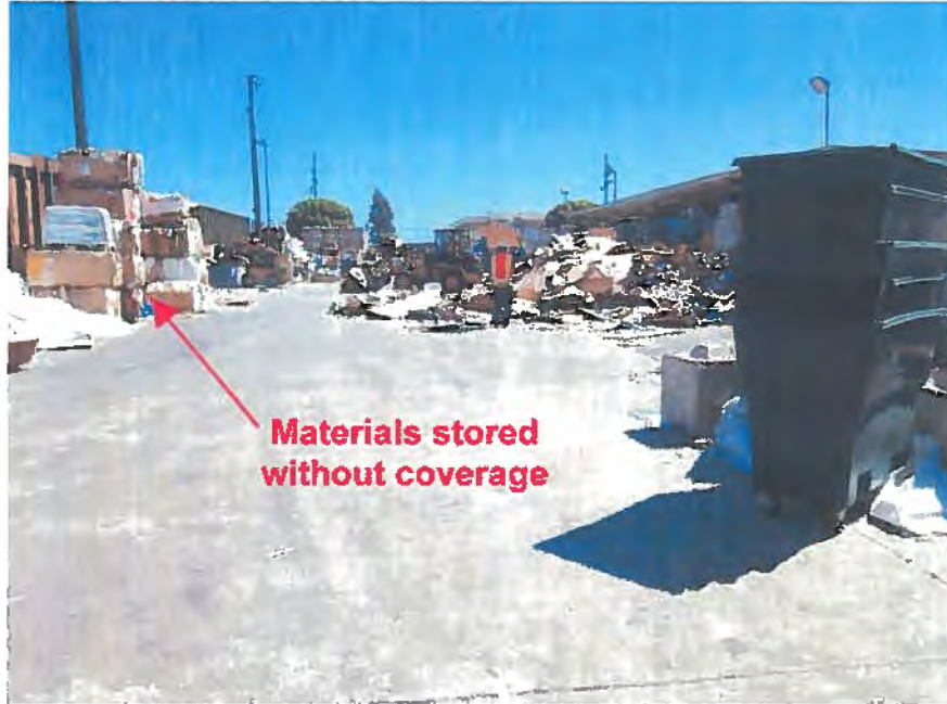
Photograph 1. Rincon Facility I/C Site Visit – View looking south of materials stored at the facility without coverage.
