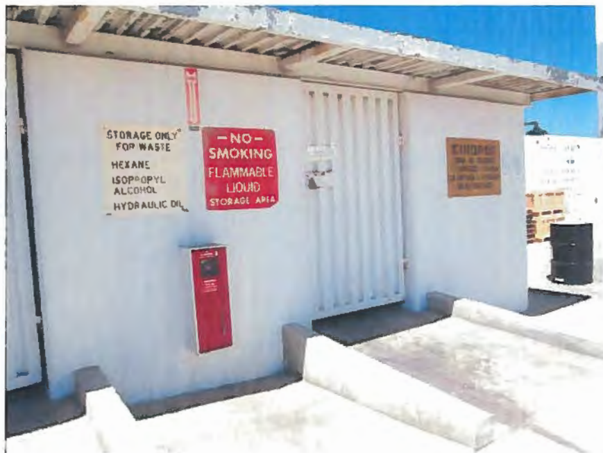
Photograph 3. PTI Facility I/C Site Visit – View of hazardous materials shed located on the northern side of the paved yard.
