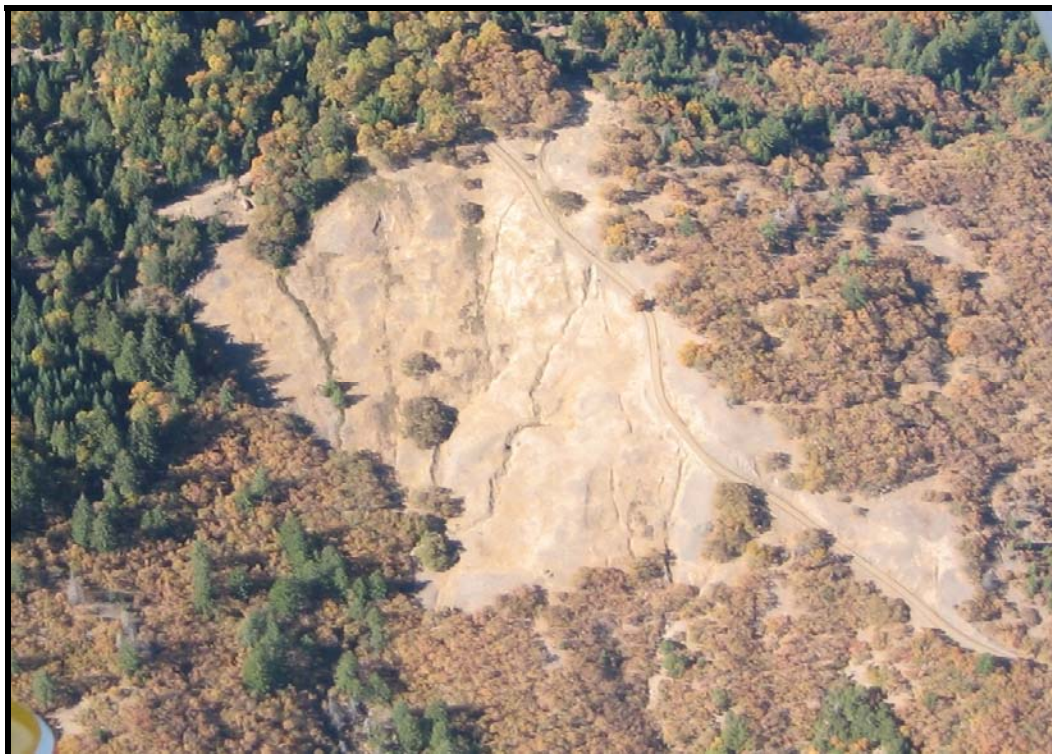
Photograph 4. Active earthflow looking obliquely to the south west. Earthflow is enlarging as a result of road drainage.
