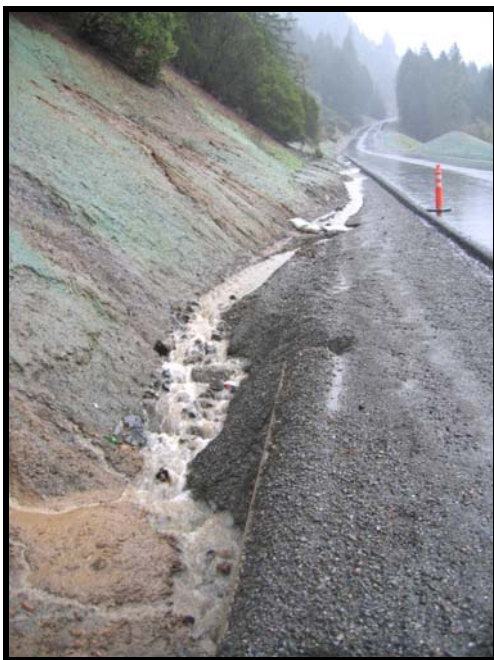
Photograph 1. Lower Mad Road (insloped and paved) looking east during December 2005 flood event. Surface erosion from road cutslope actively eroding and delivering sediment to a cross-drain and the Mad River. Measured unit sediment load ranged from 361 to 6,925 tons/mi 2 /year.
