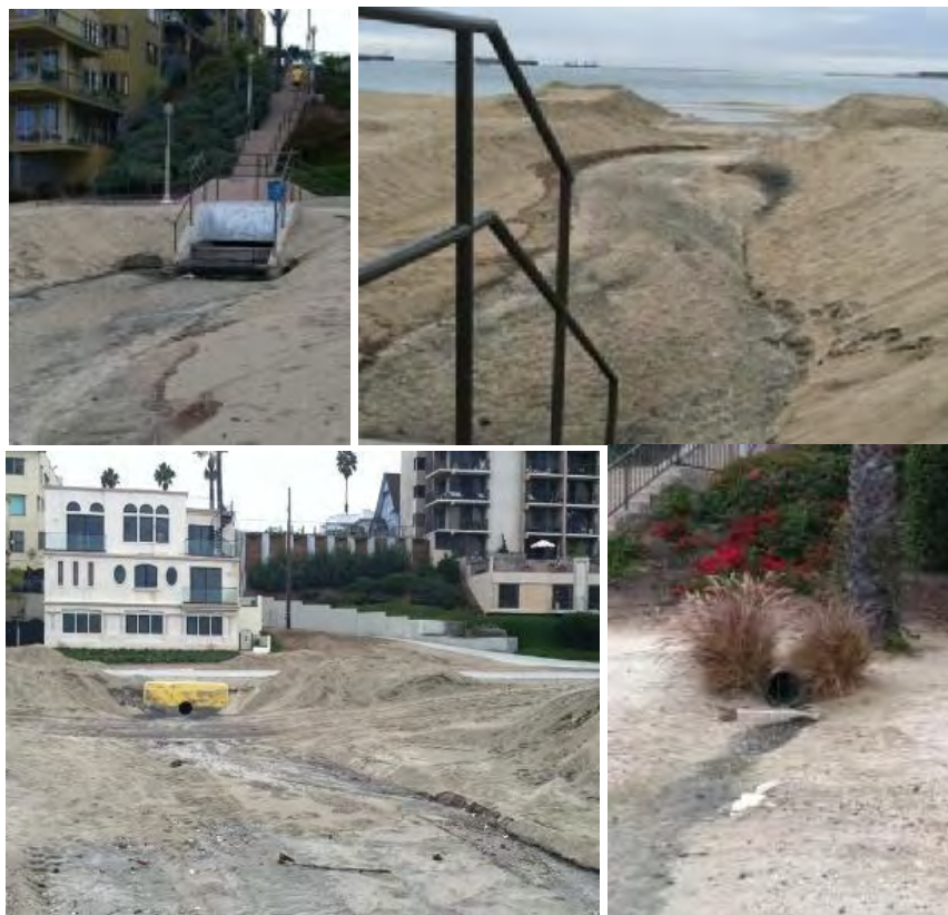
Figure 5-5. Images of storm drains between South 5 th Place and South 16 th Place on Long Beach City Beaches from November 13, 2011
