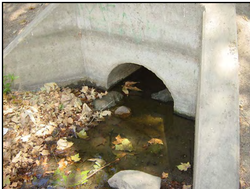
Figure 10-8. Storm Drain Discharge to a Small Depression (that Subsequently Flows to Puddingstone Reservoir)
