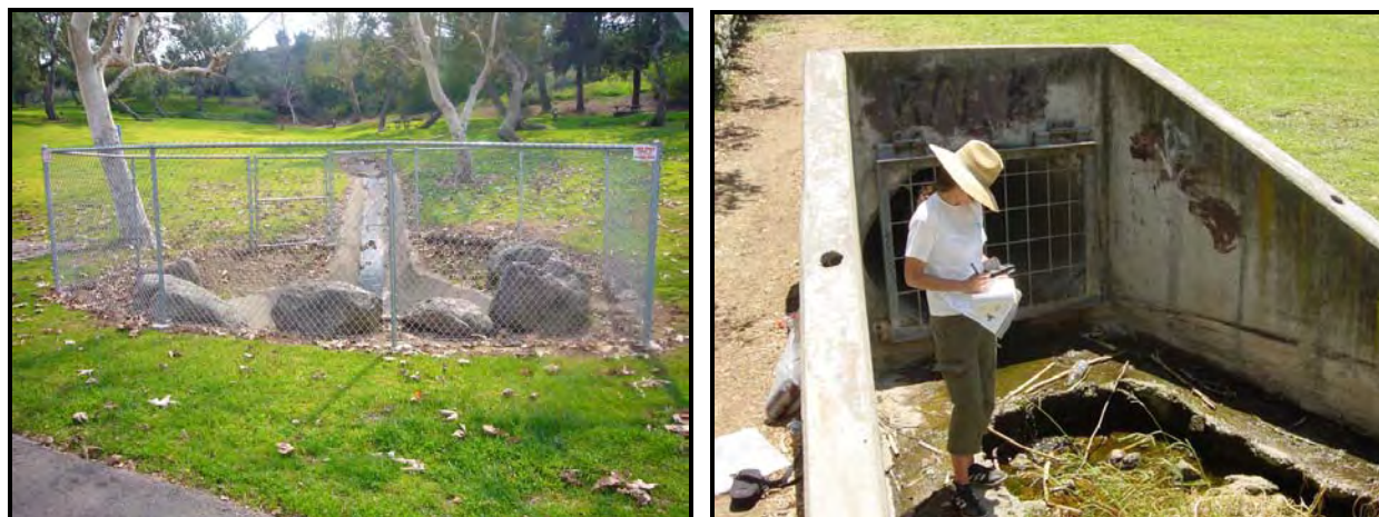
Figure 10-6. Storm Drain Discharges to Puddingstone Reservoir
