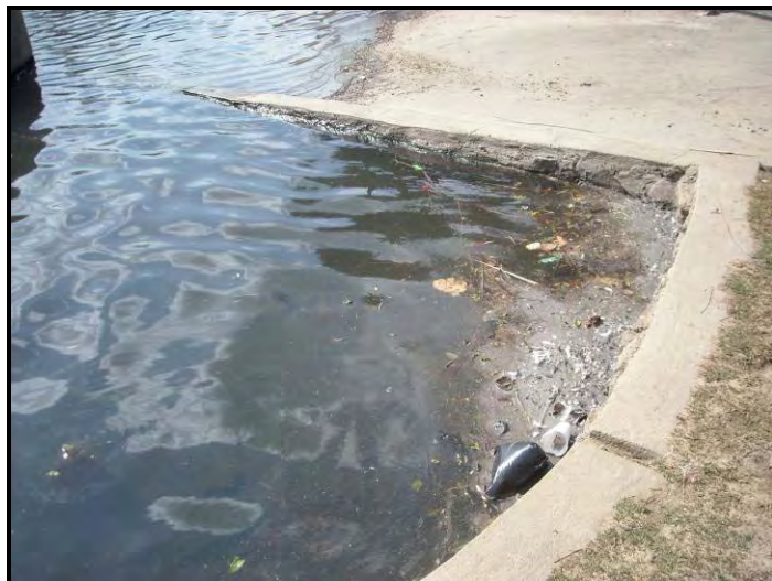
Figure 5-9. Scum and Trash Accumulate in the Sharp Corners of Lincoln Park Lake
