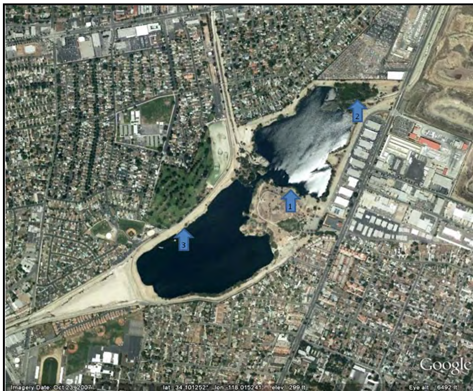
Figure 4-14. Quantitative Monitoring Locations at Peck Road Park Lake
