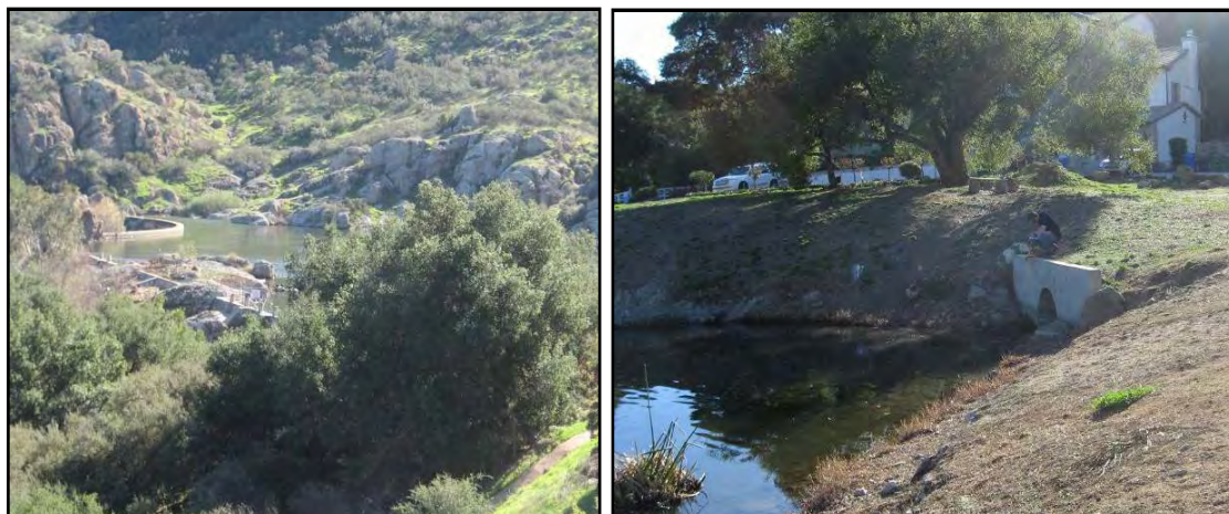
Figure 12-2. Lake Sherwood Dam and One of Several Storm Drains
