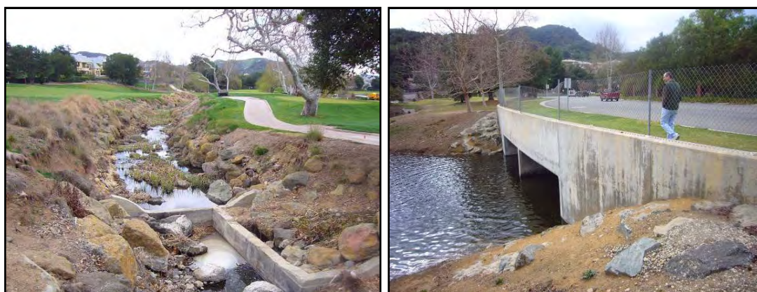
Figure 12-3. Creek Winding Through Golf Course and Discharging to Lake through Culverts
