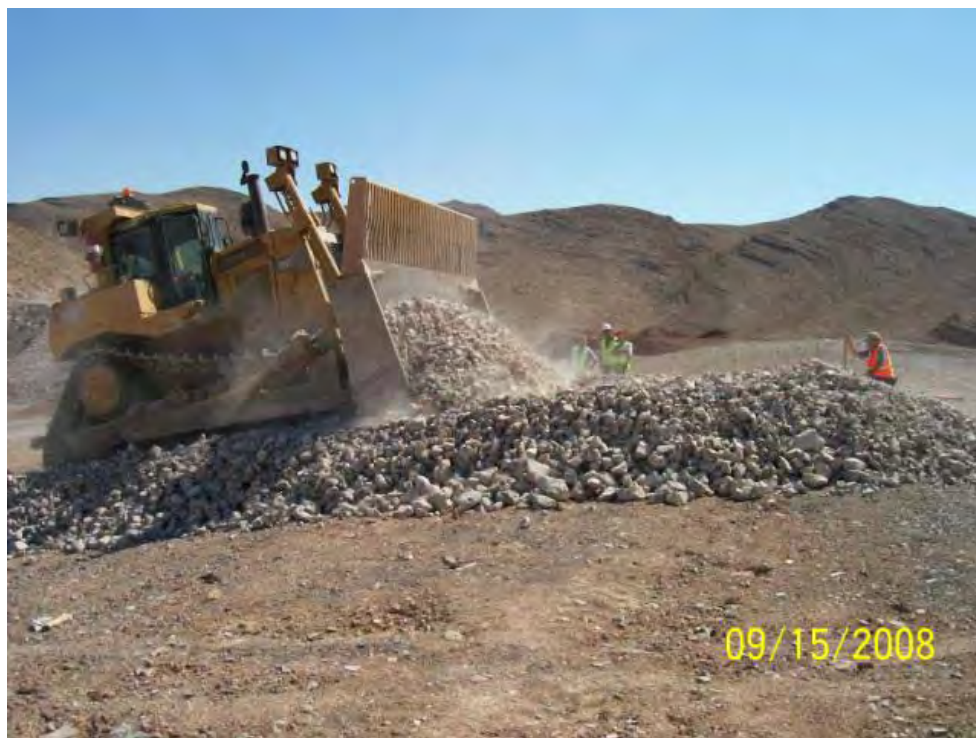
Photo 3 Spreading Erosion Layer Material to 18" thickness
