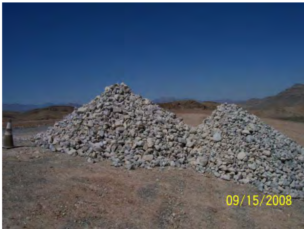
Photo 1 Erosion Layer Material Prior to Placement
