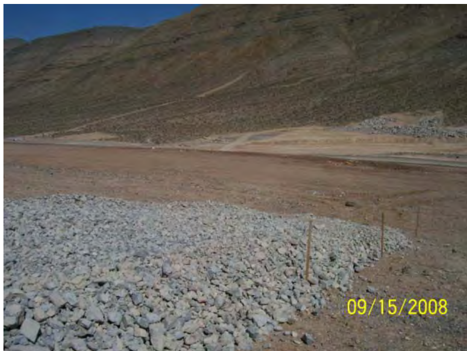
Photo 7 Finished Test Pad 18" Compacted Thickness
