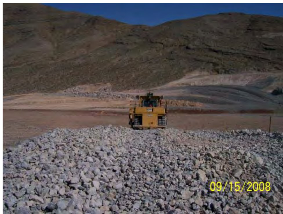
Photo 4 Compacting with Tracked Bulldozer
