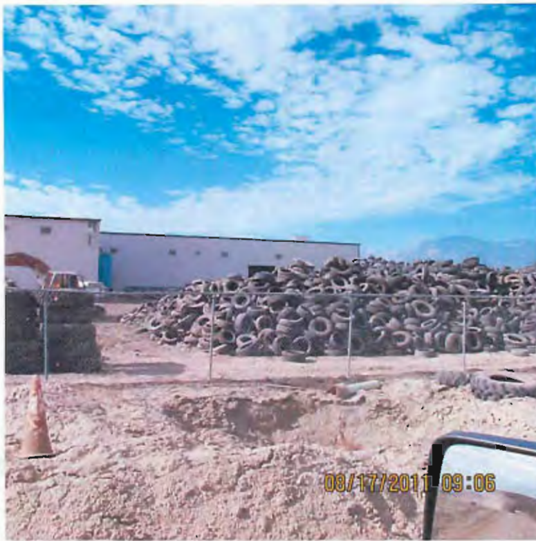
A view of the aisle with the tire handling equipment from outside the facility. The current survey photo is very similar. The tires outside of the fence, visible on the right, were placed to form a barrier for a hole that was excavated to repair piping.
