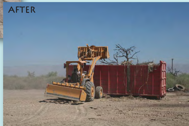
Martinez Road, before and after cleanup.
