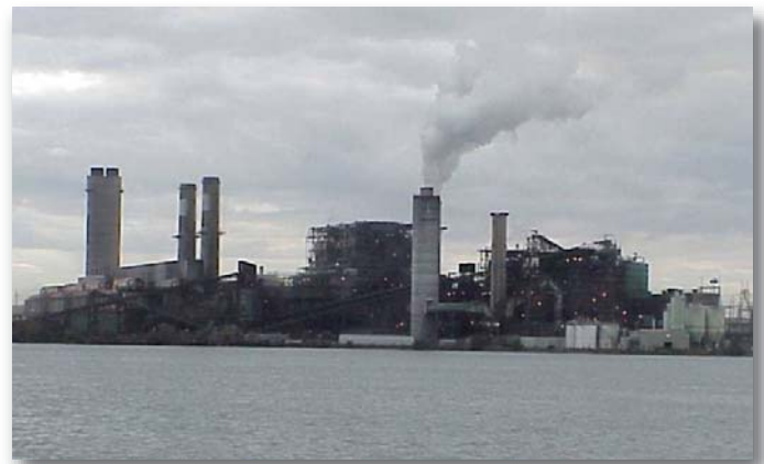
Navajo Nation - Four Corners Power Plant.
