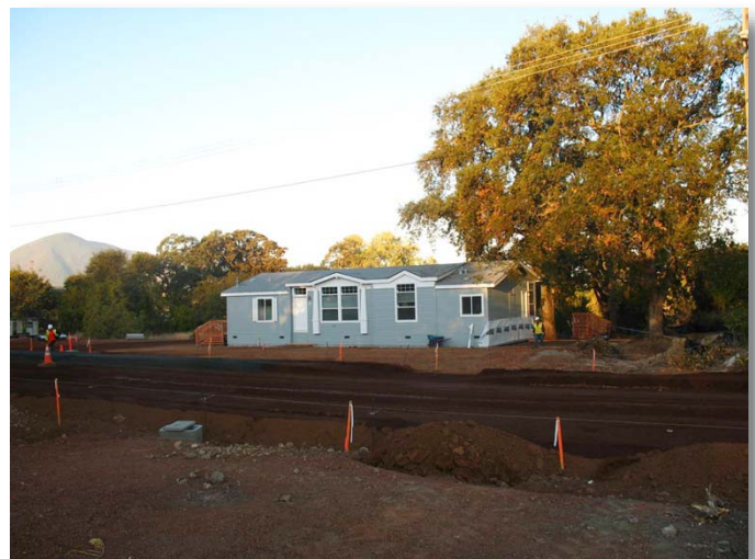
Elem Indian Colony of Pomo Indians of the Sulfur Bank Rancheria - new modular home installation.
