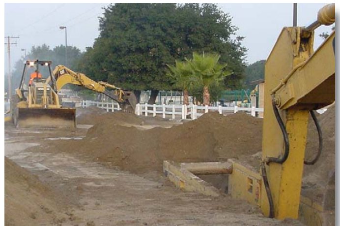
Pechanga Band of Luiseno Mission Indians of the Pechanga Reservation - trunk sewer construction.
