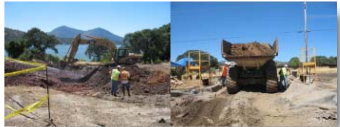
Elem Indian Colony of Pomo Indians of the Sulfur Bank Rancheria - mercury and arsenic removal (left) and vehicle cleaning pad (right).
