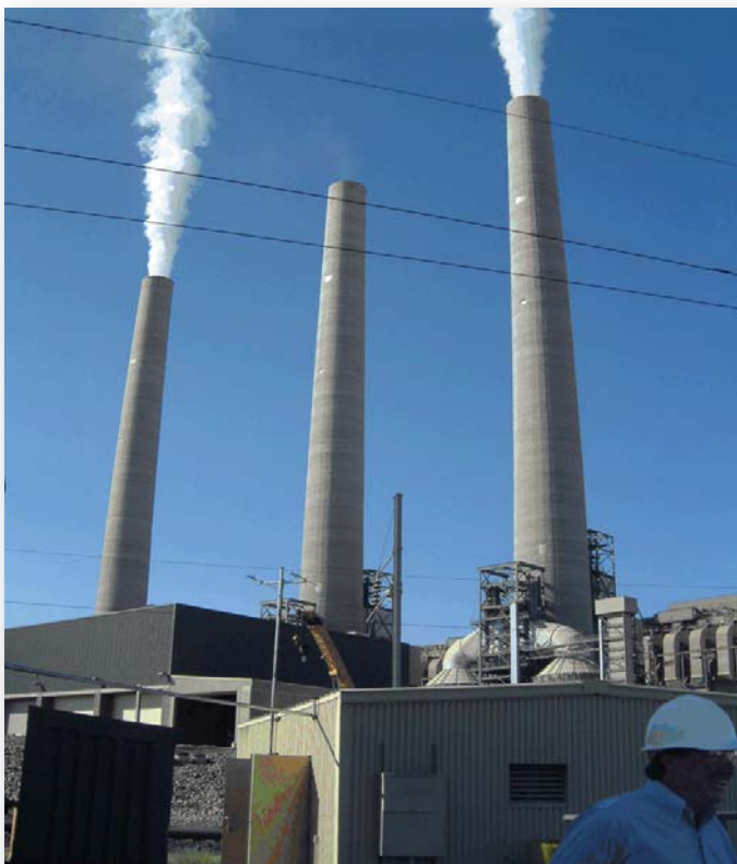
Navajo Nation - Power Generating Plant.
