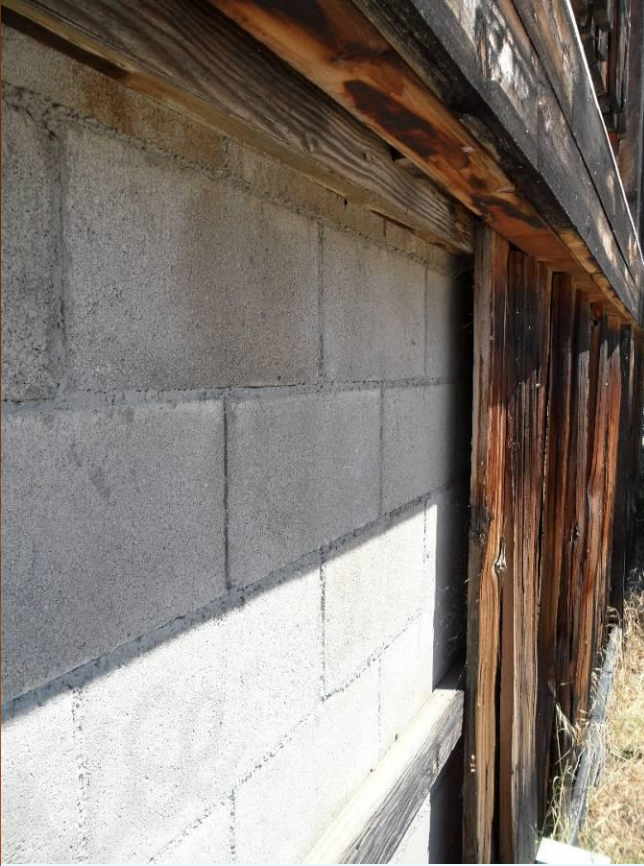
Filled concrete blocks and furring strips
