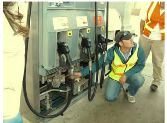
William Berquist, Inspector with the Washoe Tribe of Nevada and California, conducting a field training session and checking for leaks under the fuel dispensers at a gas station.
