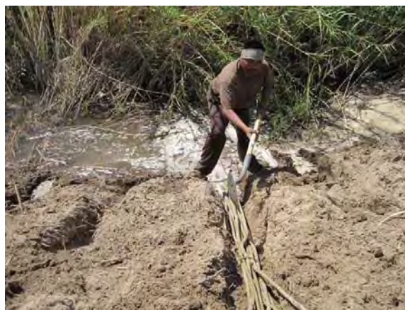
Reggie Antone, Quechan Indian Tribe Environmental Department employee and tribal member, planting bundles of sandbar (coyote) willow poles for bank stabilization along the Colorado River.
