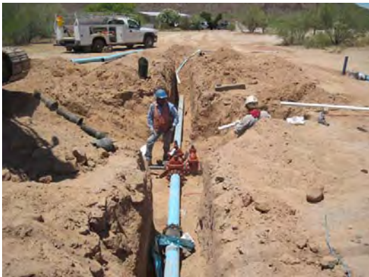
Workers James Johnson and Gary Wilson, Jr. install a valve to connect the Gunsight community wells to the upgraded water distribution system.
