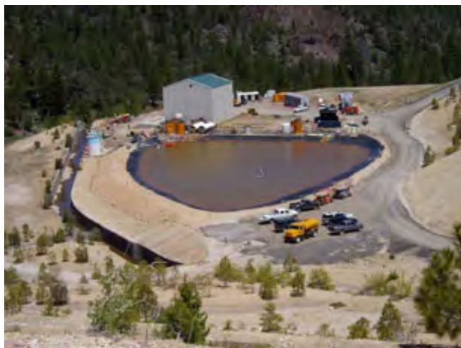
Washoe Tribe of California and Nevada, lime treatment system for acid mine drainage at Leviathan Mine, Nevada.
