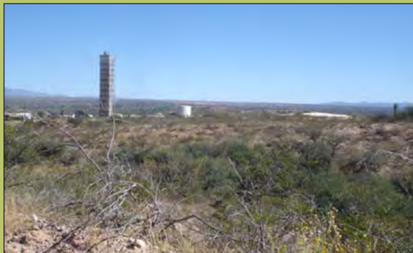
PICTURED: Apache Nitrogen Products buildings at Apache Powder Superfund site. (source: EPA)
