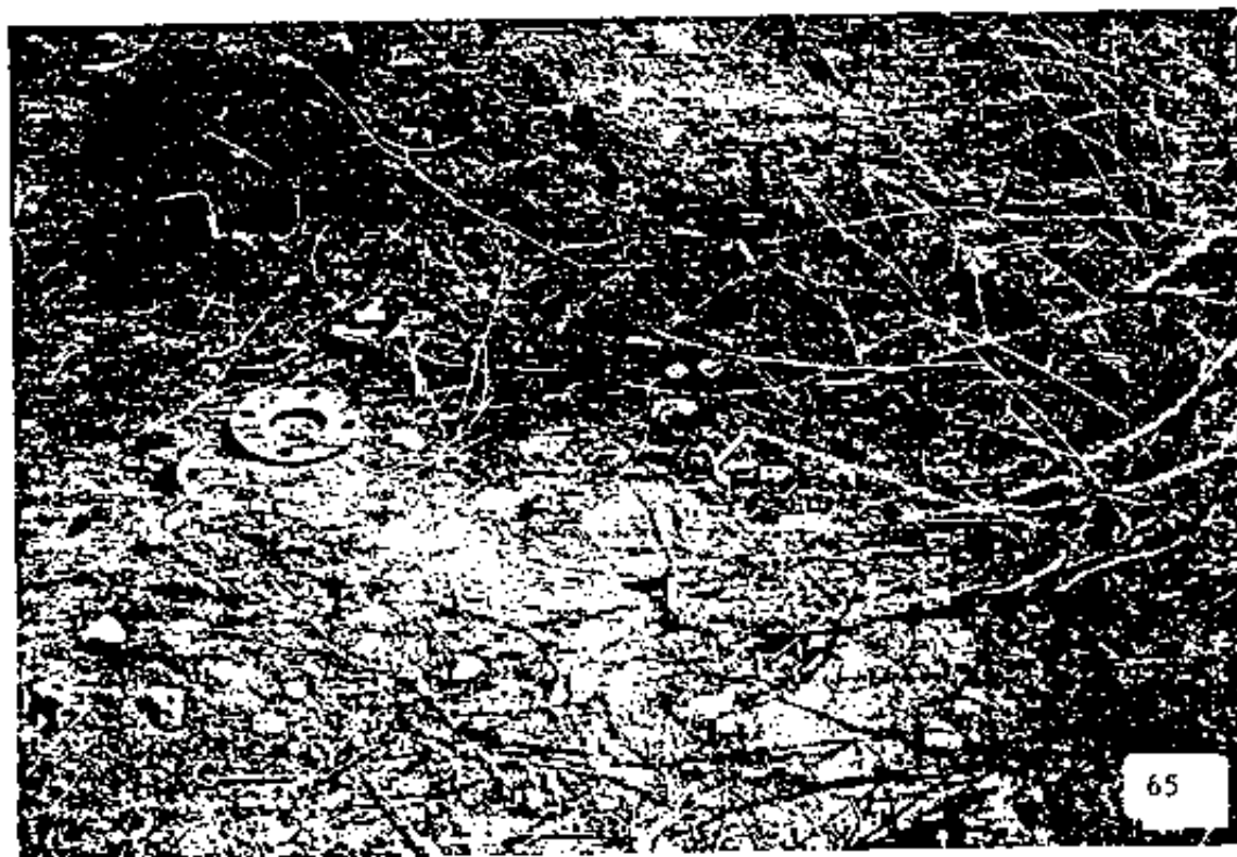
65. Stained soil, dead vegetation, and a potential asbestos gasket at the New Conservation Yard. (SWMU 7.8)
