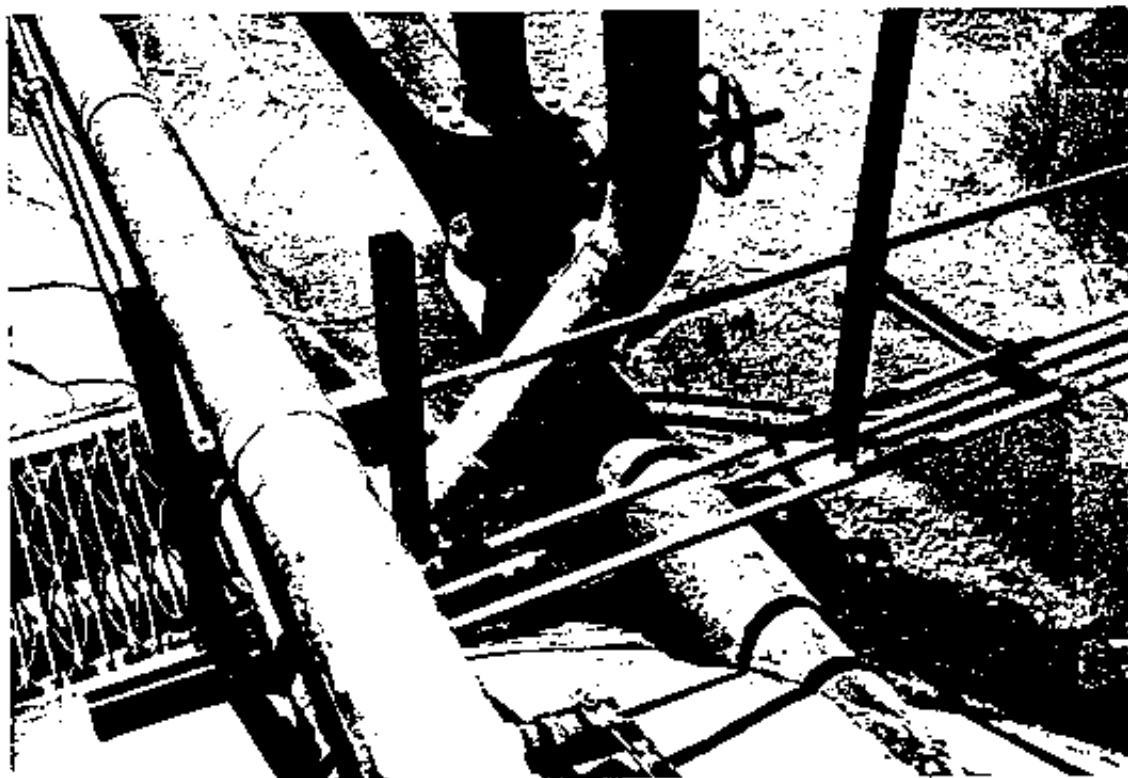
1-L. Advanced Propulsion Test Facility - Fuel lines within cement-lined trenches. (SWMU 4.9)
