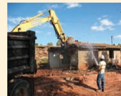
Demolition of contaminated home
