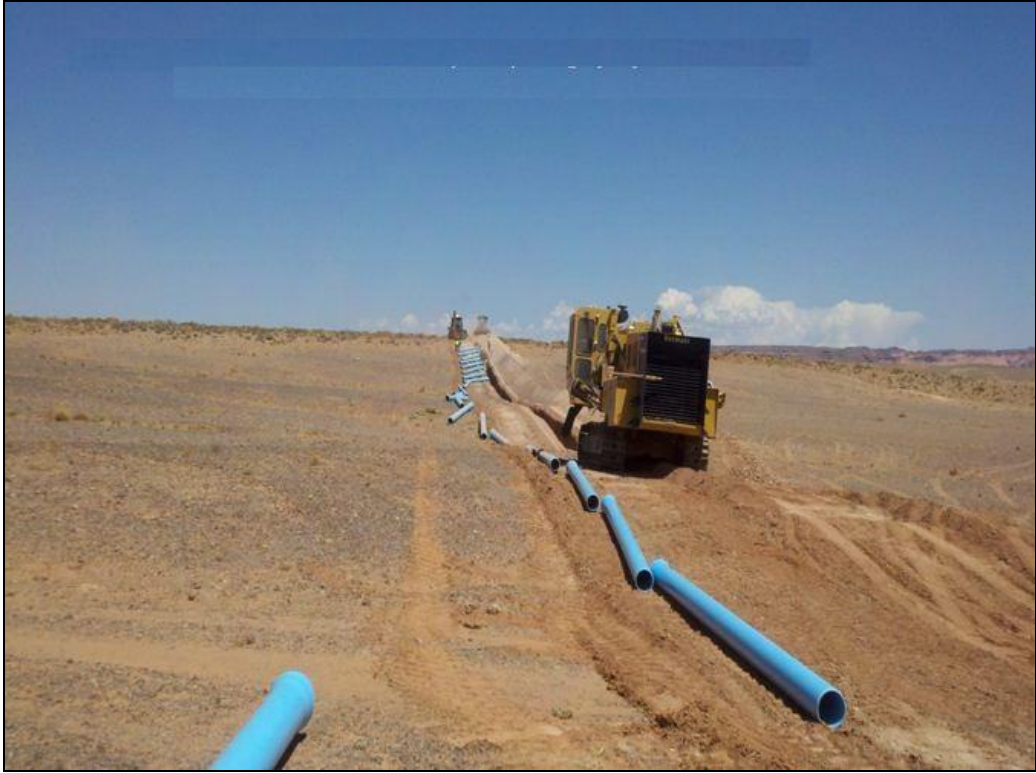
New Infrastructure Construction
