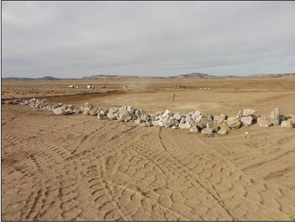
Cleanup at Section 32/33
