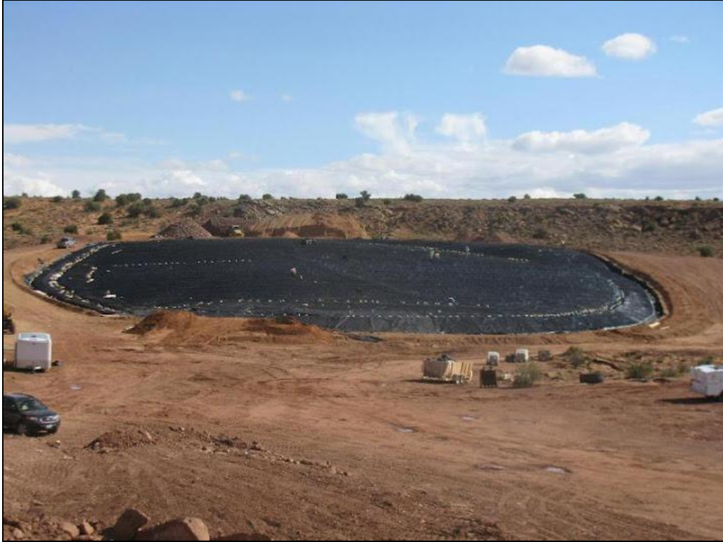
Repository Cell at Skyline Mine
