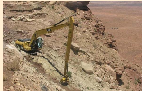
Large scale cleanup at Skyline Mine
