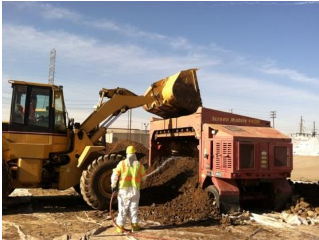
Figure 3: Loading shaker, note worker spraying soils as they fall from screen, note lack of dust.
