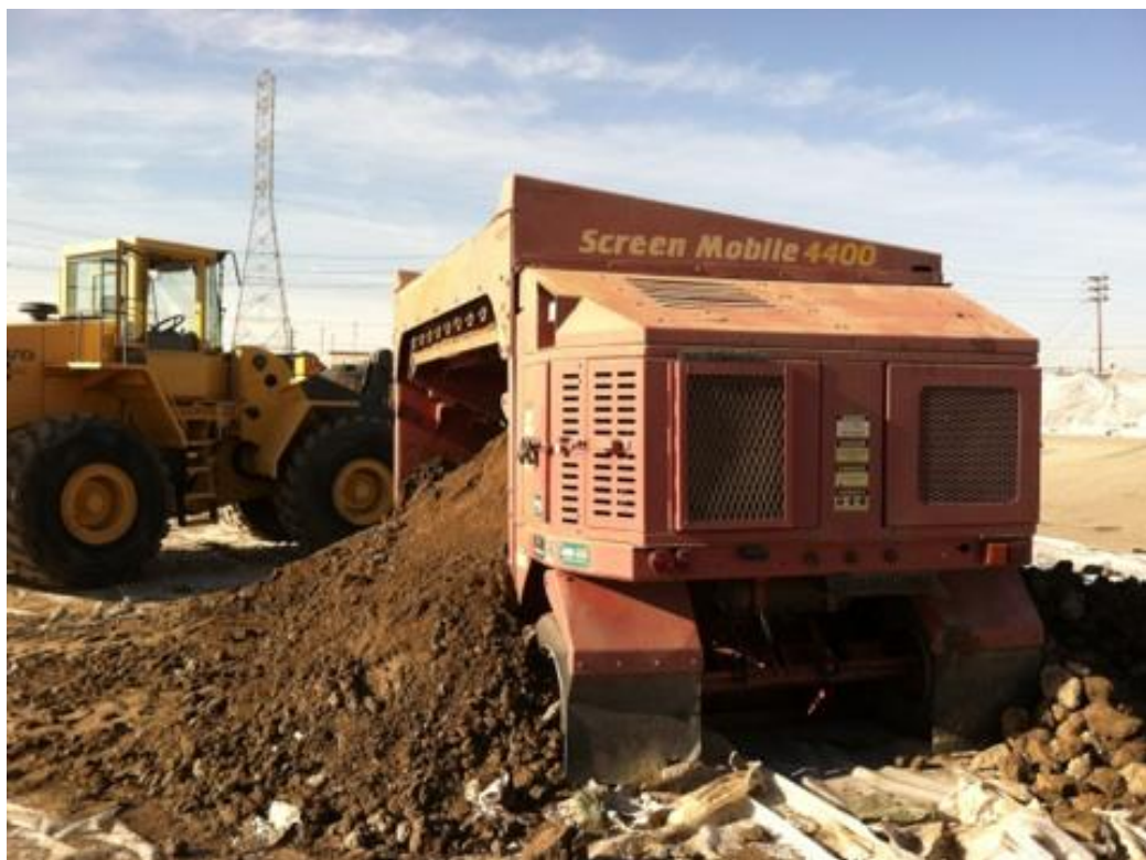
Figure 2: Soil screening machine.
