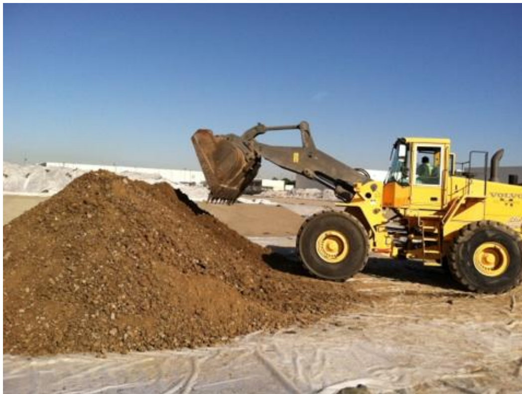
Figure 4: Screened soil being dumped on stockpile, note lack of dust.
