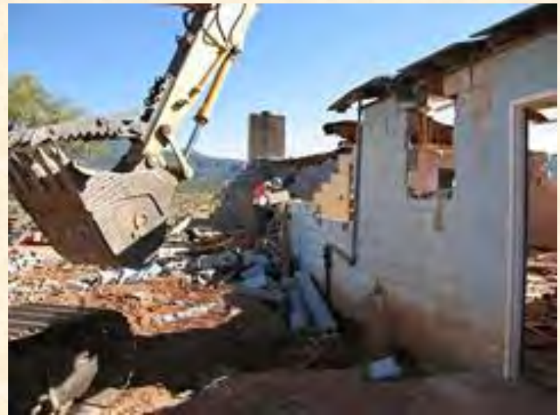
Contaminated Structure Removal
