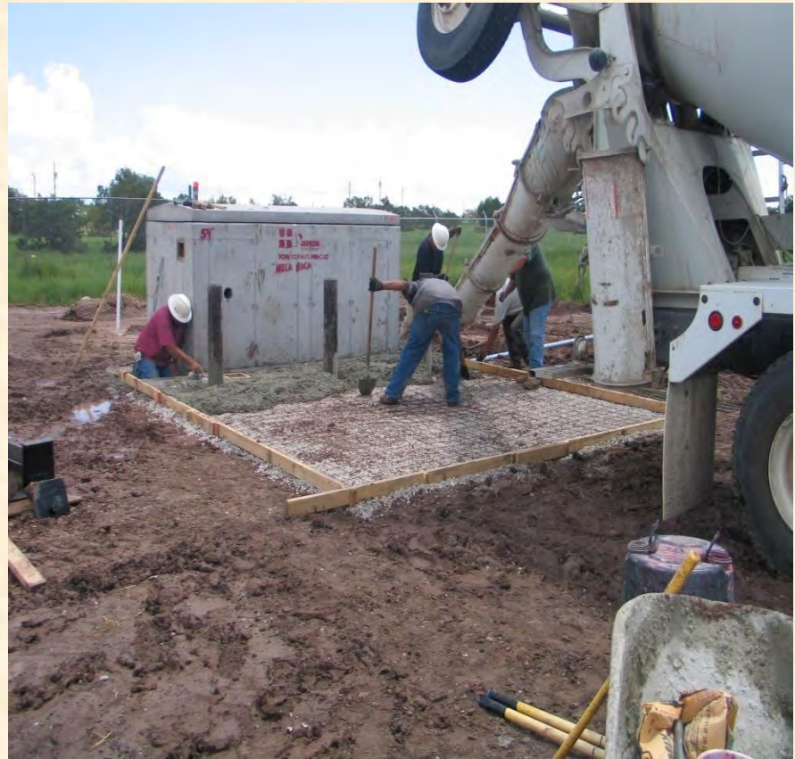
Baca Watering Point Construction
