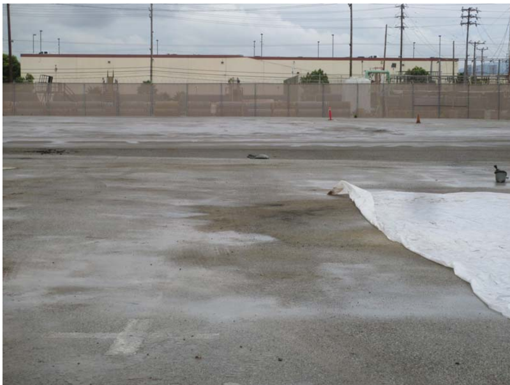
Figure 3: Pavement areas sprayed with water to control dust. No dust observed.
