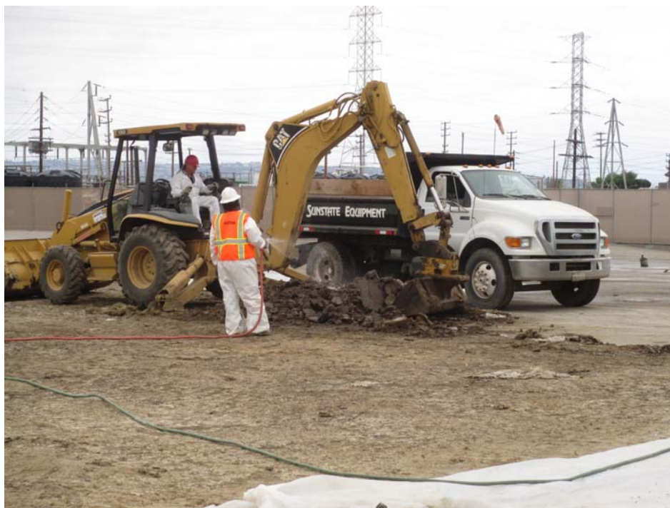
Figure 2: Worker spraying water for dust control on soil material being removed from stockpile and loaded into dump truck for use as fill. No dust observed.
