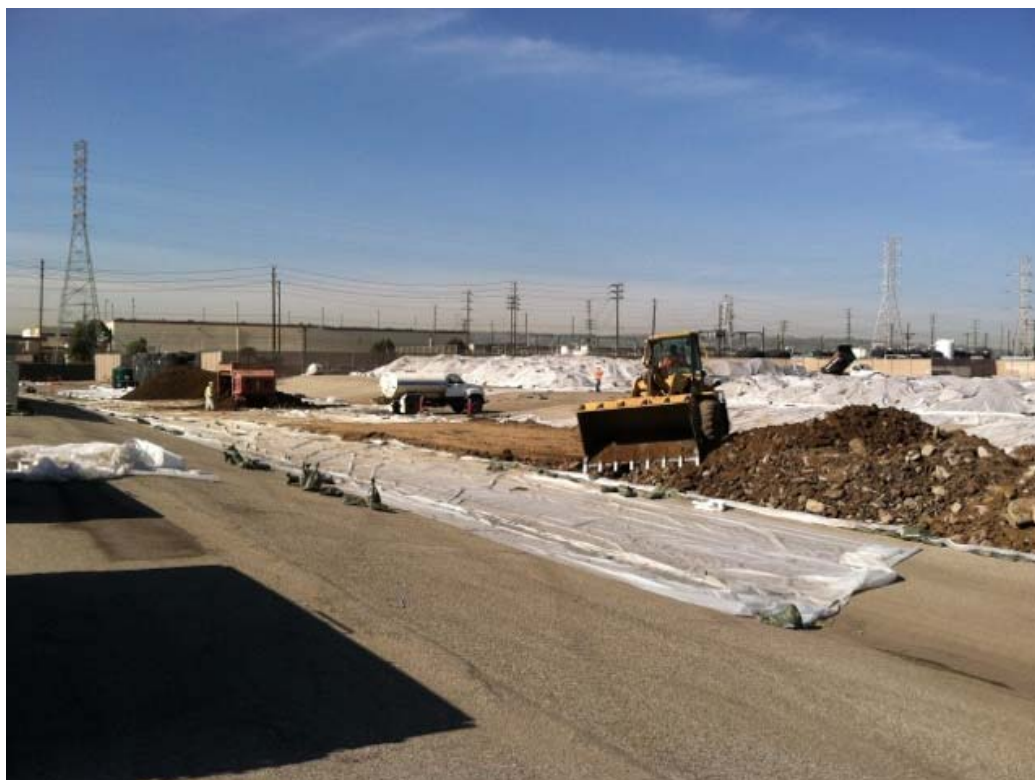
Figure 1: Soil screening - stockpile from excavation north of shaker, shaker (red machine), and stockpile of screened soil south of shaker (distance).
