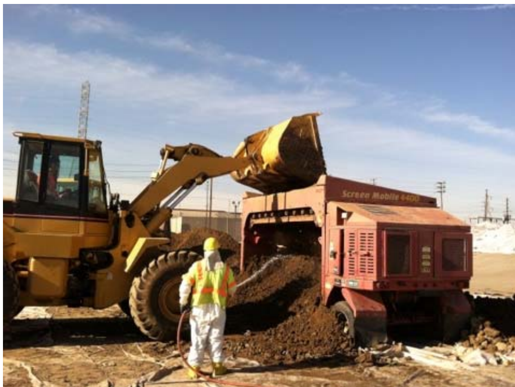
Figure 3: Loading shaker, note worker spraying soils as they fall from screen, note lack of dust.
